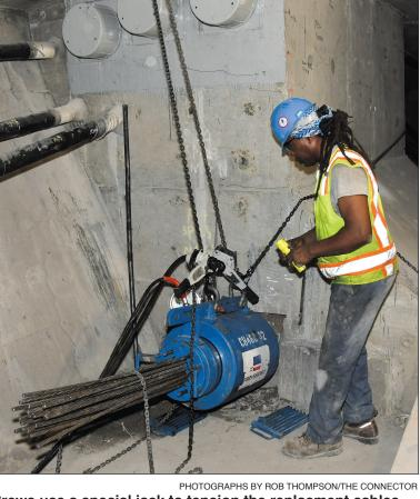
Crews use a special jack to tension the replacment cables on the structure. Two extra cables are being installed on both west and east bound bridges for safety and redundancy.
