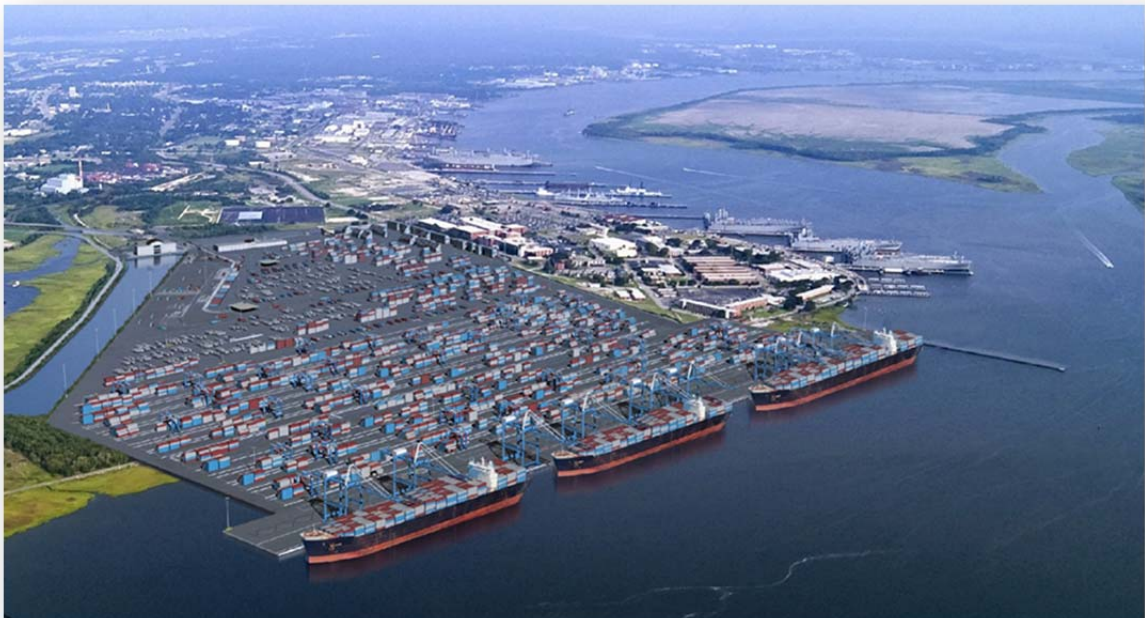
Figure ES-3: Rendering of the Built-Out New Container Terminal at Port of Charleston
