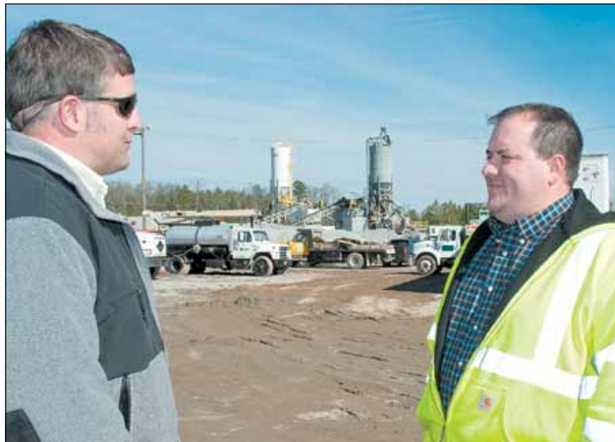
PHOTOGRAPHS BY ROB THOMPSON/THE CONNECTOR Laurens Resident Maintenance Engineer Nick Waites, left, talks with McCarthy Improvement Company Project Manager Nick Wolf at the two concrete plants for the I-385 rehabilitation project.
