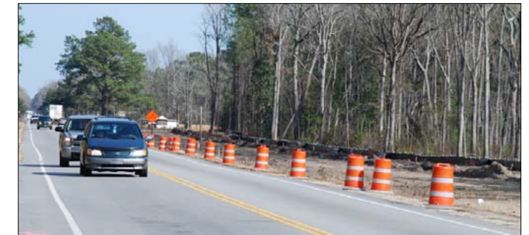
Silt fences are used along the widening project to protect the wetlands and natural habitat of wildlife throughout the ACE Basin area.
