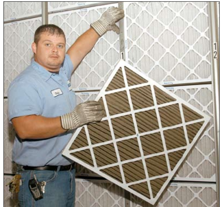
Chris Huepenbecker shows the difference between a dirty and clean air filter. The building maintenance staff is changing filters in the heating and air system to ensure clean, fresh air circulates in the building.
