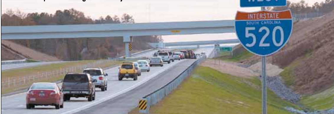
The Palmetto Parkway - Phase II project is an example of a Design Build Project.
