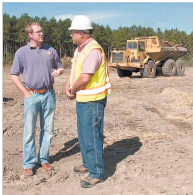
SCDOT Project Manager Daniel Burton, left, and Lane Construction Corporation Project Manager Bill Hameza watch PET graduates Steve McMillan and Ephas Brown work at the borrow pit for the US 17 project in Walterboro.
