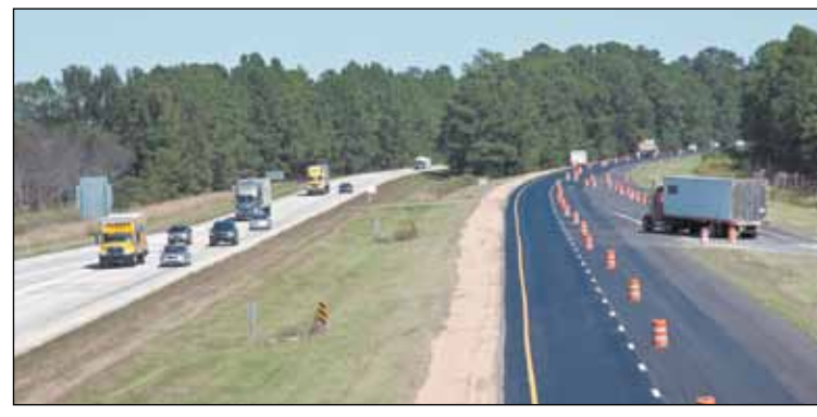
Here, the northbound lanes have been resurfaced with asphalt providing a new, smooth surface. The southbound lanes will be paved next.
