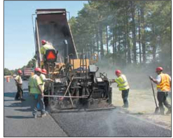
Here, the northbound lanes have been resurfaced with asphalt providing a new, smooth surface. The southbound lanes will be paved next.
