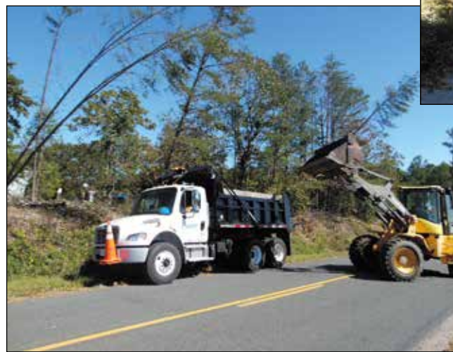
Road clearing in Calhoun county
