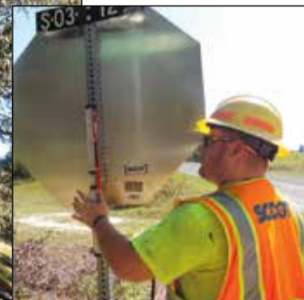
Sign replacement in Allendale
