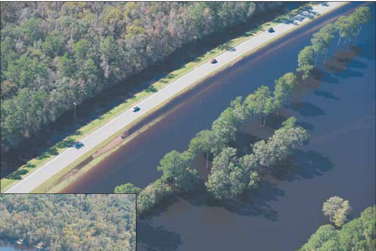
Flooding on S.C. 9, northwest of Loris, in Horry County on Oct. 13, 2016.
