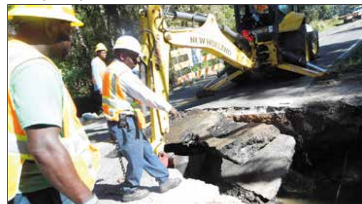
Repairs on Brown Road (S-14-365) in Clarendon County
