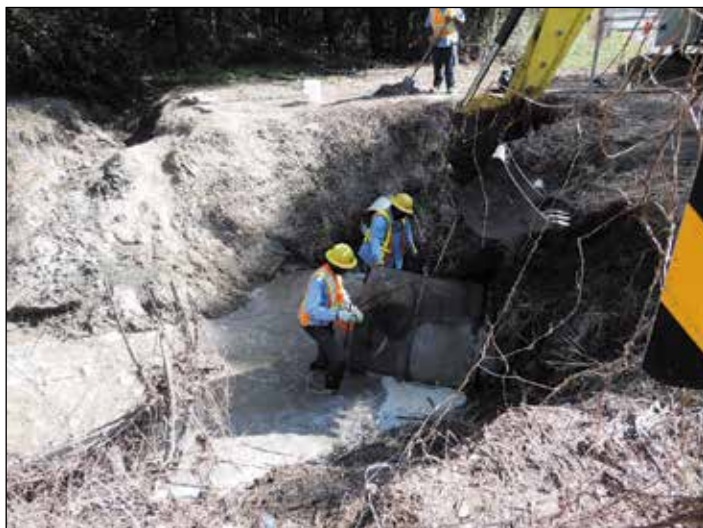
Pipe replacement near Holly Hill on S.C. 210
