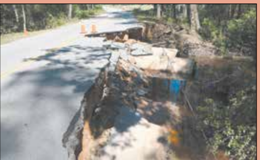
After the Hurricane Matthew floods recede, road washouts are exposed and SCDOT crews get to work making repairs.
