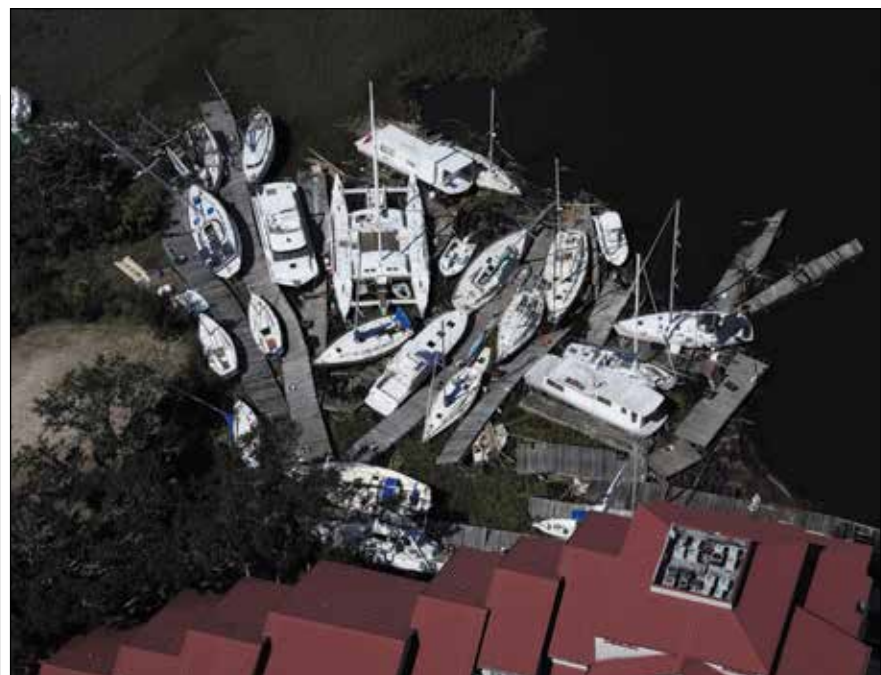
A marina full of boats was damaged when piers broke away from its supports.
