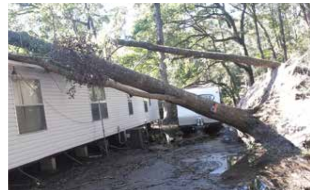
Kenny Smith of Jasper Maintenance had damage to his home from the storm.
