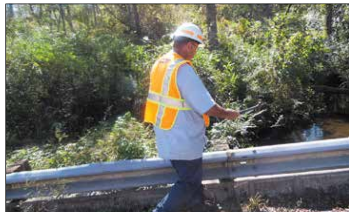
Bridge inspection on S-336 in Allendale
