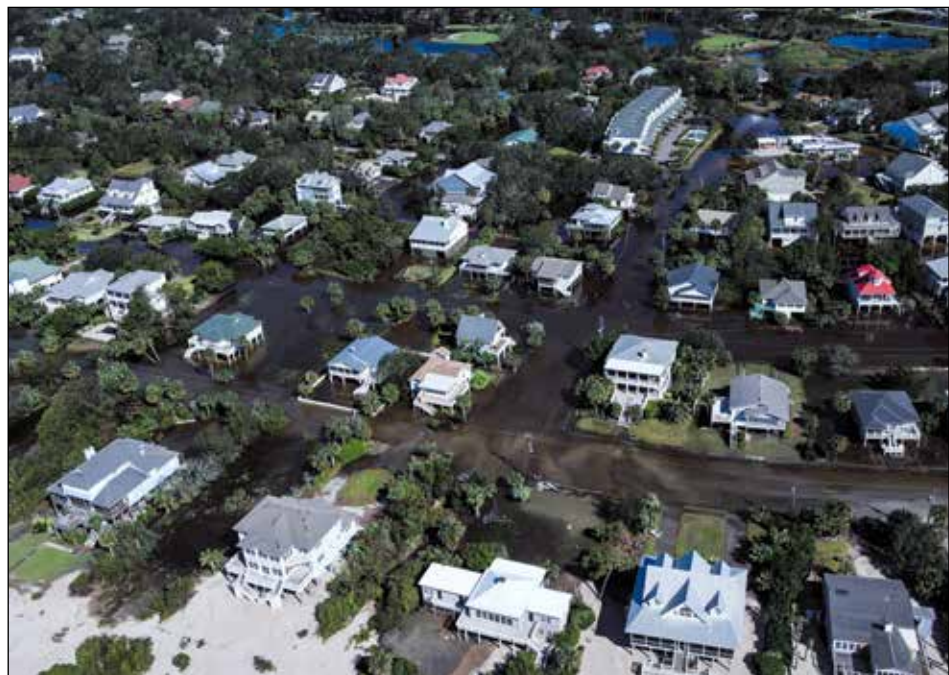
The view of Edisto Island on Oct. 9, 2016, after Hurricane Matthew shows flooded highways and damage to roofs and trees.
