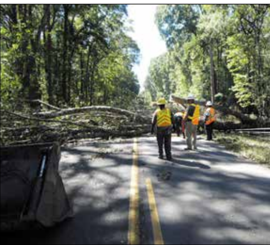
Crews remove a tree on Highway 36 in Hampton County.
