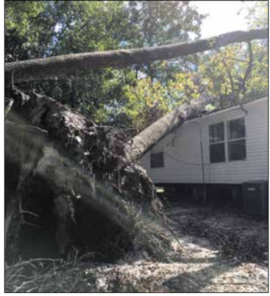
After Hurricane Matthew, more than 65 SCDOT employees' homes were damaged or destroyed by wind and flooding.
