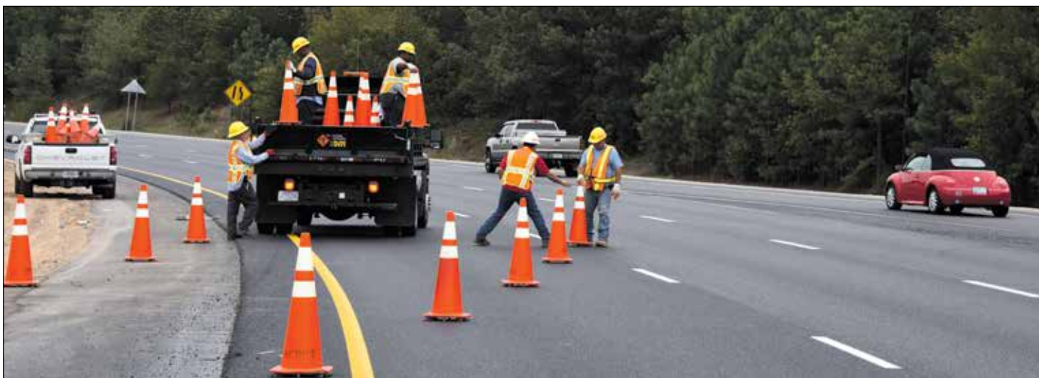
Lexington Maintenance crews put out the cones right as the last cars are stopped from traveling down I-26 East.
