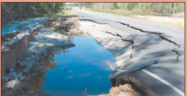
After the Hurricane Matthew floods recede, road washouts are exposed and SCDOT crews get to work making repairs.
