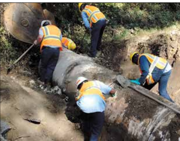
SCDOT employees repair a pipe on Gausetown Road in Kingstree.
