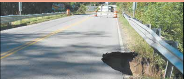
After the Hurricane Matthew floods recede, road washouts are exposed and SCDOT crews get to work making repairs.
