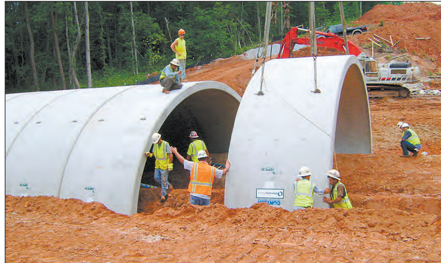
PHOTOGRAPHS BY RYAN MILLER/OCONEE CONSTRUCTION
