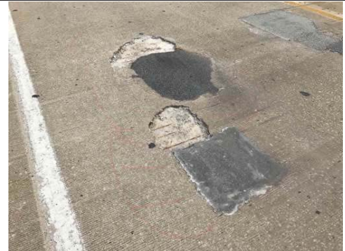
Photo #: 2 Caption: Span 9 deck ramp lane next to white line at approximately 25ft from bent 9, spall/delamination (5.5ft x 12ft x 2in) with exposed rebar
