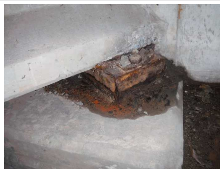
Photo #: 6 Caption: Clean and paint bearings [10 bearings]
