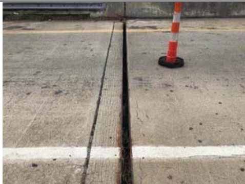
Photo #: 3 Caption: End bent 1 joint, joint material missing (full length)
