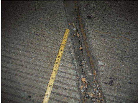
Photo #: 1 Caption: Expansion joint damage
