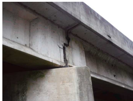
Photo #: 2 Caption: Patch Spalls in Beams [approx 14LF]
