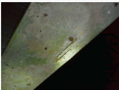
Photo #: 5 Caption: clean and paint exposed prestressing strands in beams [approx 16LF]
