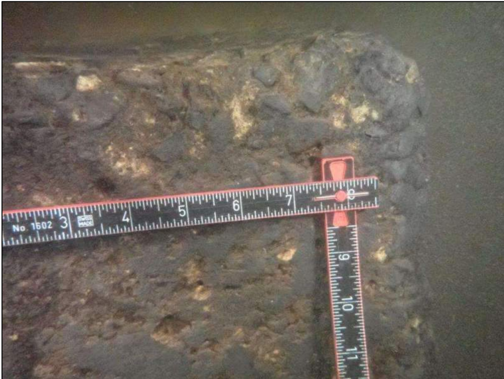
Photo 10: Bent 8, Footing 2, Typical Concrete Condition Below Waterline
