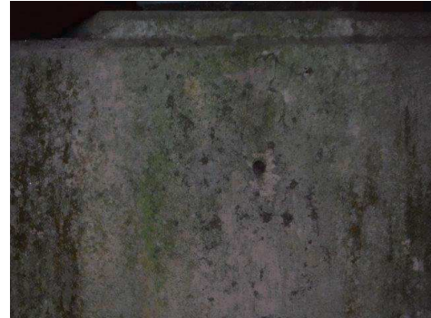
Photo #: 2 Caption: Spalls in concrete cap
