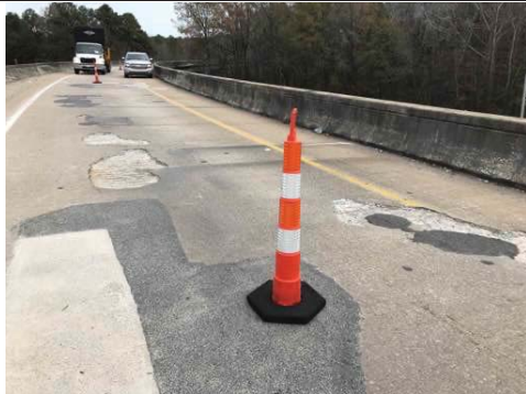
Photo #: 1 Caption: Span 12 middle of ramp lane near midspan, (3) spalls (up to 4ft x 9ft x 2in) with exposed rebar
