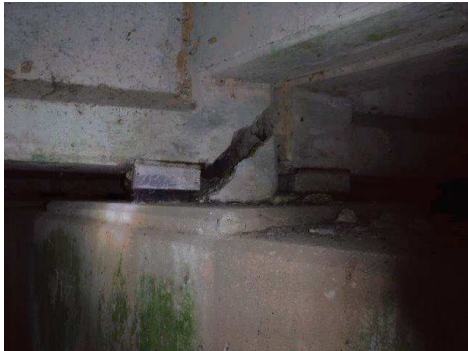
Photo #: 3 Caption: Spalls in concrete beams
