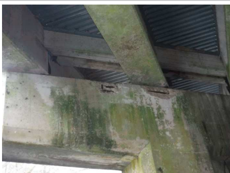
Photo #: 3 Caption: Clean and paint all exposed rebar in caps, columns and deck. [approx 41LF]
