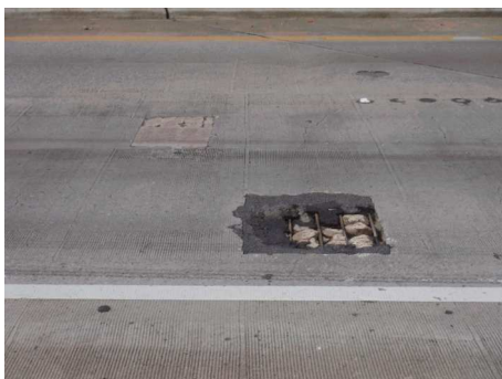
Photo #: 7 Caption: Patch spalls in top of deck [approx 75SF]
