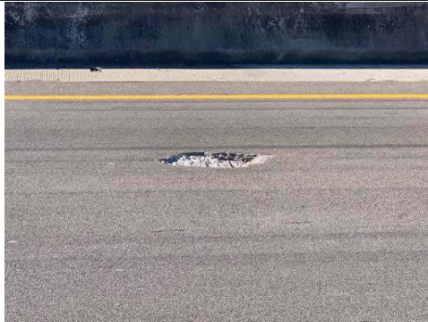
Photo #: 1 Caption: Span 4 deck left lane near midspan, spall (2ft diameter x 2in deep) with exposed rebar
