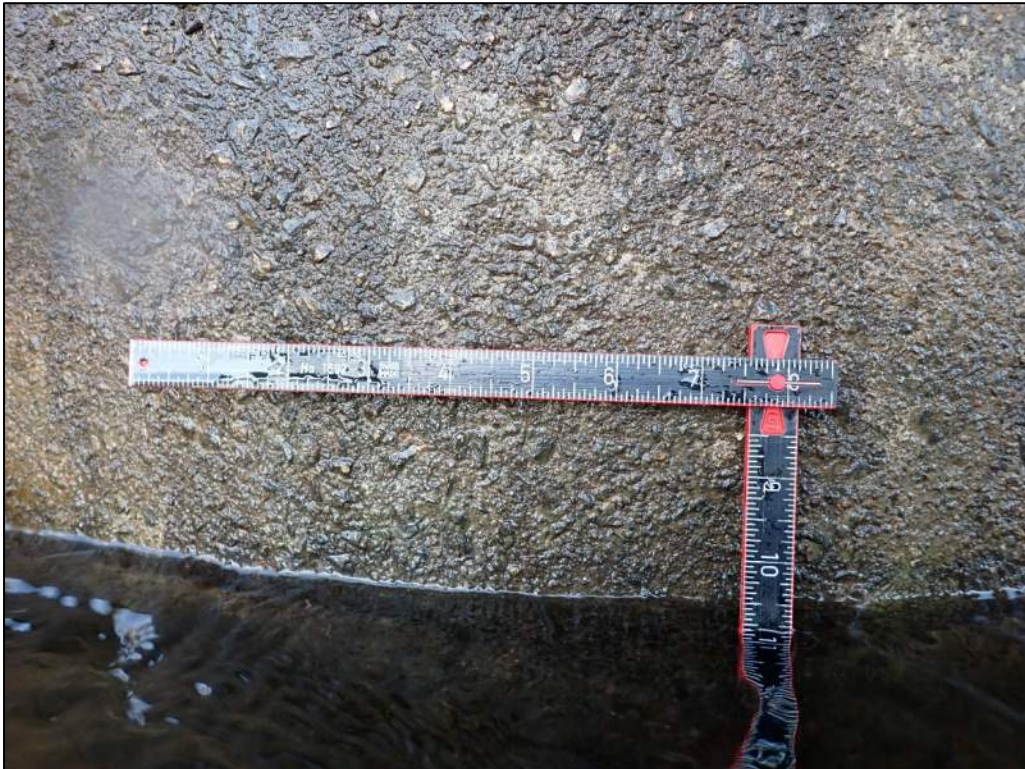
Photo 8: Bent 17, Upstream Nose, Typical Concrete Condition at Waterline
