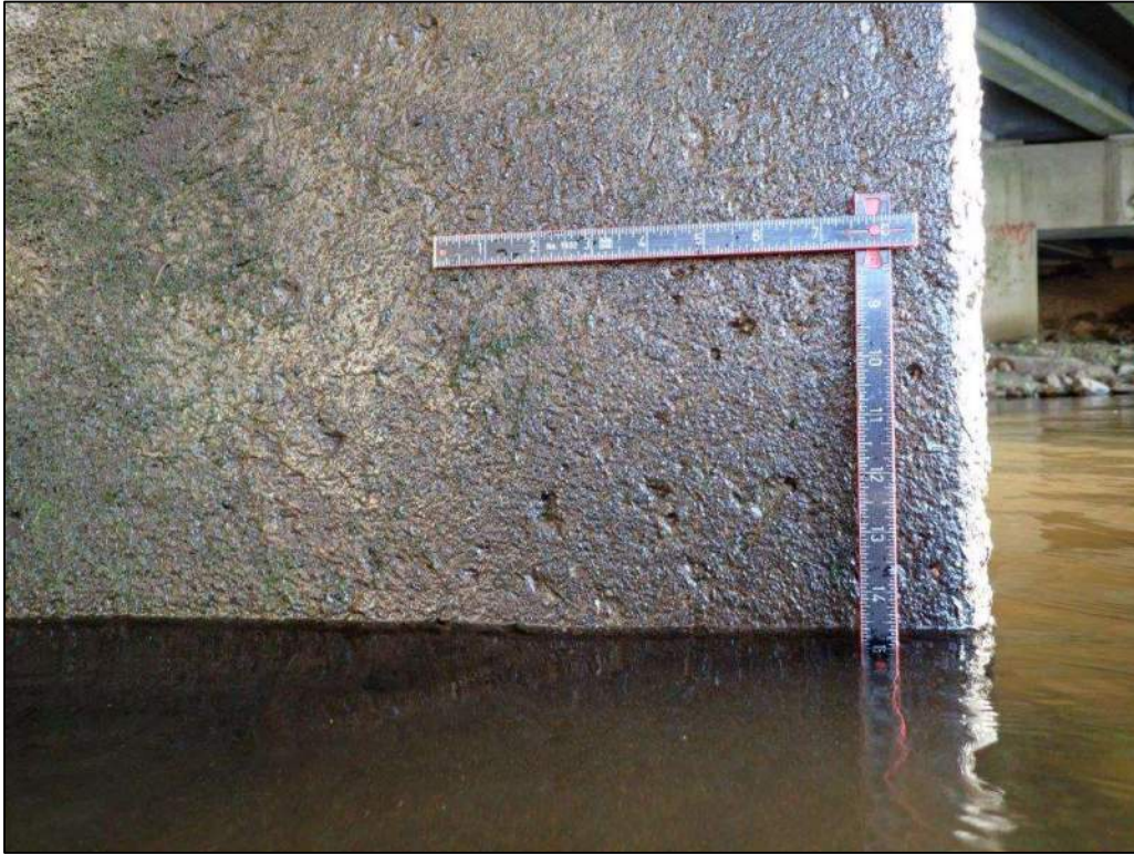
Photo 9: Bent 9, Column 5, Typical Concrete Condition at Waterline
