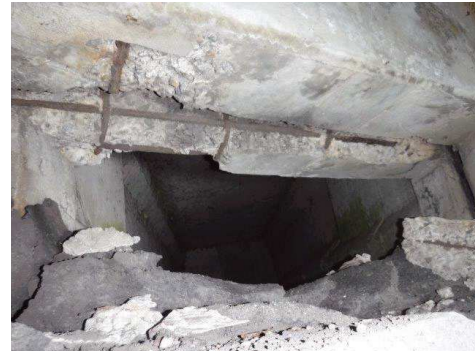
Photo #: 4 Caption: Spalls in concrete diaphragms
