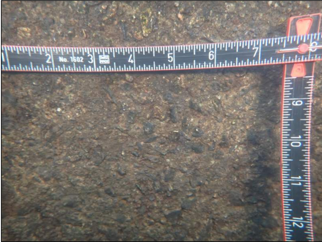
Photo 9: Bent 17, Upstream Nose, Typical Concrete Condition Below Waterline
