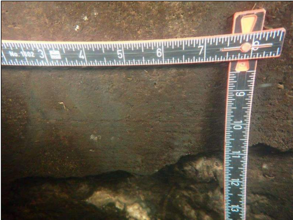
Photo 12: Bent 8, Column 4, Delamination/Spall
