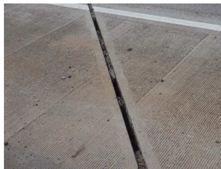
Photo #: 8 Caption: repair/replace joints due to seal adhesion/missing [approx 1100LF]
