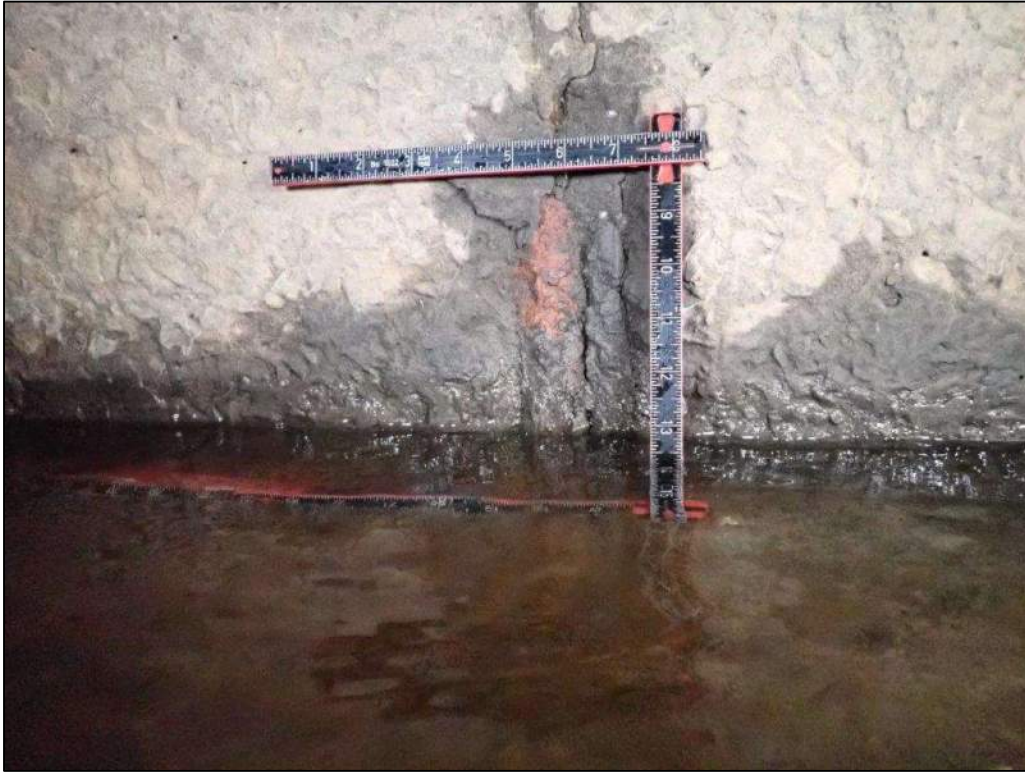
Photo 11: Bent 8, Column 2, Spall with Exposed Rebar
