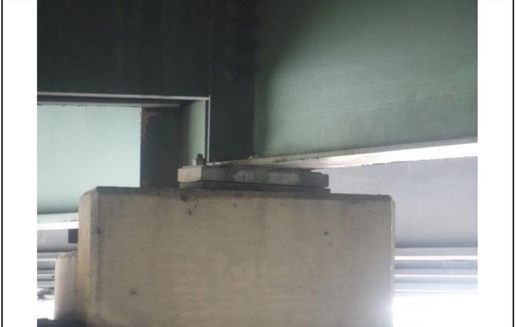
14 TYPICAL INTERIOR BENT BEARING
