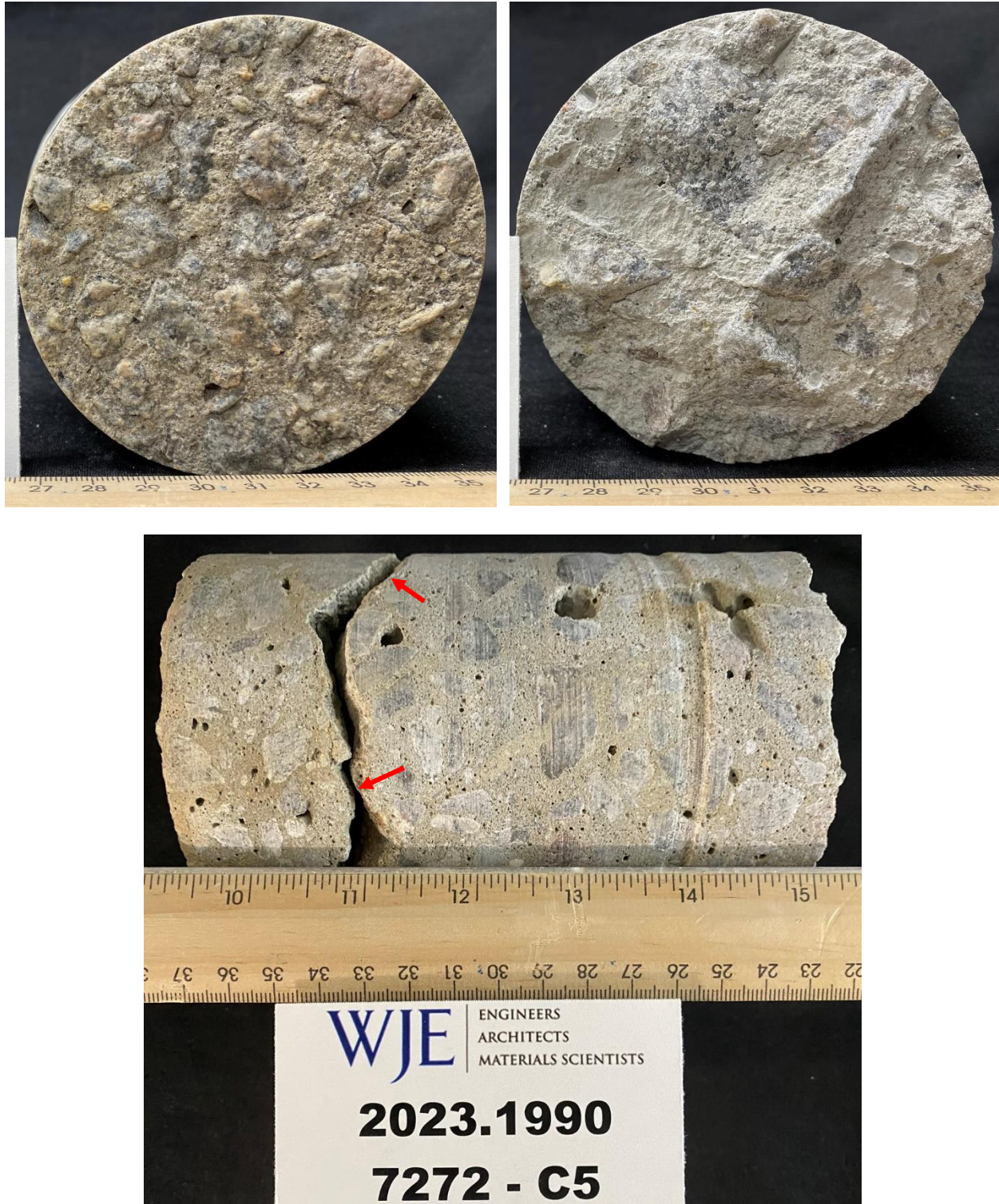
Figure 2. 7272-C5. As-received, with the top surface in the top left image, bottom surface in the top right, and a longitudinal view of the core with the top surface to the left in the bottom image. Red arrows indicate a surface-parallel to surface-oblique fracture.
