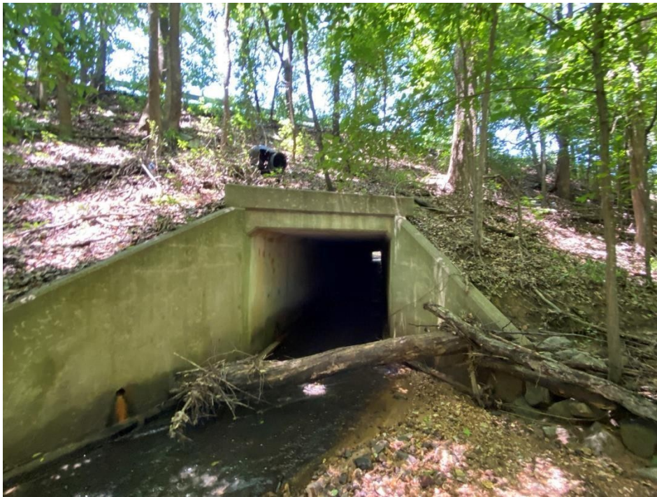
Photograph 2 – Phase 3, Unnamed Culvert (Box) 1010
