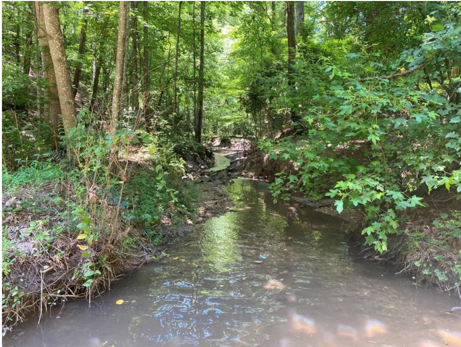
Photograph 3 – Phase 3, Culvert EC-3201 – Outflow to stream
