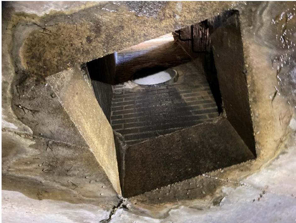
Photograph 8 – Phase 3, Culvert EP-2201 (Double Box) – Inside view to street access
