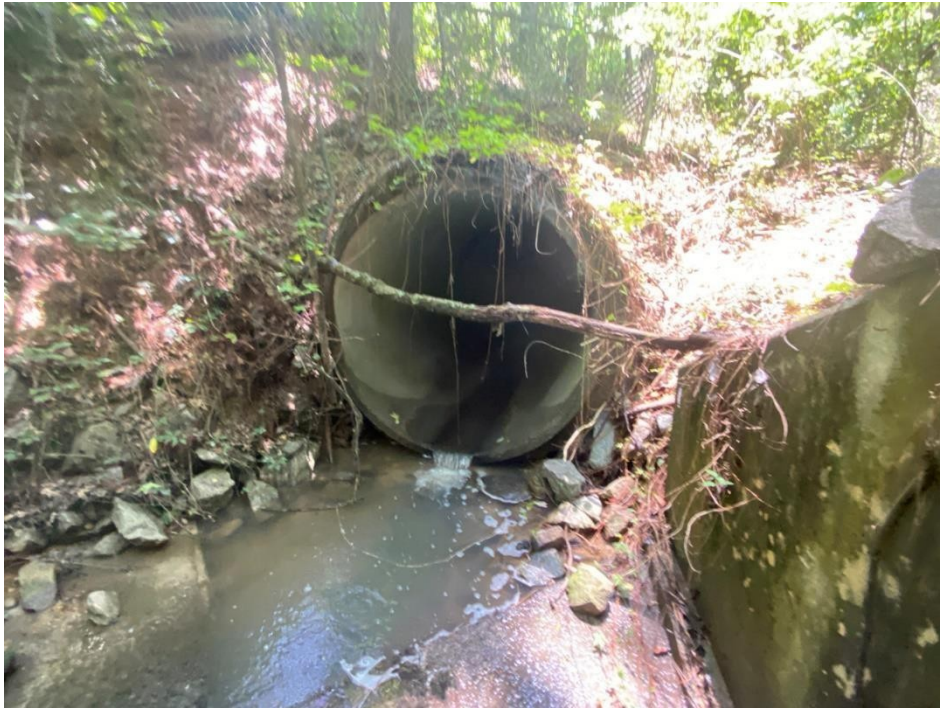
Photograph 1 – Phase 1, Unnamed Culvert (Pipe) 1001 – Outflow
