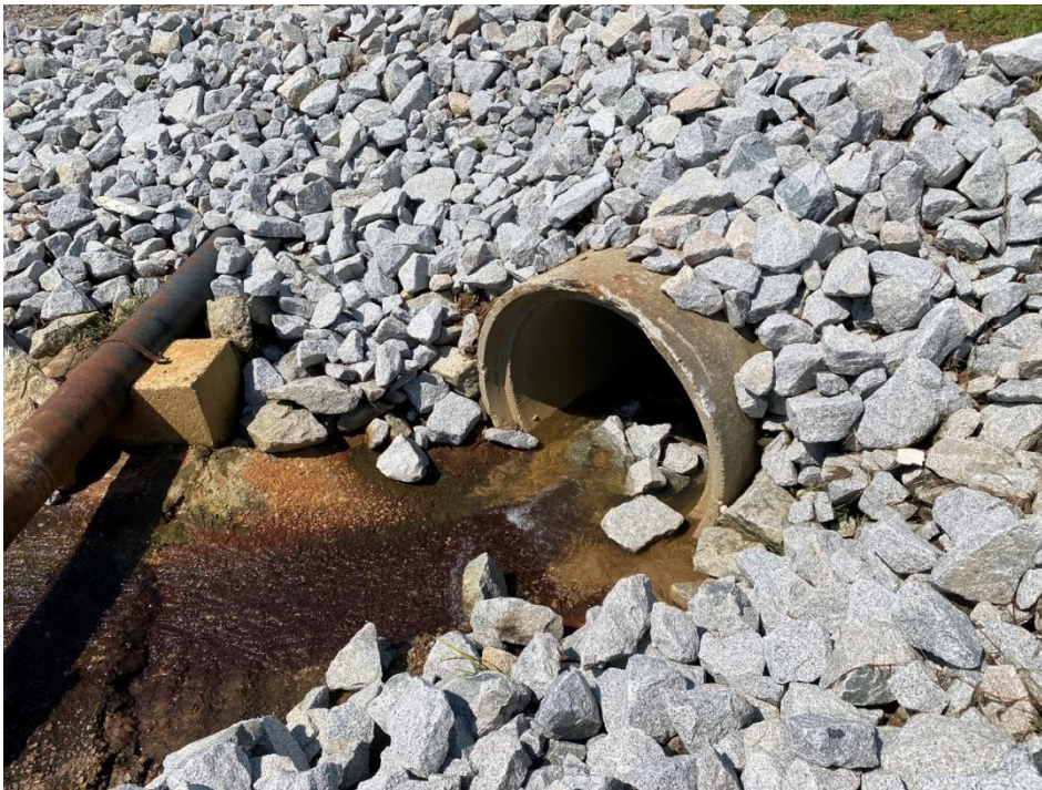
Photograph 4 – Phase 3, Culvert EP-2201 – Inaccessible
