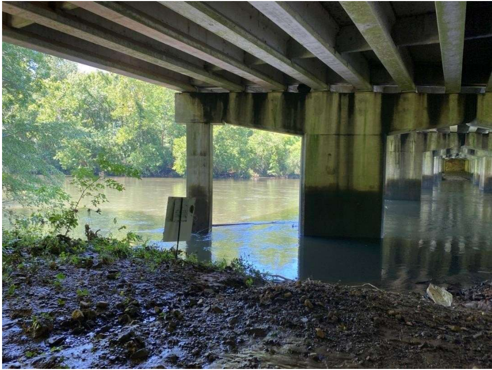
Photograph 5 – Phase 3, Bridge 4604: I-20 over Saluda River
