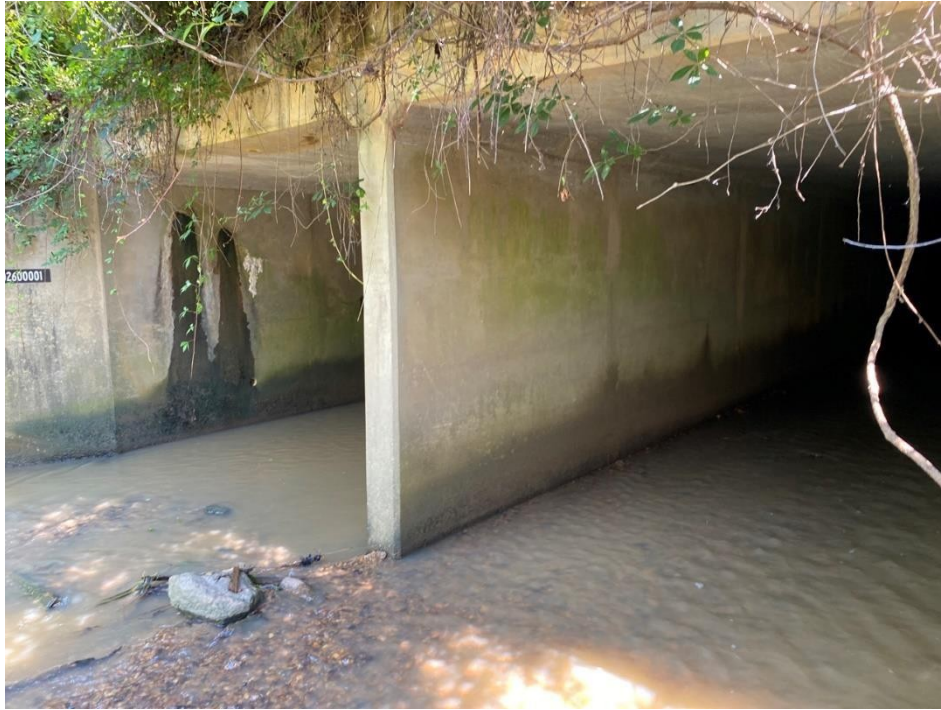
Photograph 7 – Phase 3, Culvert EP-2201 (Double Box)
