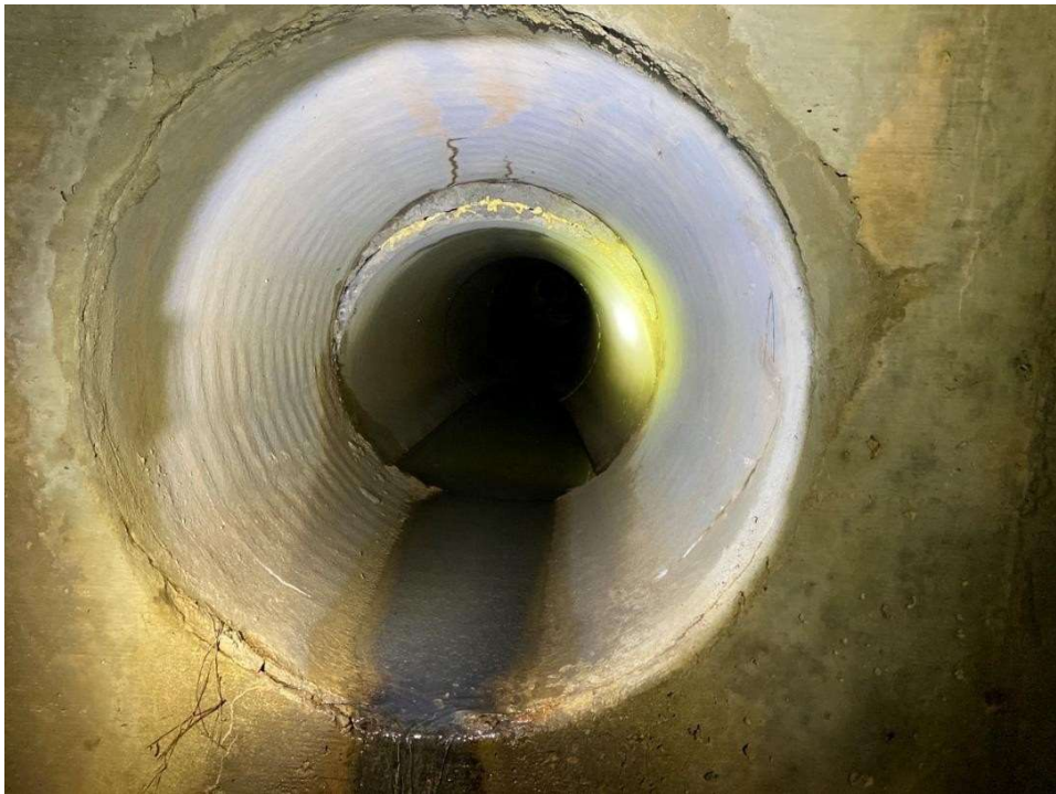
Photograph 6 – Phase 3, Culvert EP 2121 (Pipe) – Inside view
