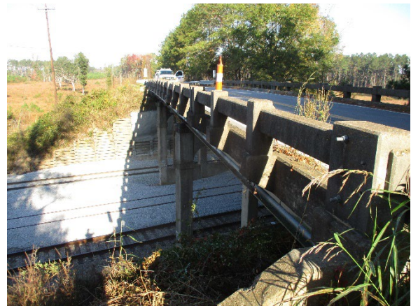
Photo 4. Southwest Side View of Bridge.
