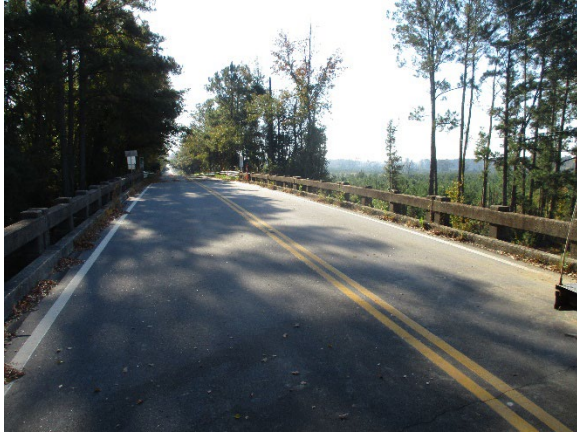
Photo 1. Top View of Bridge Deck.
