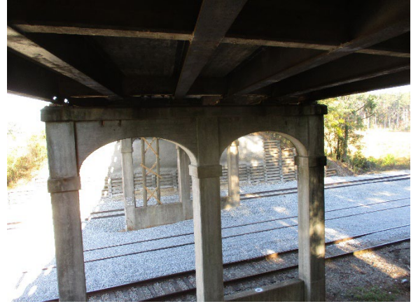
Photo 2. Underside View of Bridge.
