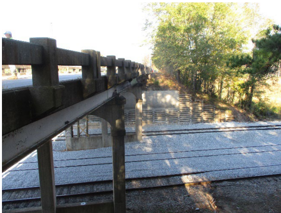
Photo 3. Southeast Side View of Bridge.
