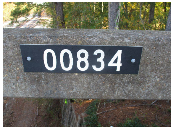
Photo 6. SCDOT Bridge Asset Placard Attached to the Concrete Guardrail.
