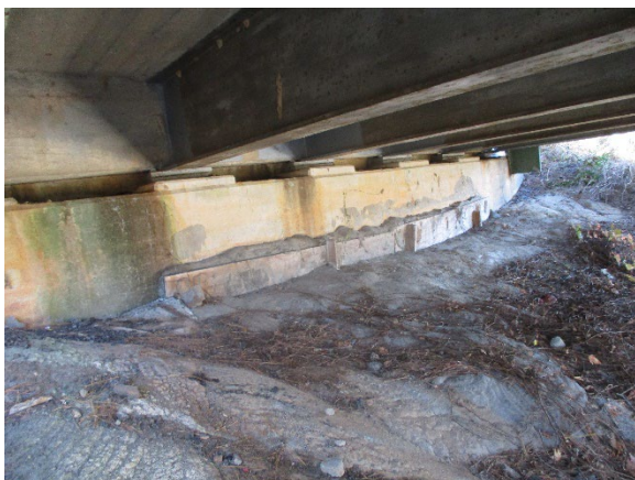
Photo 5. End Bent Underside View.
