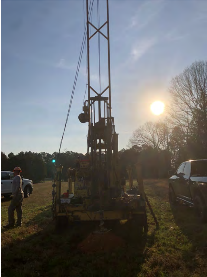
Figure No. 1: Rear View of Drill Rig
