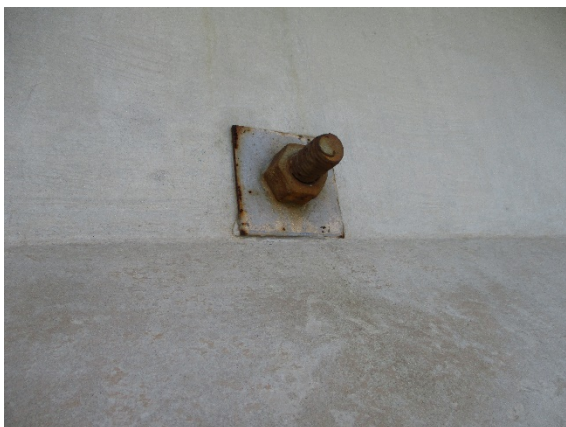
Photo 5. LBP Positive Tie Rod Bolt
