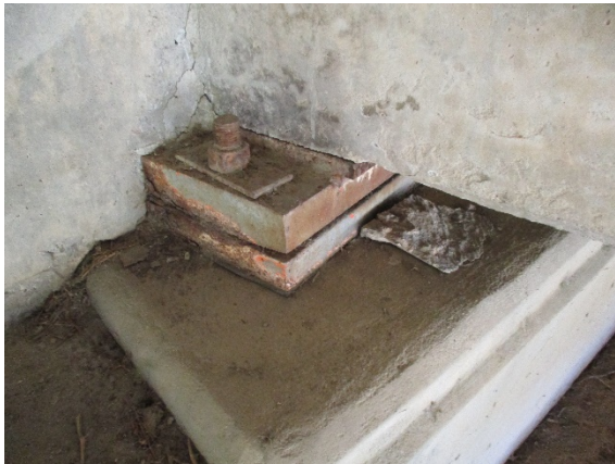
Photo 3. LBP Positive Bent Plate
