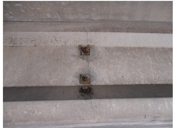
Photo 4. LBP Positive Tie Rod Washer
