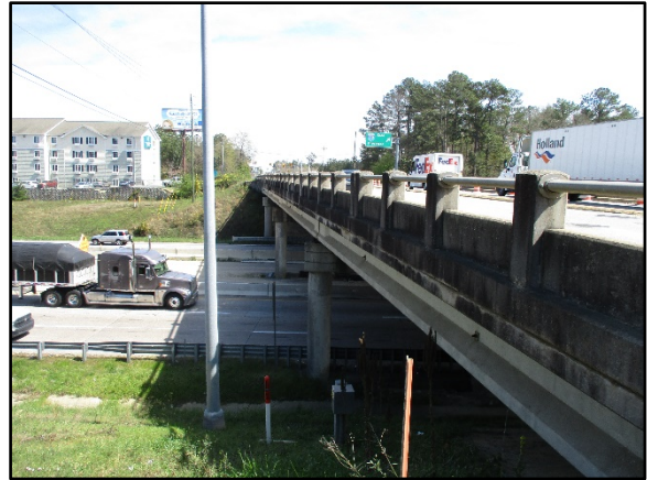
Photo 1 – US-1 Bridge over I-20 in Lexington, SC.
