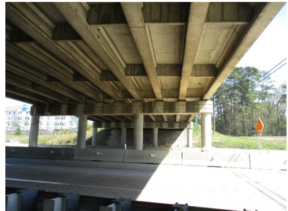
Photo 4. View of Underside of Bridge
