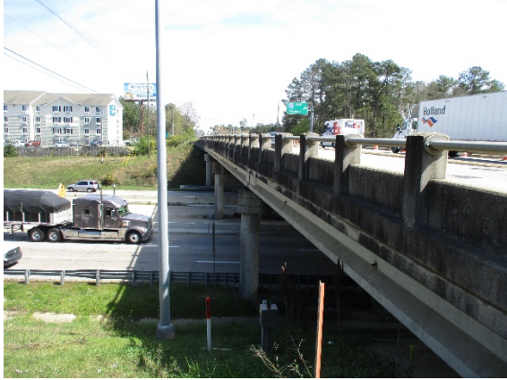
Photo 1. North Side View of Bridge
