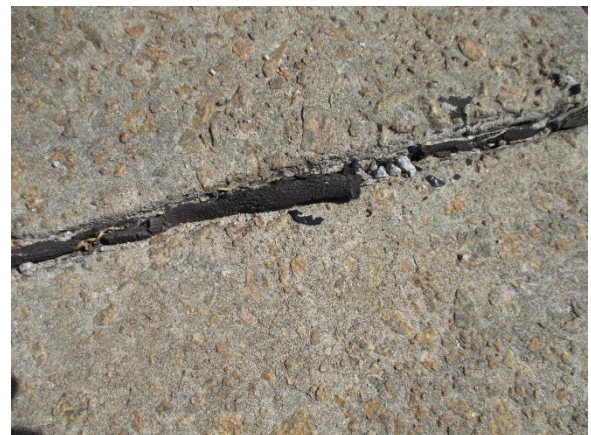
Photo 6. Non-ACM Expansion Joint Material
