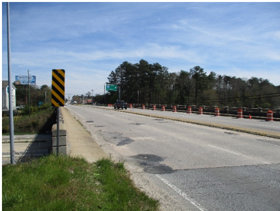
Photo 3. View of Topside of Bridge
