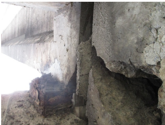
Photo 5. Non-ACM Expansion Joint Board
