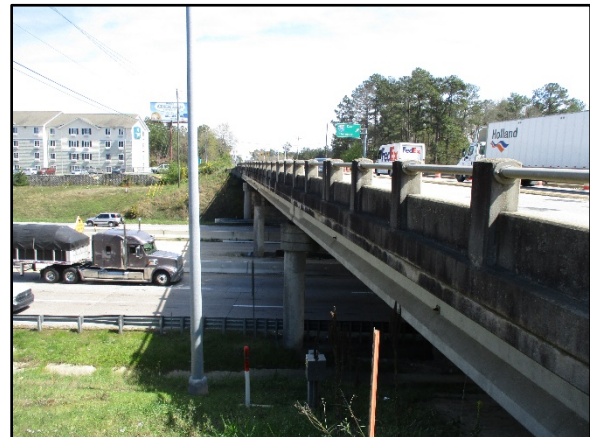
Photo 1 – US 1 Bridge over I-20 in Lexington, SC.
