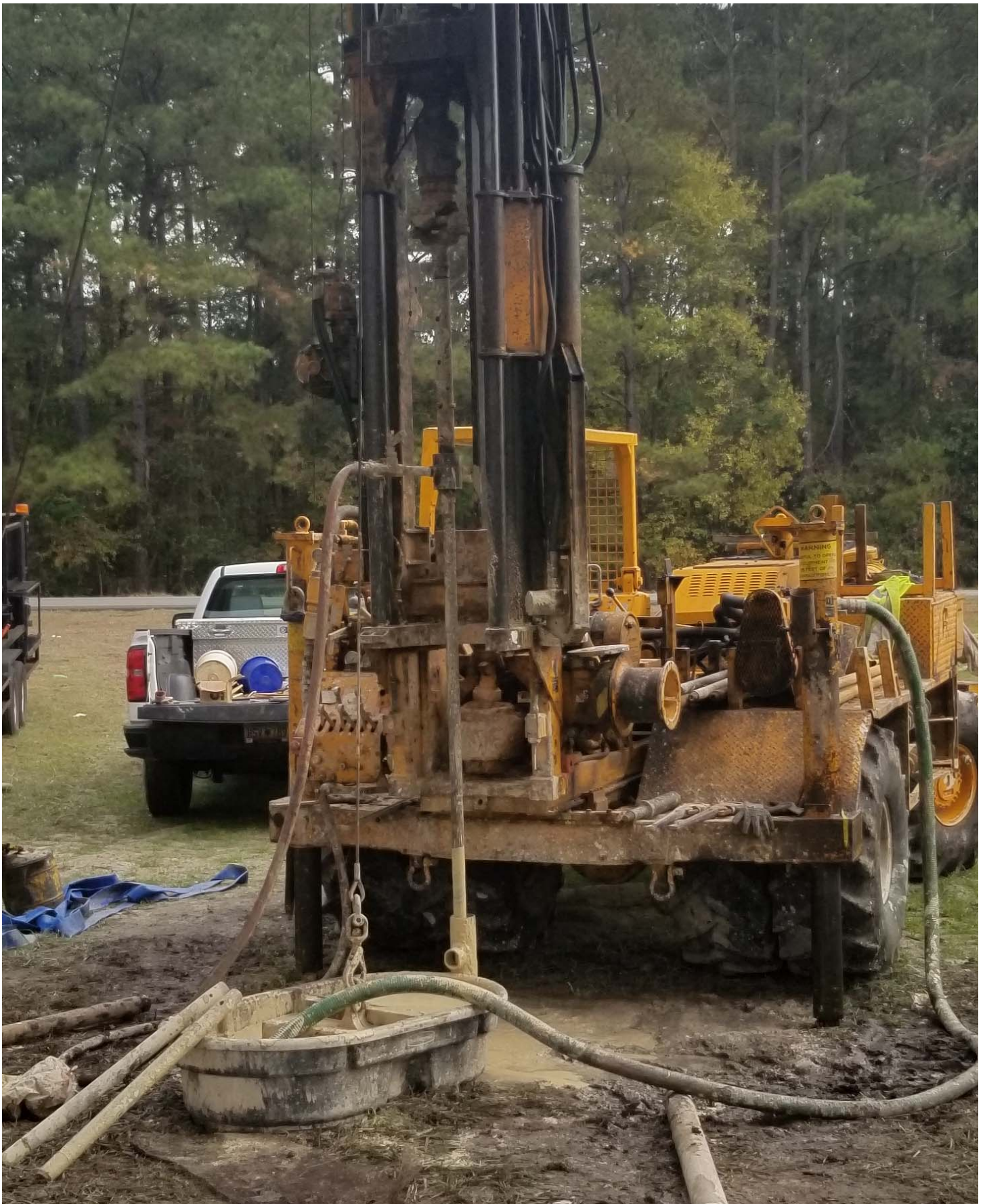
Figure No. 5: Photograph of Boring STB-03 Being Drilled
