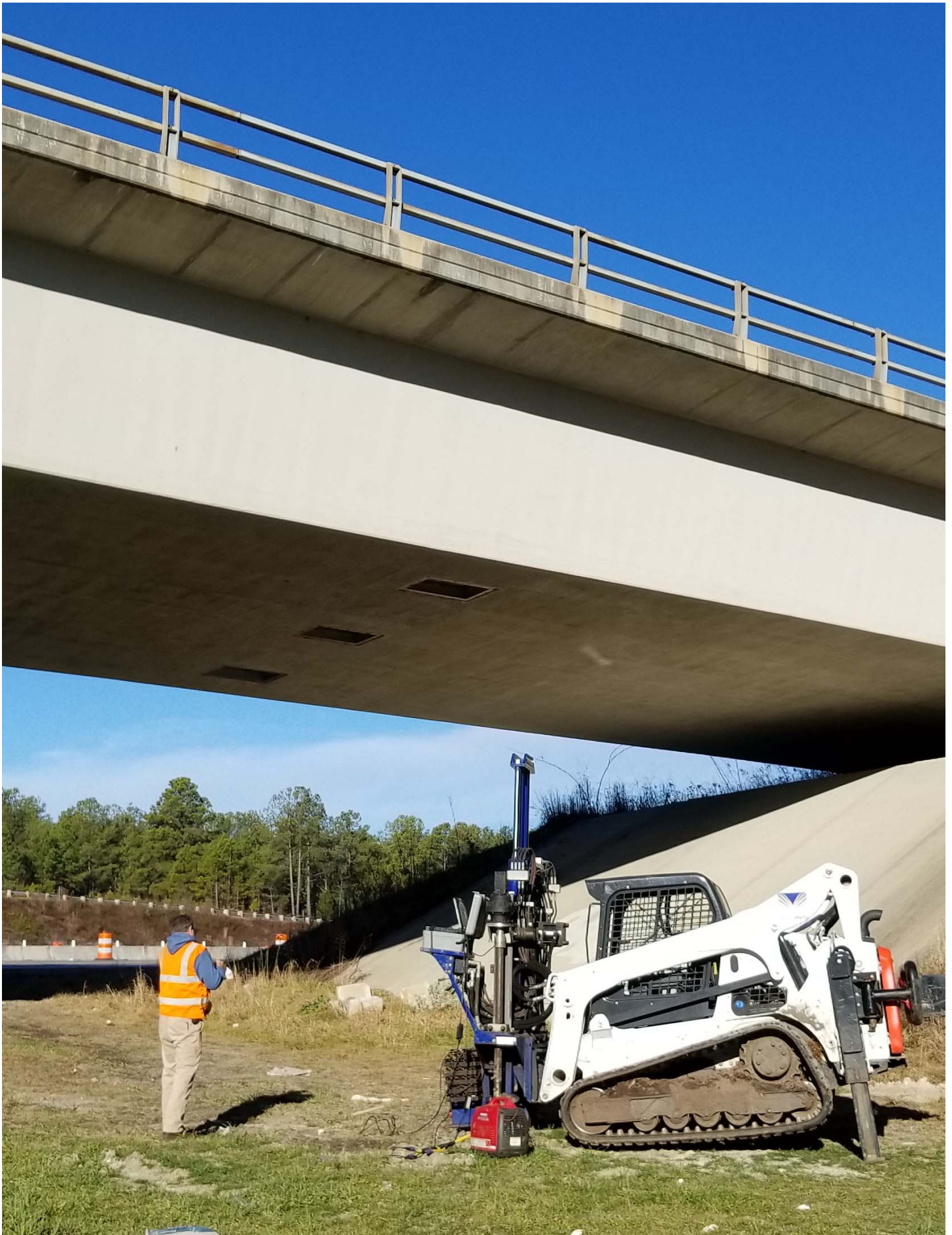
Figure No. 6: Photograph of CPT-03 Being Drilled
