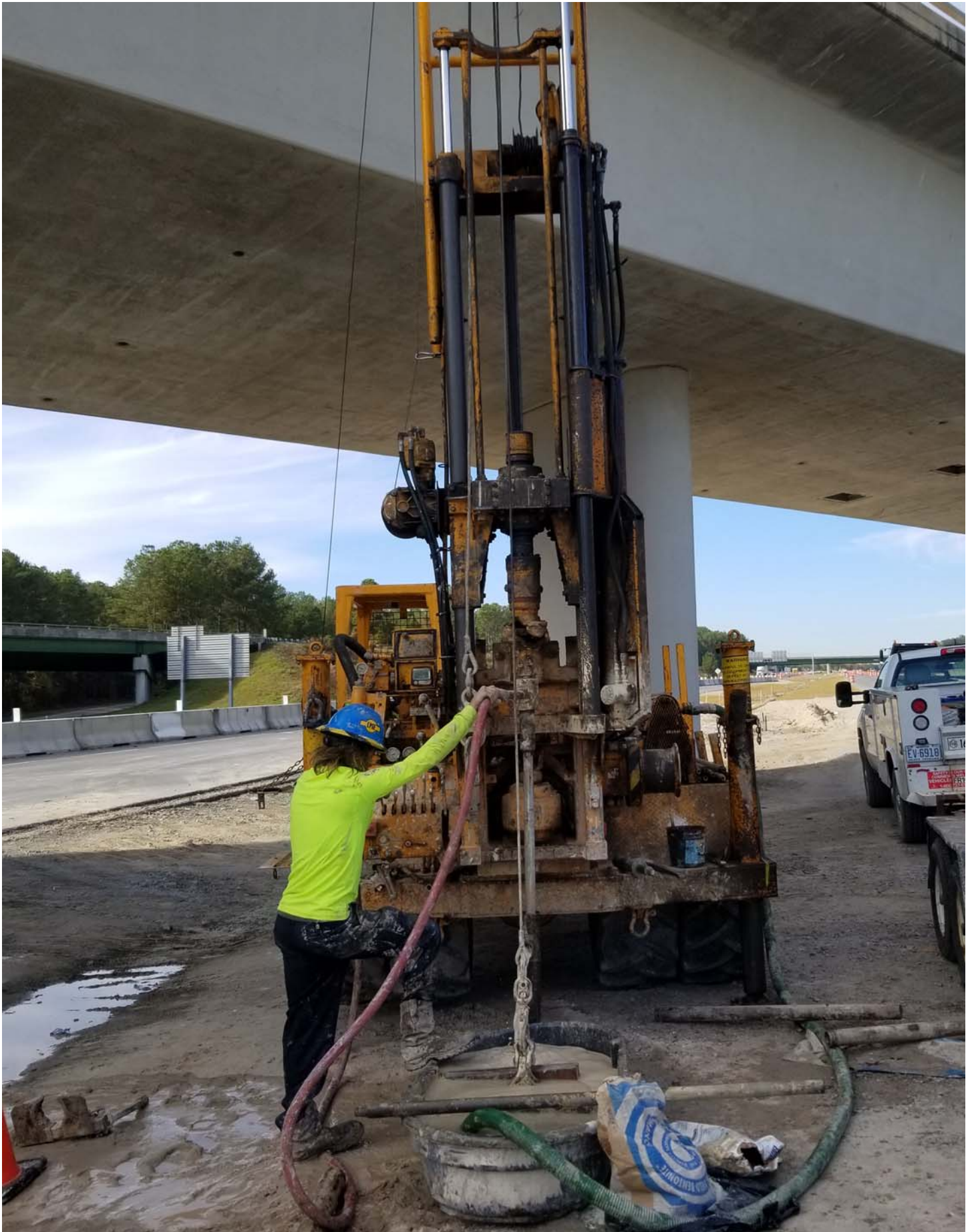
Figure No. 4: Photograph of Boring STB-02 Being Drilled
