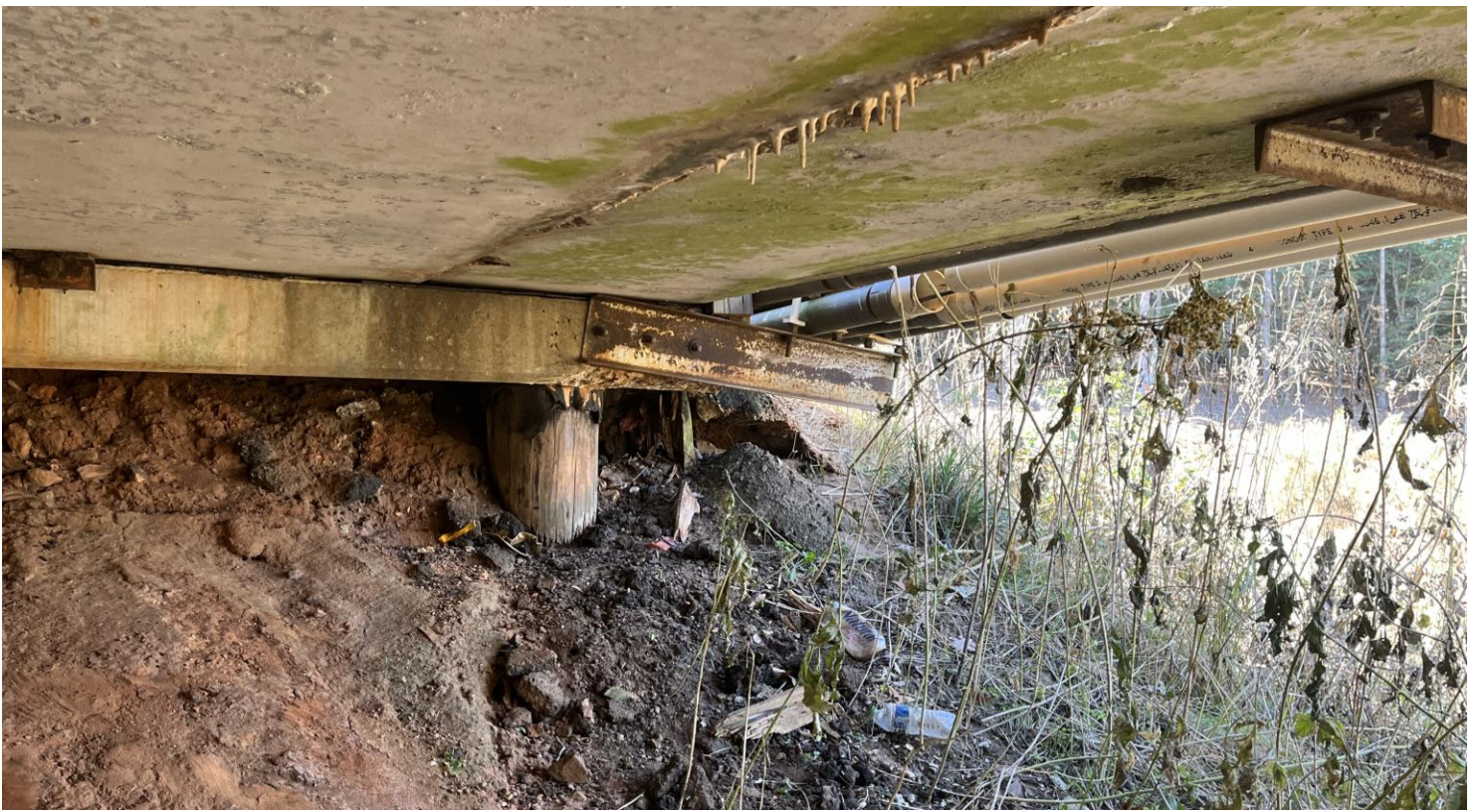
PHOTO # 5 View of LP-1 silver paint on structural pipe brace.
