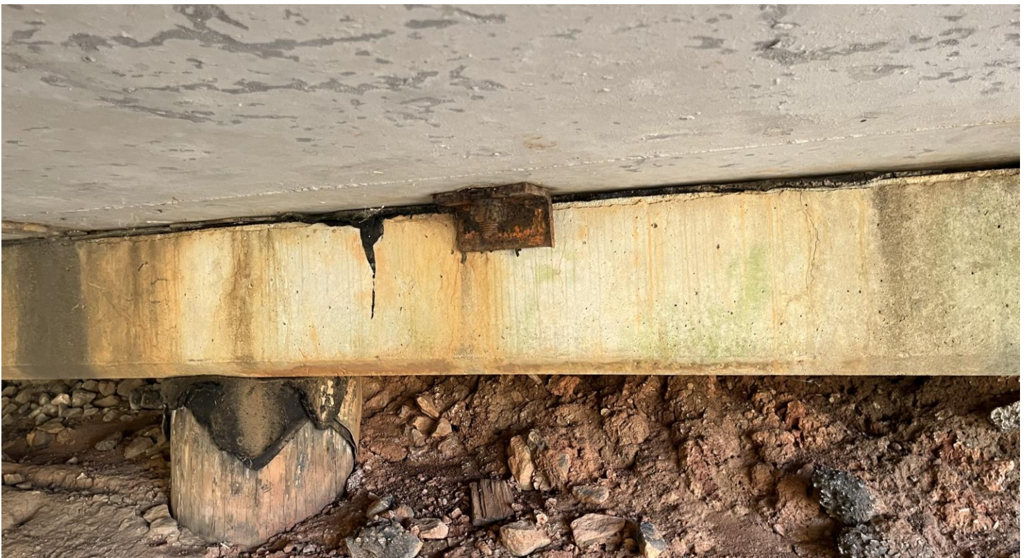
PHOTO # 6 View of LP-2 orange paint on metal decking bracket.
