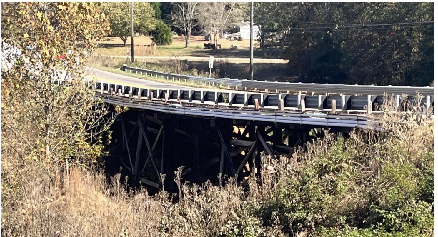
PHOTO # 2 View of the bridge facing northeast.
