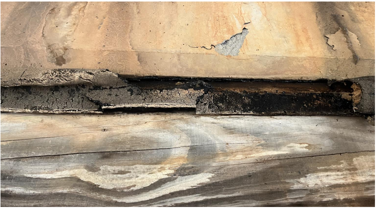
PHOTO # 3 View of HA #1 thick shingle and tar friction barrier
