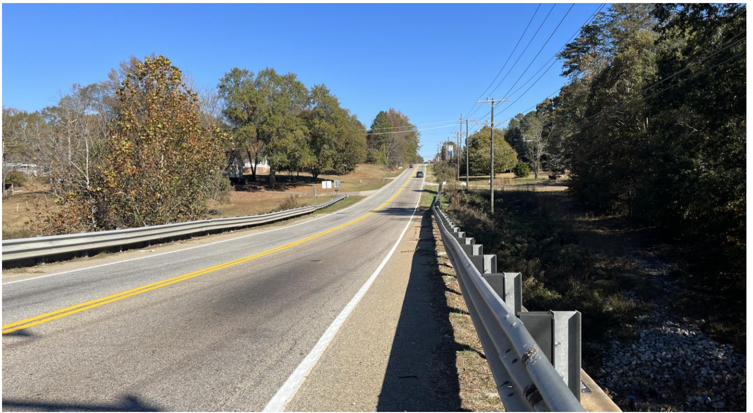
PHOTO # 1 View of the bridge facing north with LP-3 (White Paint) and LP-4 (Yellow Paint) in view.
