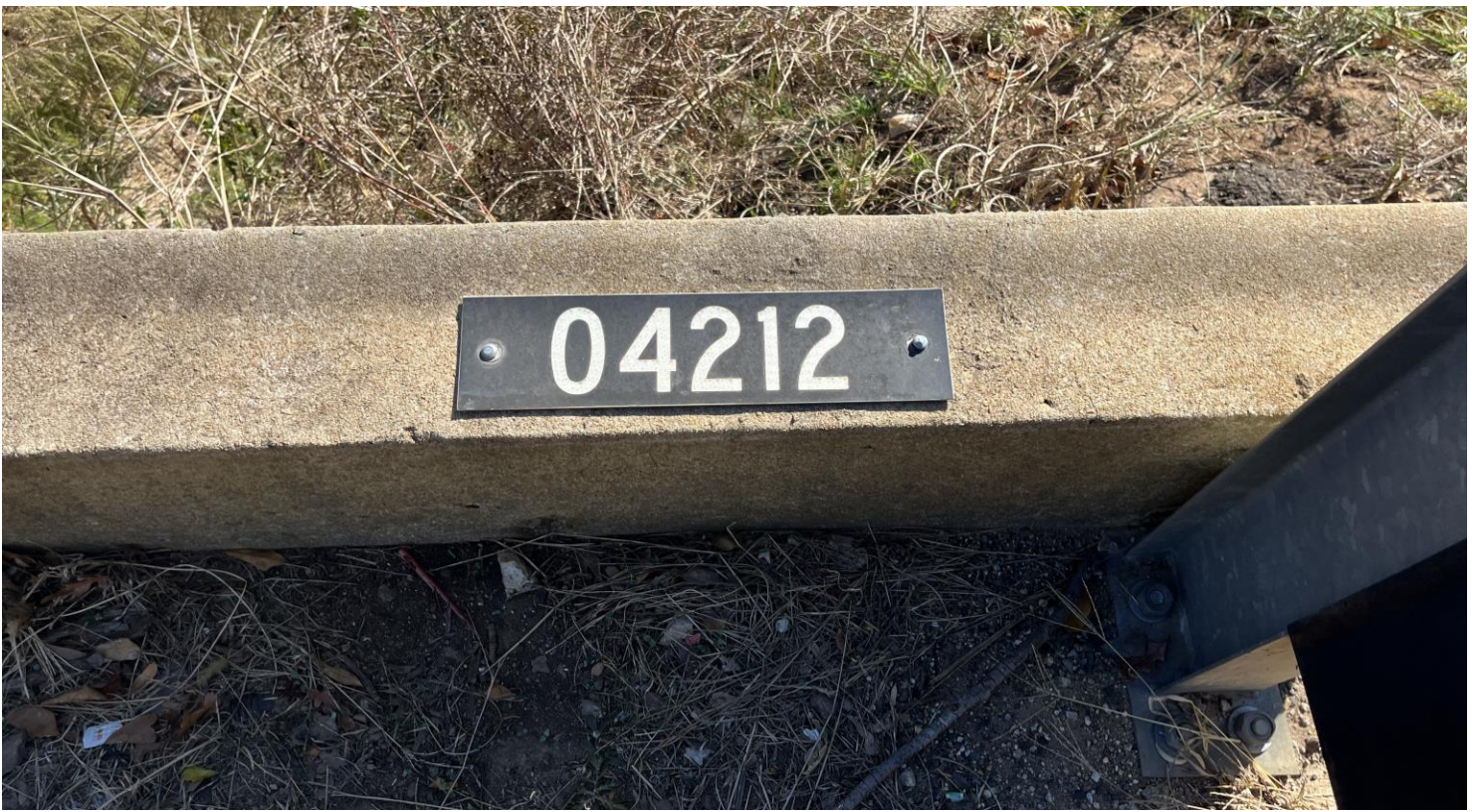
PHOTO # 7 View of the bridge asset number.
