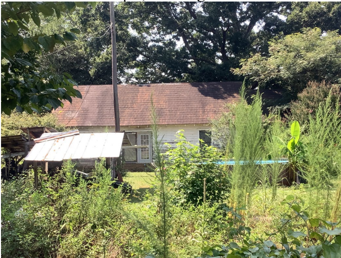
c. North Elevation Detail, Looking South
