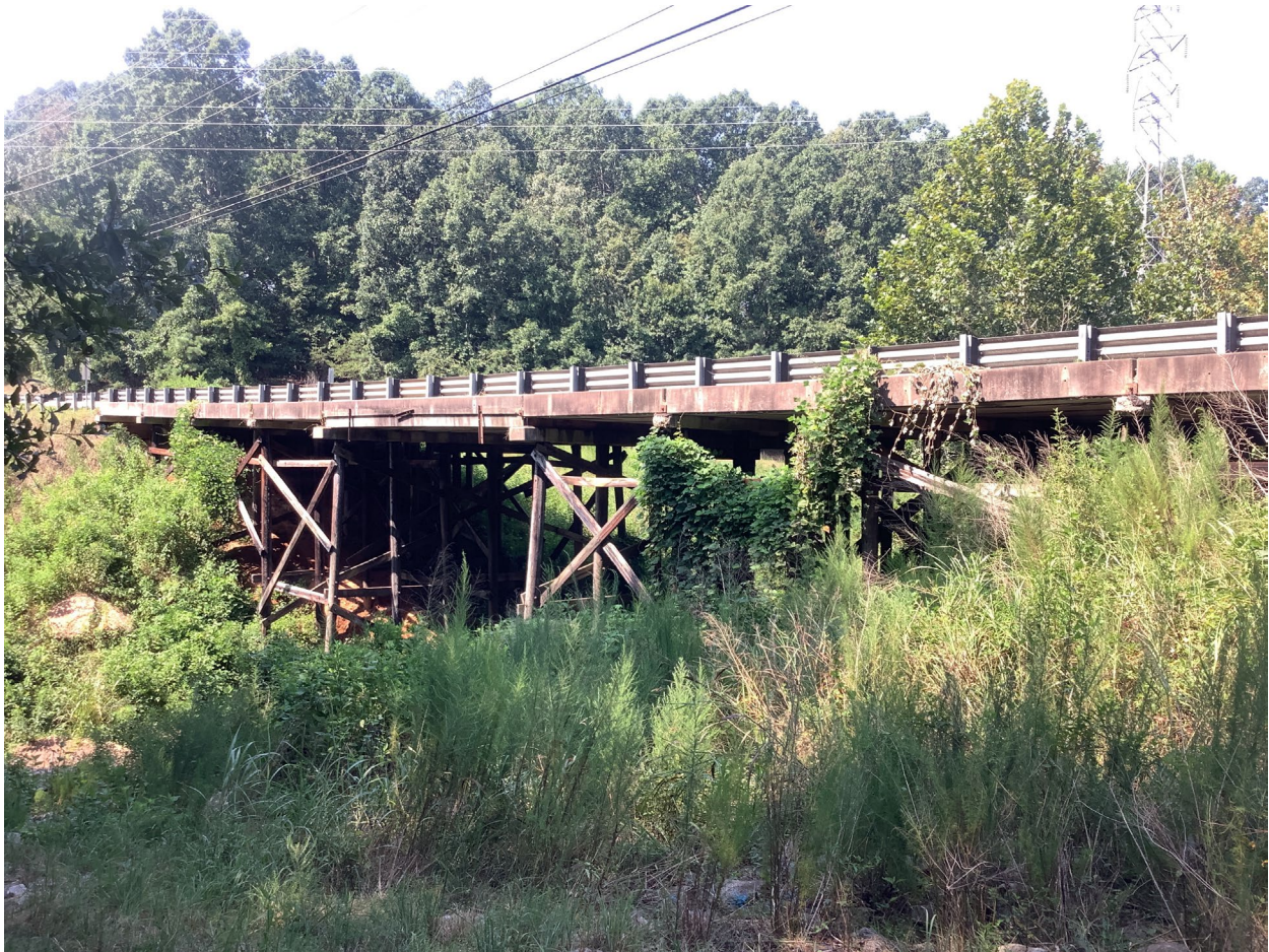
Figure 10. S-42-31 Bridge over Peters Creek, Built 1963 and Not Assessed
