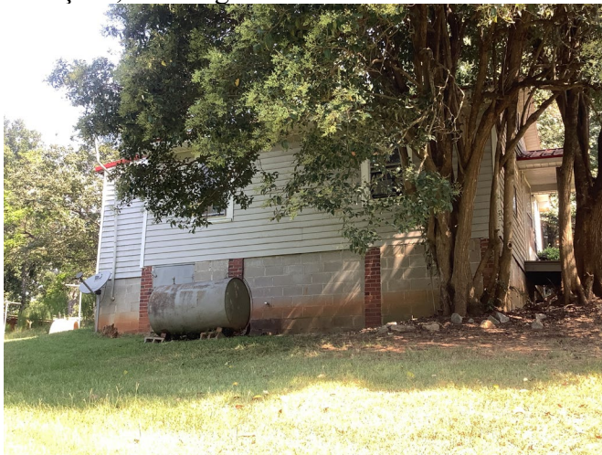
c. South Elevation Detail, Looking Northwest
