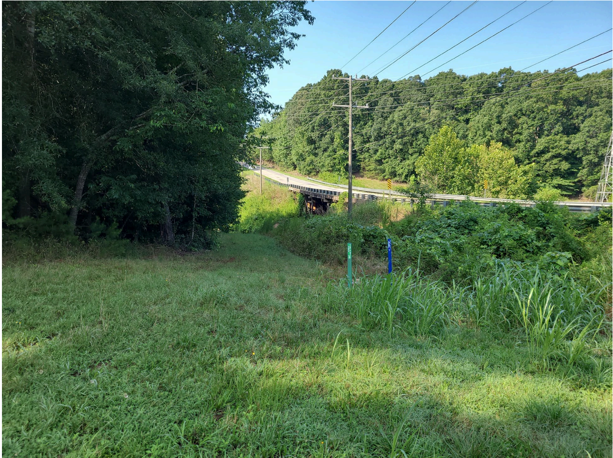
Figure 3. Slope to the Peter's Creek Bridge, Looking South
