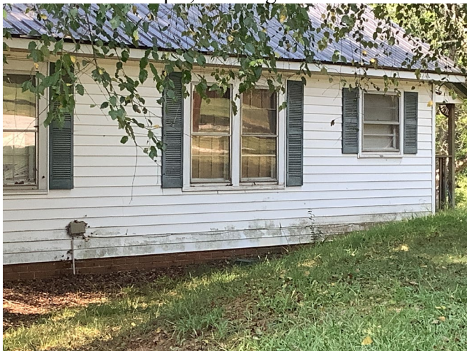
c. North Elevation Detail, Looking Southwest
