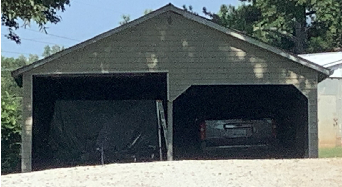
b. Façade Detail, Looking West
