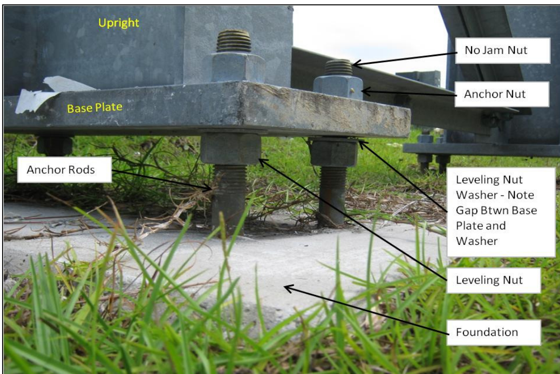
FIGURE 3.2 FOUNDATION ELEMENTS
