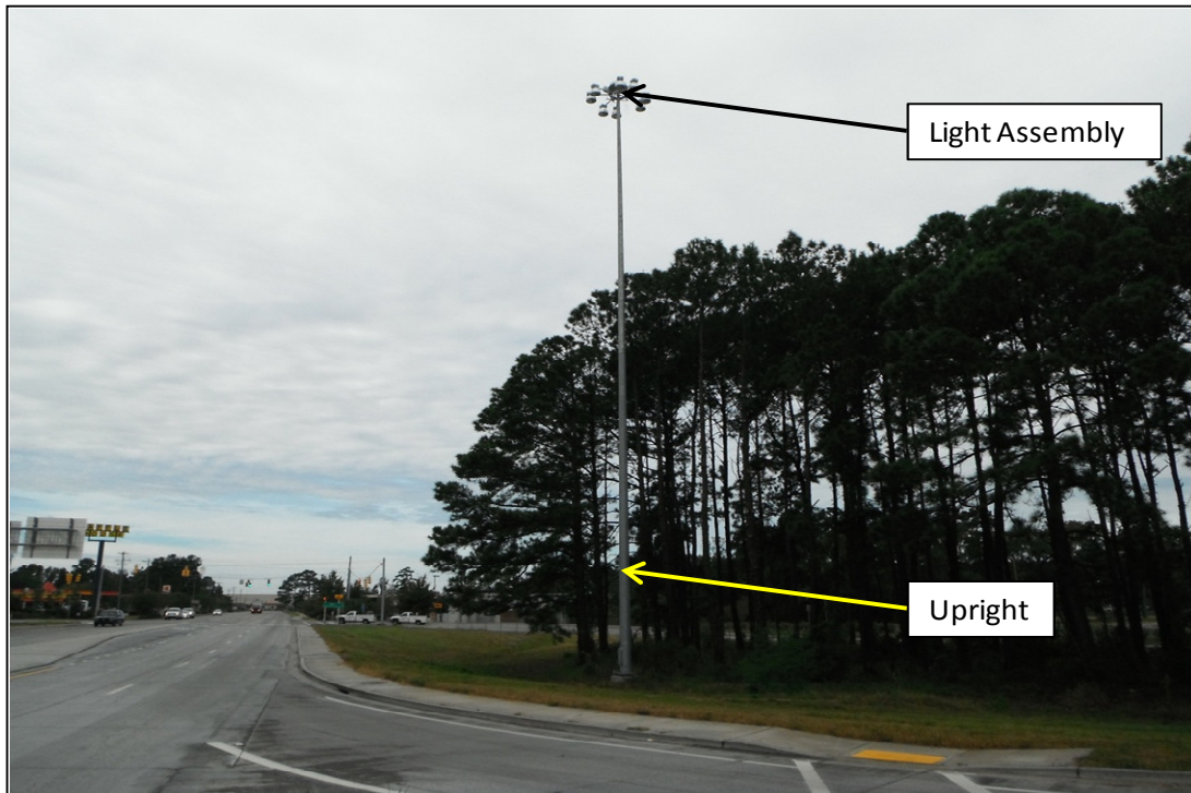
FIGURE 3.19 HIGH MAST LIGHT POLE COMPONENTS
