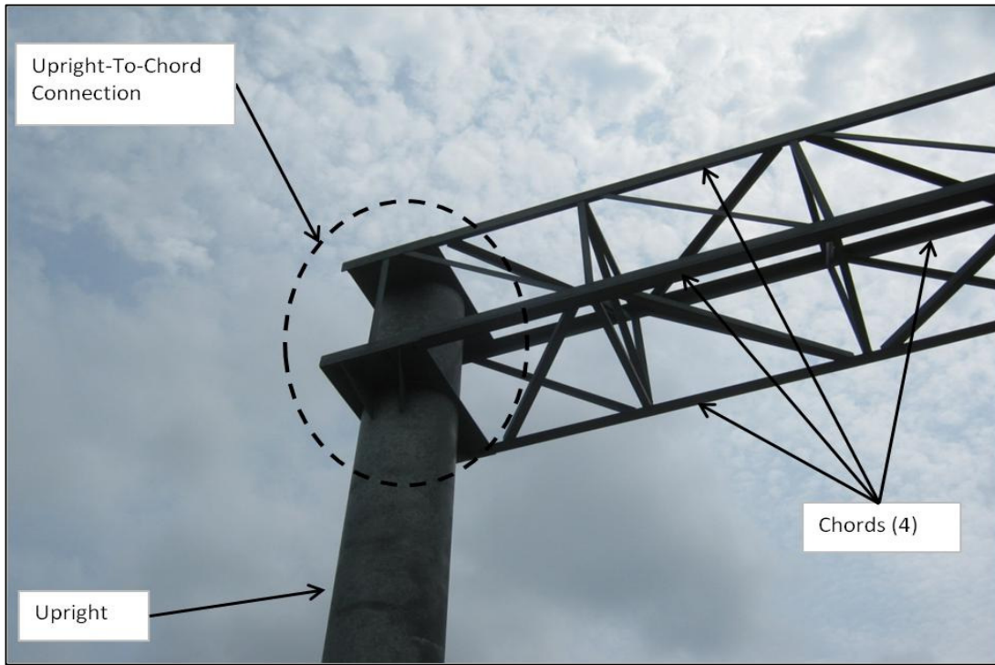
FIGURE 3.5 UPRIGHT AND SPAN ELEMENTS
