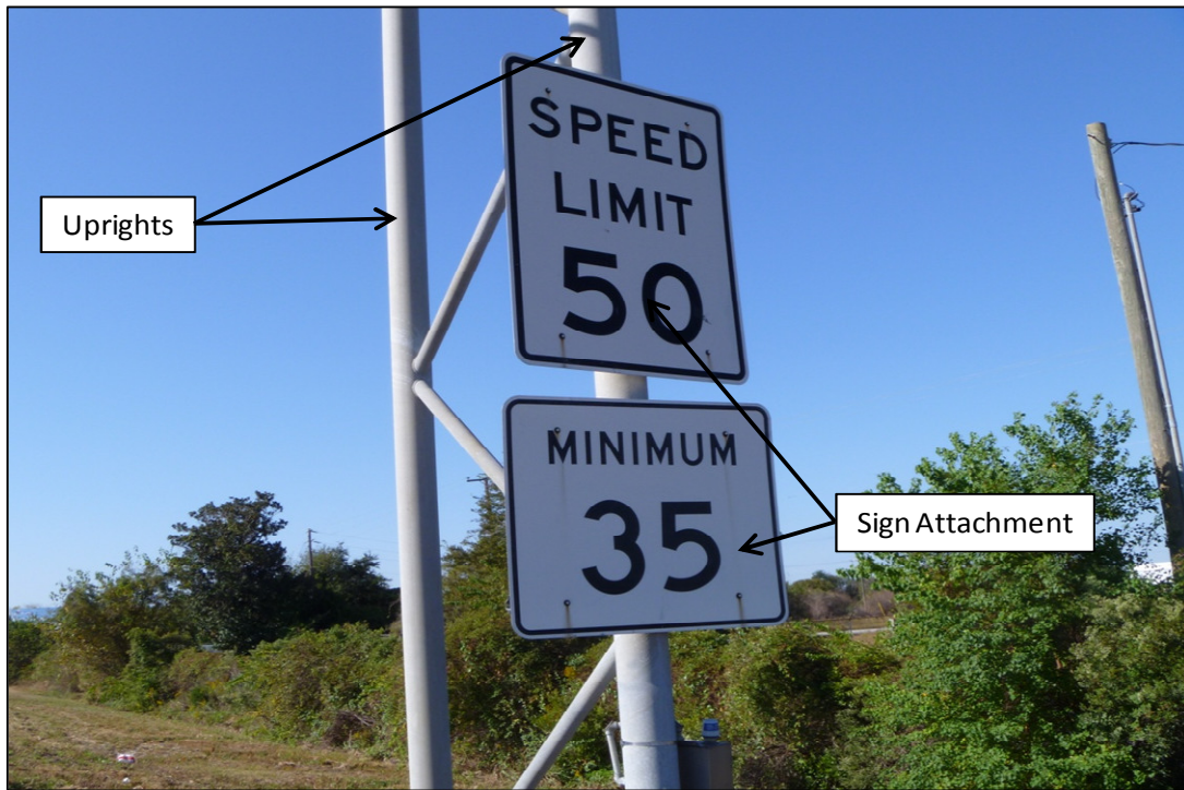
FIGURE 3.15 SIGN ATTACHMENT ELEMENT
