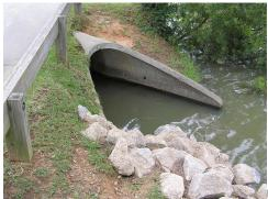
Use Pipe Flared End Section when specified in the plans
