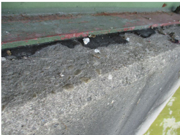
Photo 5. Non-ACM Repair Bond Break Bearing Pad.
