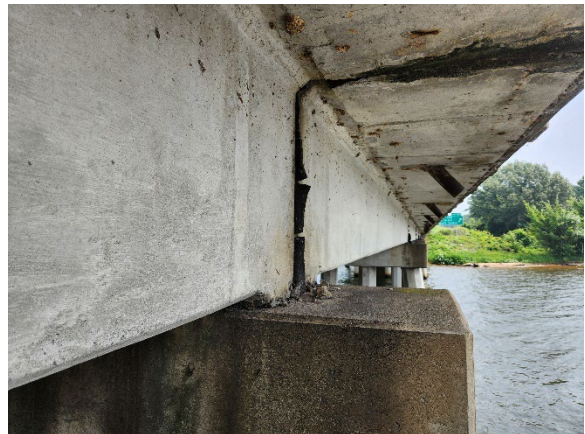
Photo 6. Non-ACM Expansion Joint Material.
