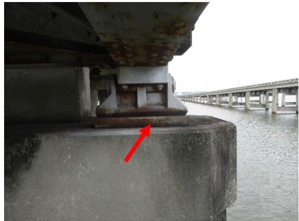
Photo 4. LBP on Gray Bearing Plate under Rocker Bearing on South End of Bridge #6.
