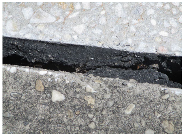
Photo 6. Non-ACM Expansion Joint Material.
