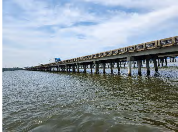
Photo 2. Northeast View of I-95 NBL Bridge #2.
