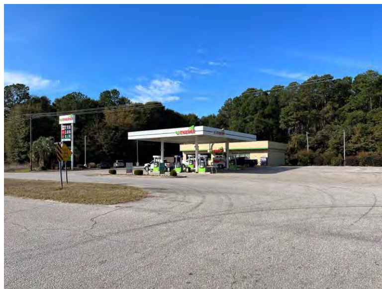
View of Parcel 37, identified as EZ Shop #24 / EZ Shop 24 / ENK 889 / Easy Shop 24 / Enmarket within EDR regulatory information, located at 8440 St. Paul Road / Jim Sniffen within the Project Area. This UST/LUST/RGA LUST site is considered CREC 1.
