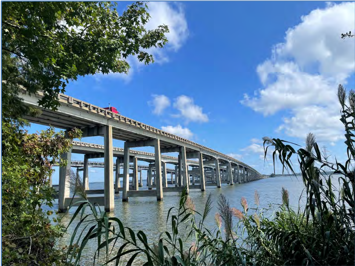
View looking north at the I-95 WJ Gooding main span bridges over Lake Marion.
