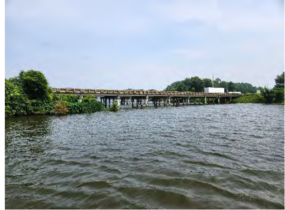
Photo 2. Southeast Corner View of Bridge #1.
