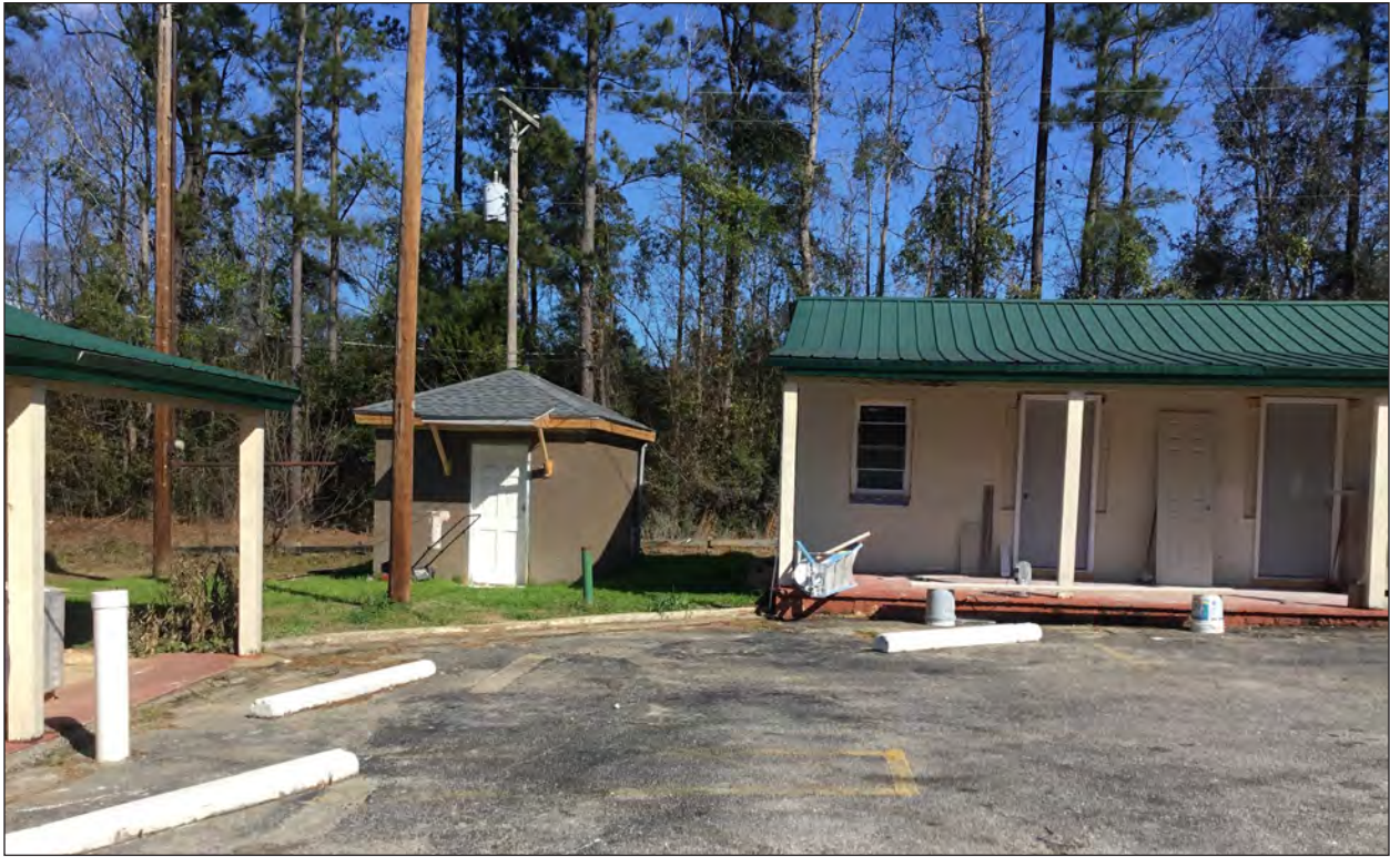
A. Resource 0457.04, Facing Northeast
