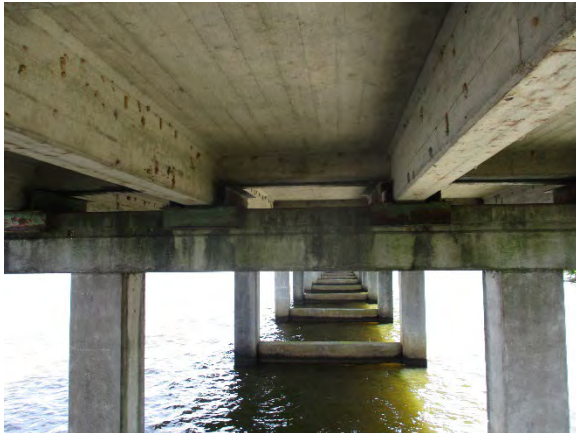
Photo 3. Underside View of US 301/15 Trail Bridge over Lake Marion Overflow.
