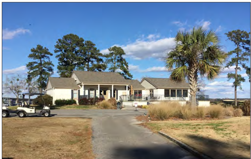
C. Rear Elevation, Facing East
