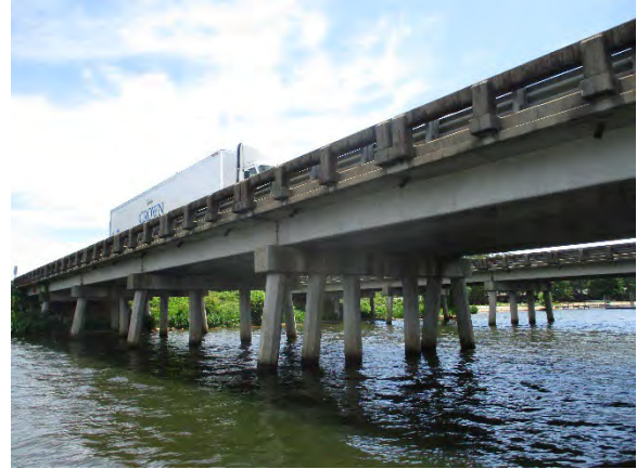
Photo 2. Southwest Corner View of SB I-95 Overflow Bridge #4.
