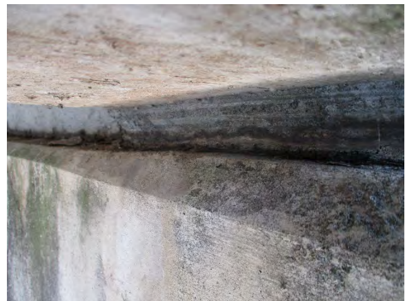
Photo 6. Non-ACM Bond Break Bearing Pad.
