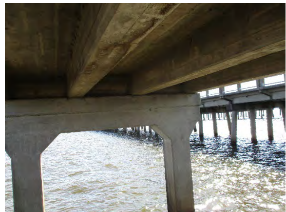
Photo 6. Underside View of Bridge Remnant.
