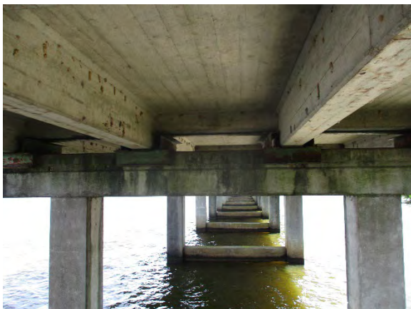
Photo 5. Underside View of Bridge #5.
