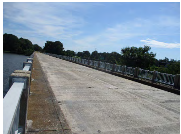
Photo 6. Top Deck View of Bridge #5.
