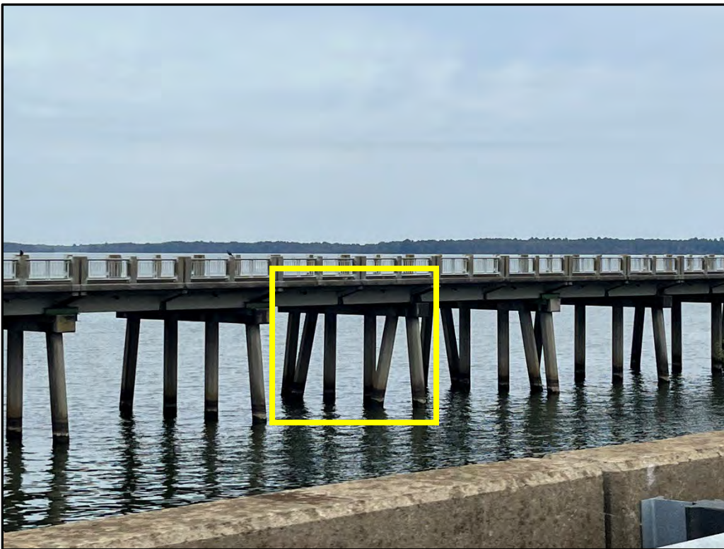
Photo 2. Cylindrical Concrete Piles. Six concrete piles per bent cap.
