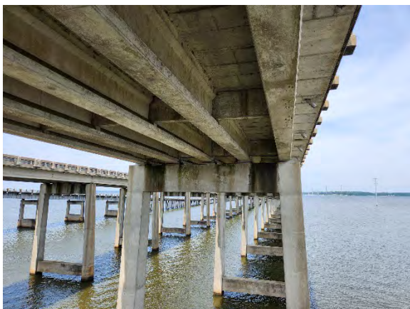
Photo 5. Underside View of Bridge #2.
