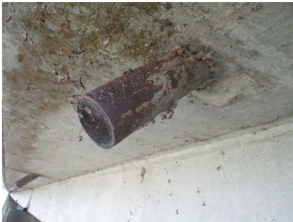
Photo 5. Metal Scupper on West Side of Bridge.
