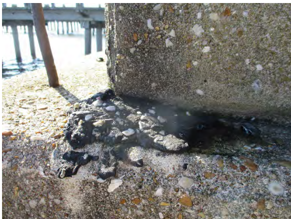
Photo 5. Non-ACM Expansion Joint Sealer.
