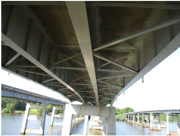
Photo 3. Underside View of Bridge #3.
