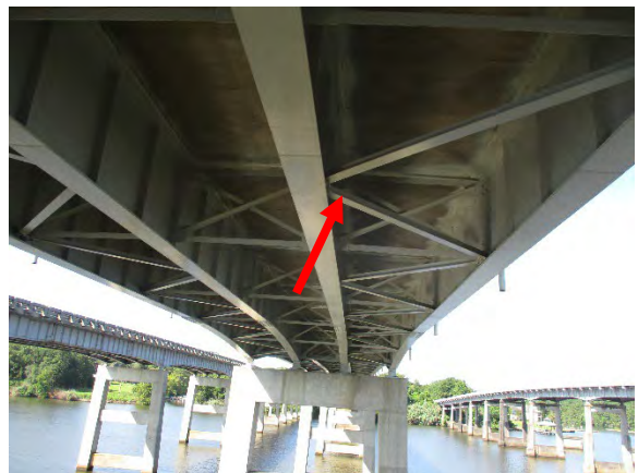
Photo 6. Underside View of Bridge #3.
