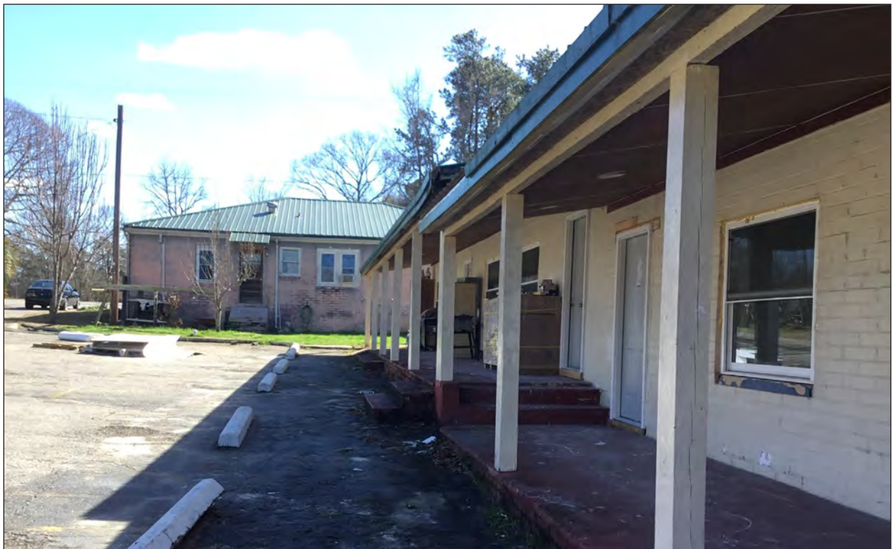
B. Detail, Facing South
