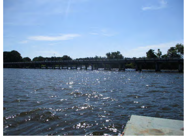
Photo 2. Southwest View of US 301/15 Trail Bridge over Lake Marion Overflow.
