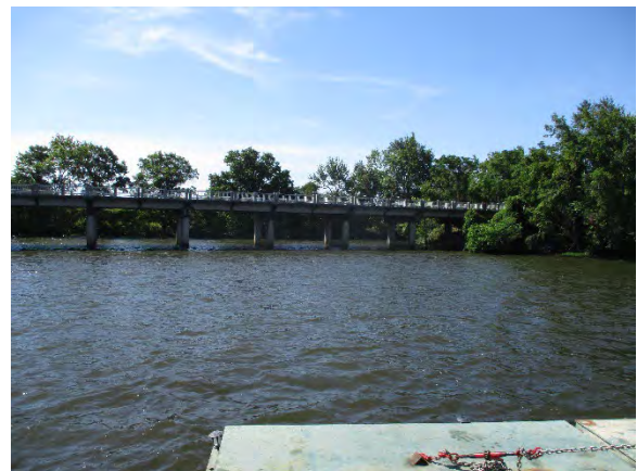
Photo 6. West View of the Southwest Side of Bridge #5.
