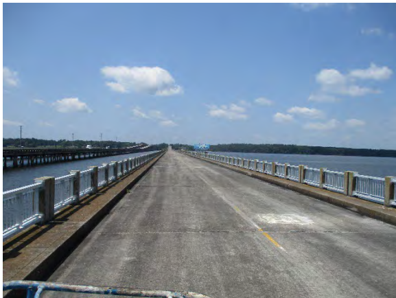
Photo 5. Top Side View of Bridge Deck.
