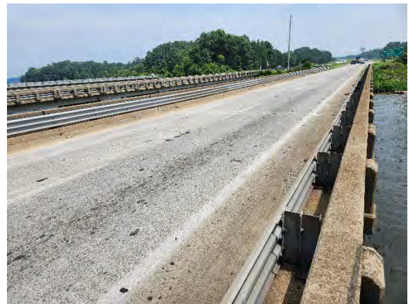
Photo 4. Topside View of Bridge #1.
