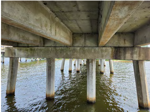
Photo 3. Underside View of NB I-95 NBL Overflow Bridge #1.
