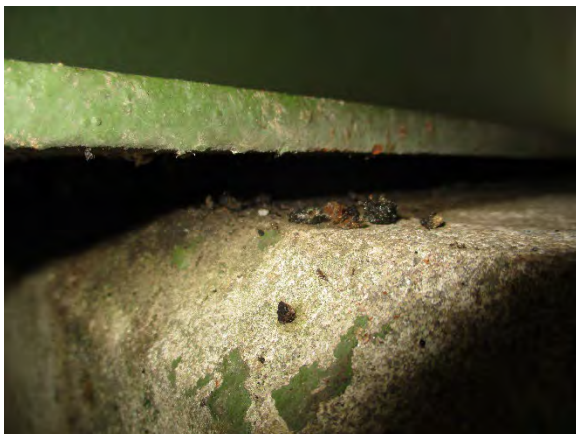
Photo 5. Non-ACM Bond Break Bearing Pad.
