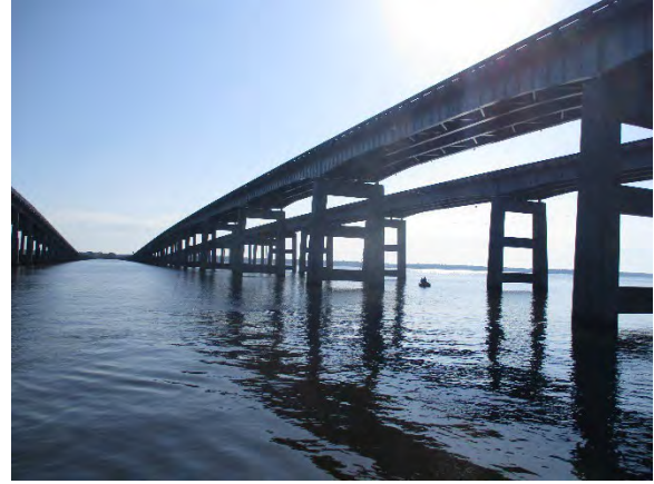
Photo 2. Southwest View of SB I-95 Bridge #3.
