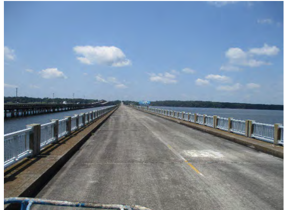
Photo 4. Top View of Bridge Deck.
