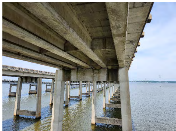
Photo 6. Underside View of I-95 NBL Bridge #2.
