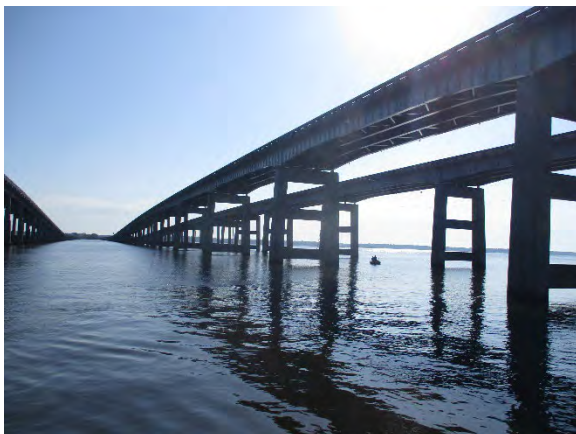
Photo 5. Southwest View of Bridge #3.
