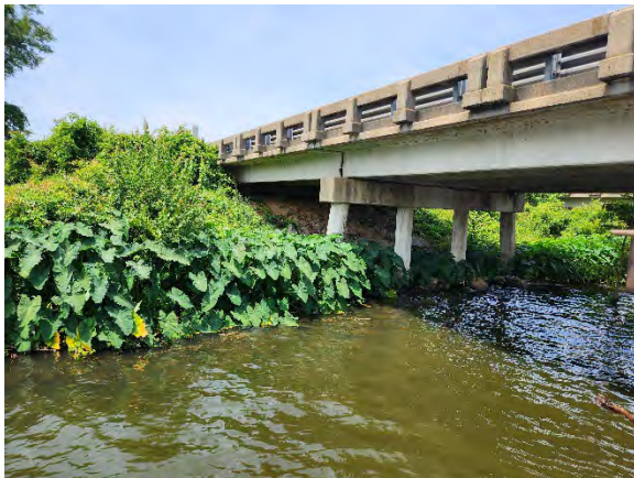
Photo 5. Northeast View of South End Bent.
