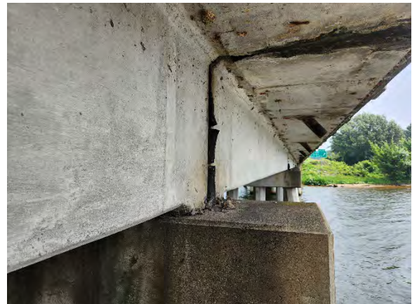
Photo 6. Non-ACM Expansion Joint Material.
