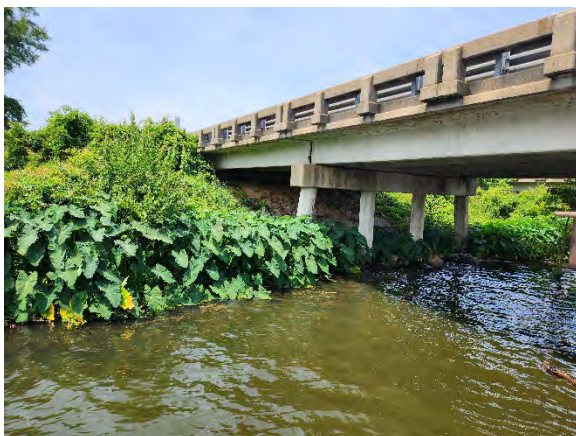
Photo 5. Northeast View of South End Bent.
