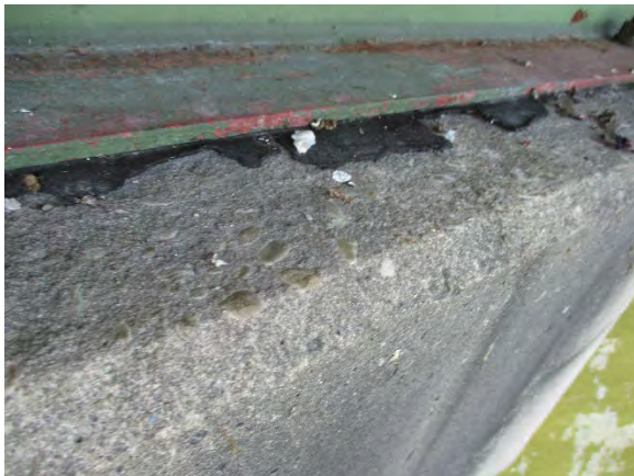
Photo 5. Non-ACM Repair Bond Break Bearing Pad.
