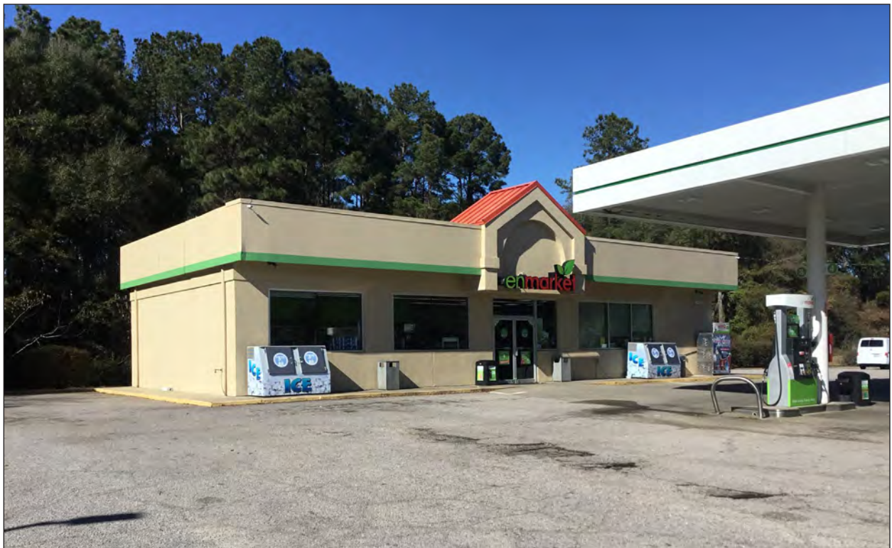
B. Facing Northwest
