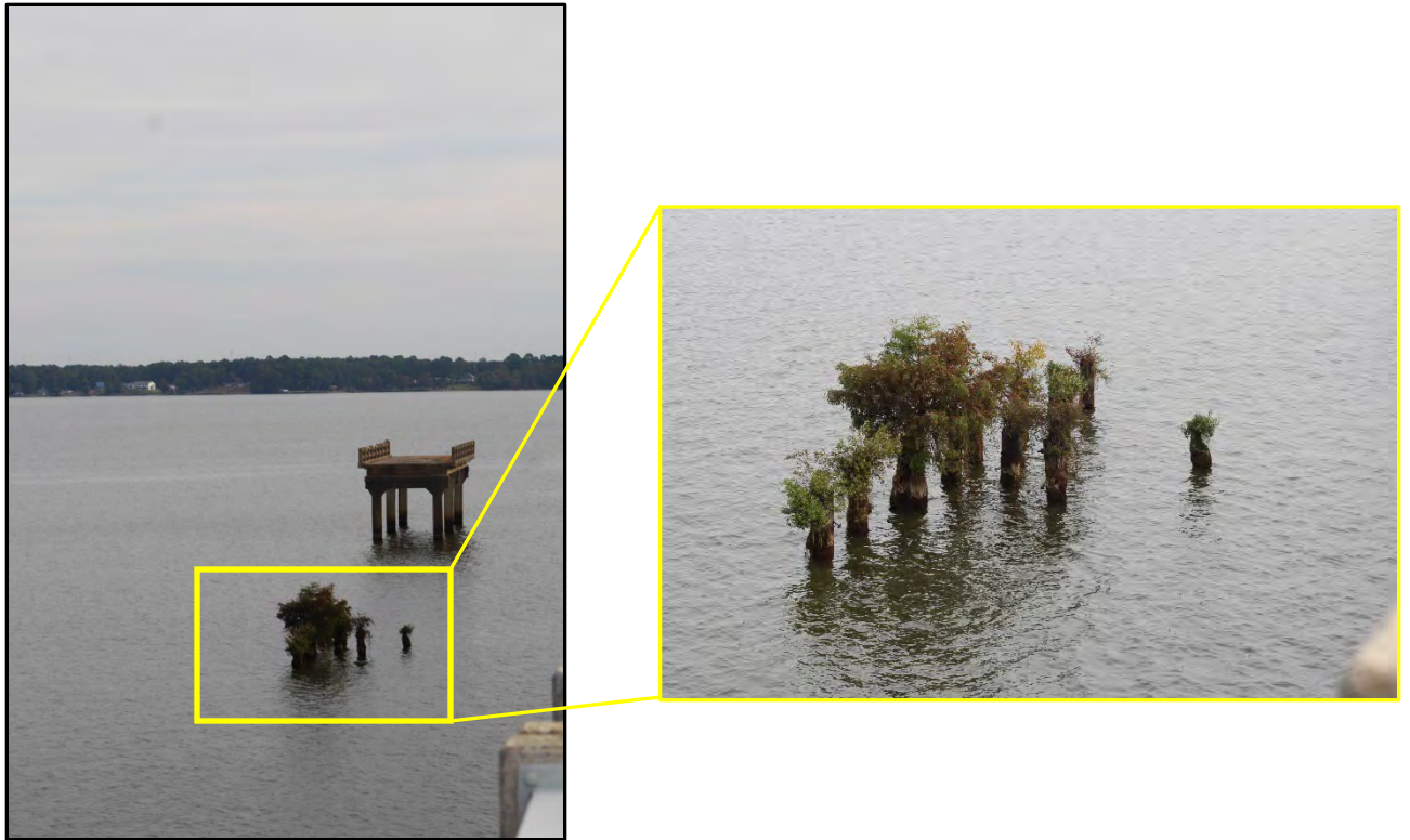
Photo 7. Standalone timber piles west of the US 301 bridge.
