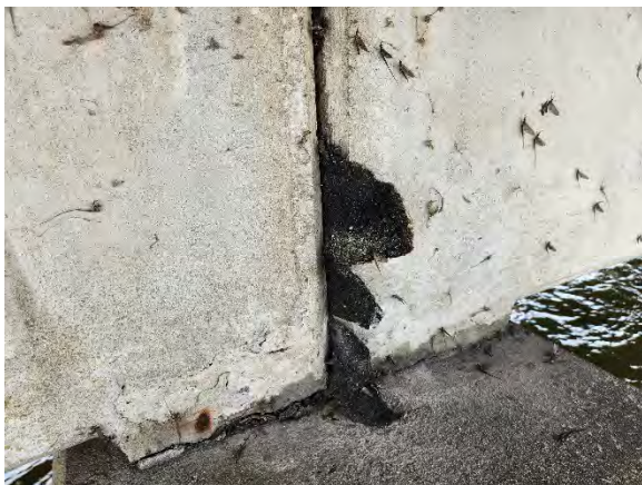
Photo 5. Non-ACM Expansion Joint Material.
