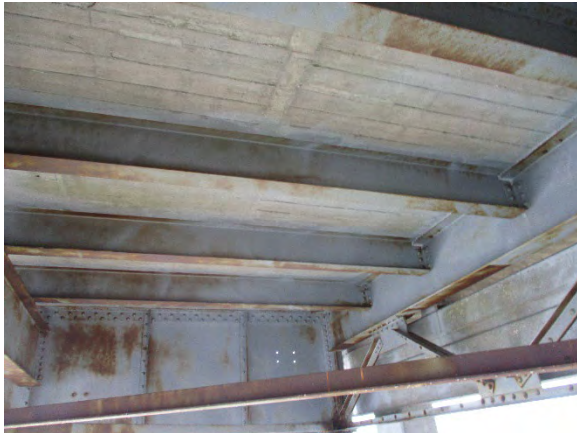
Photo 3. Underside View of US 301/15 Bridge over Lake Marion.
