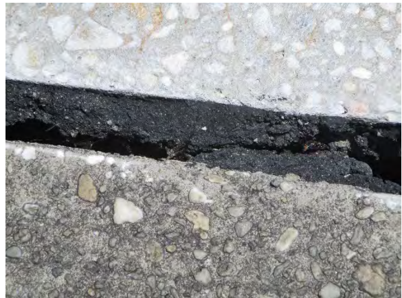
Photo 6. Non-ACM Expansion Joint Material.
