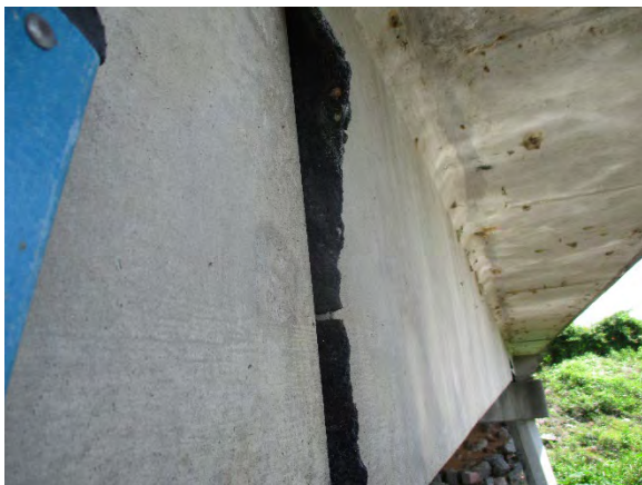
Photo 5. Non-ACM Expansion Joint Material.
