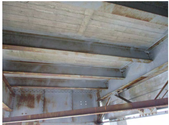
Photo 6. Underside View of Bridge #6.
