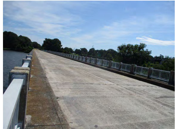
Photo 4. Top View of Bridge Deck of Bridge #5.
