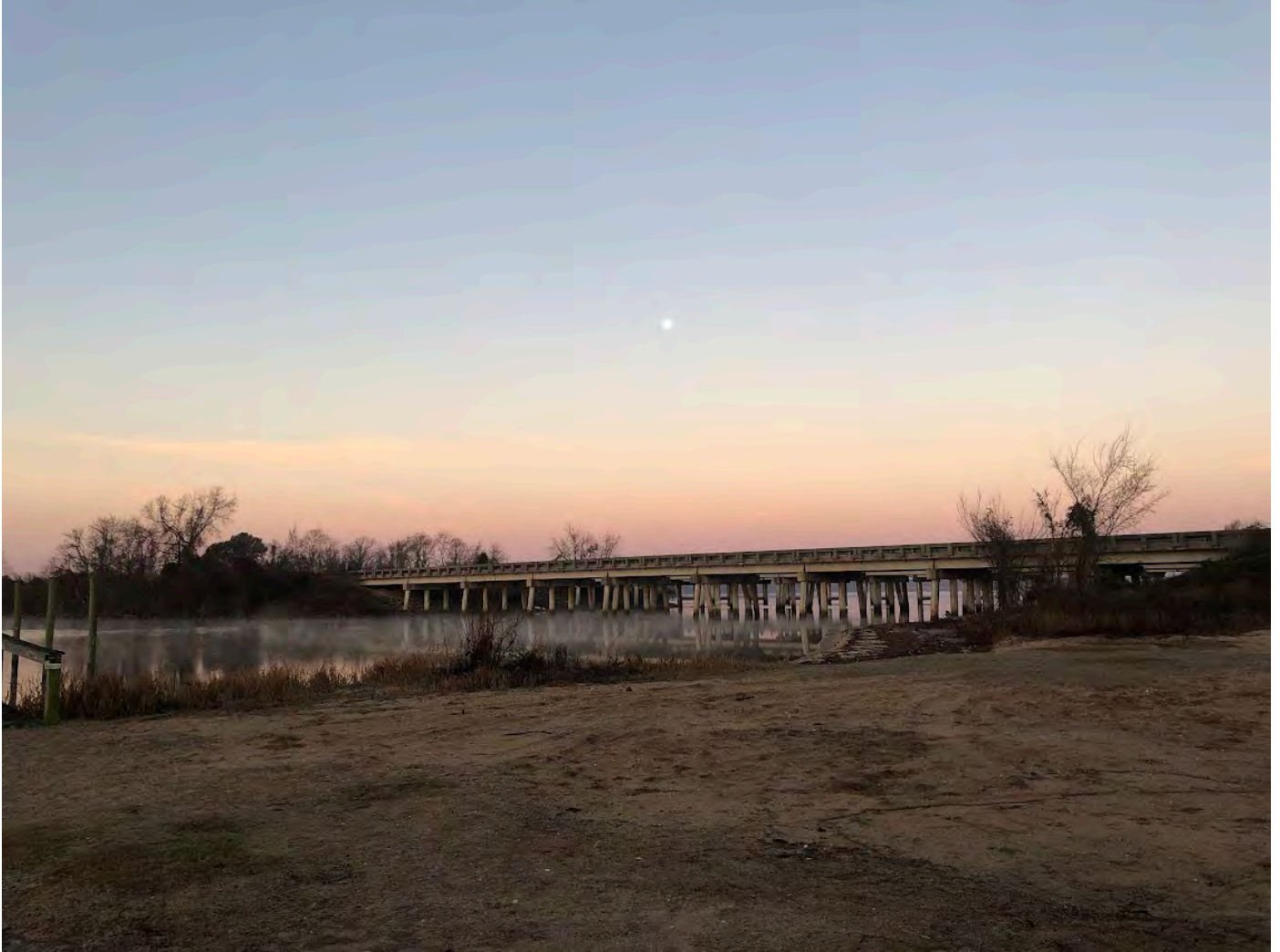
Plate 5. View Southwest of the Northbound Lanes of the I-95 Bridges from the North Shoreline. (Photographer: Lee Cox; Date: February 07, 2023).
