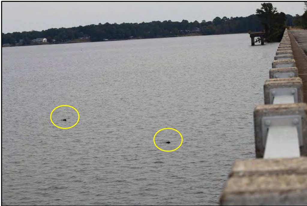
Photo 8. Standalone timber piles west of the US 301 bridge in the lake channel.
