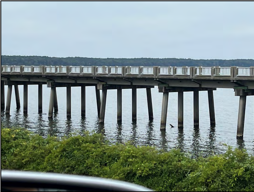
Photo 1. Cylindrical Concrete Piles. Four concrete piles per bent cap.
