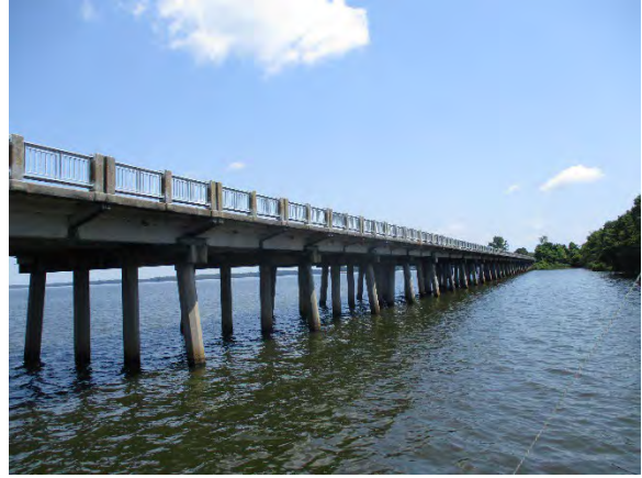
Photo 2. Southeast View of US 301/15 over Lake Marion.
