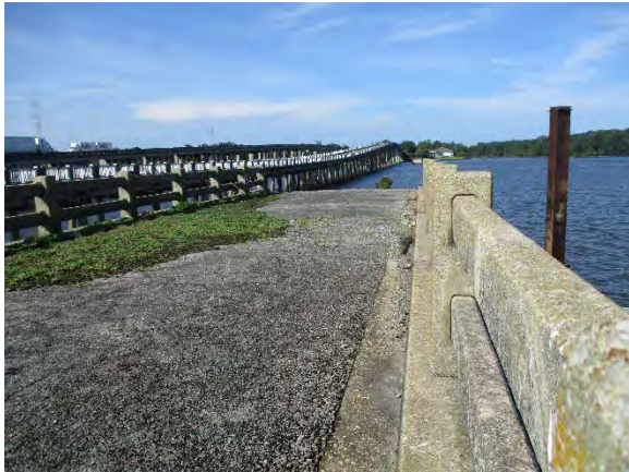
Photo 3. Top View of Deck of Bridge Remnant.
