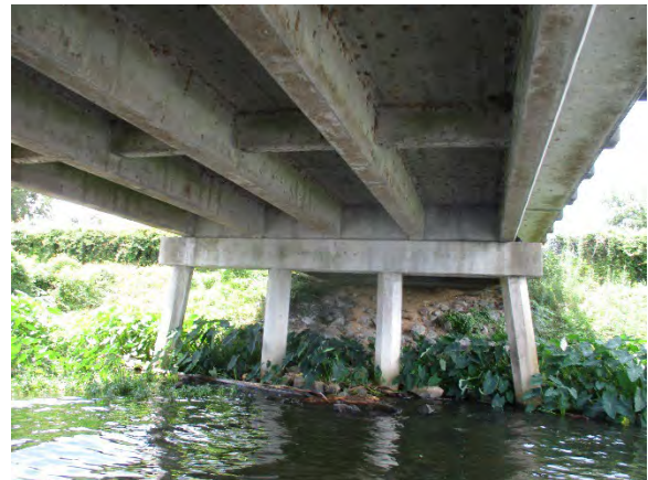
Photo 4. View of South End Bent.
