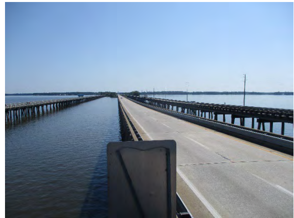
Photo 6. Topside View of Bridge Deck.
