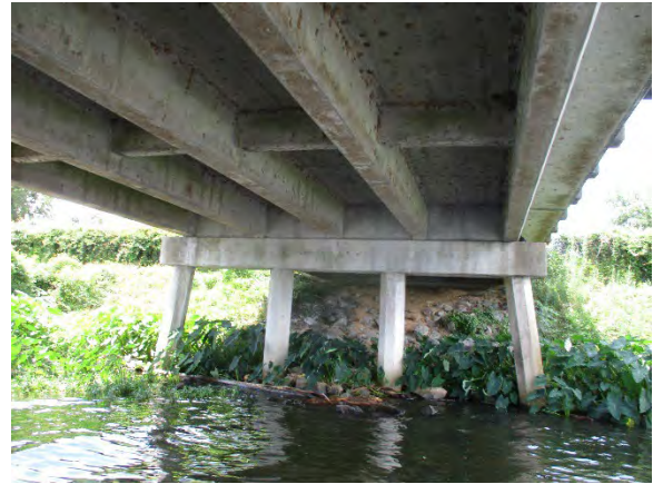
Photo 4. View of South End Bent.
