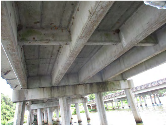
Photo 3. Underside View of SB I-95 NBL Overflow Bridge #4.
