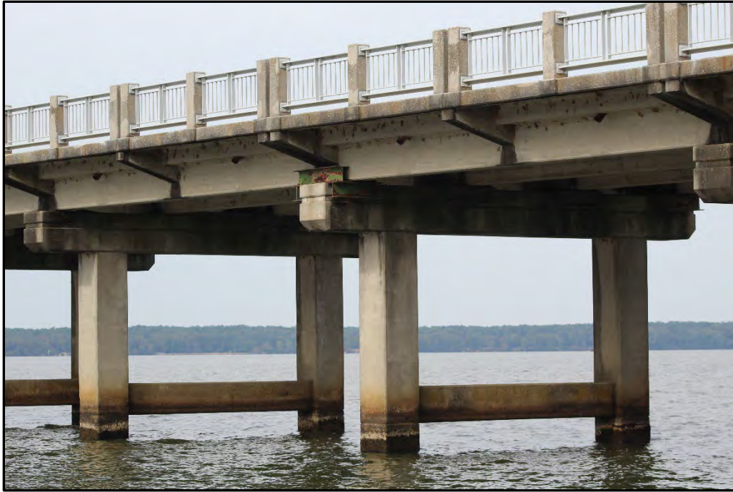
Photo 3. Concrete piles with concrete strut.
