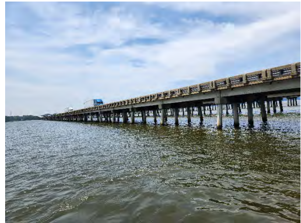
Photo 4. Northeast View of Bridge #2
