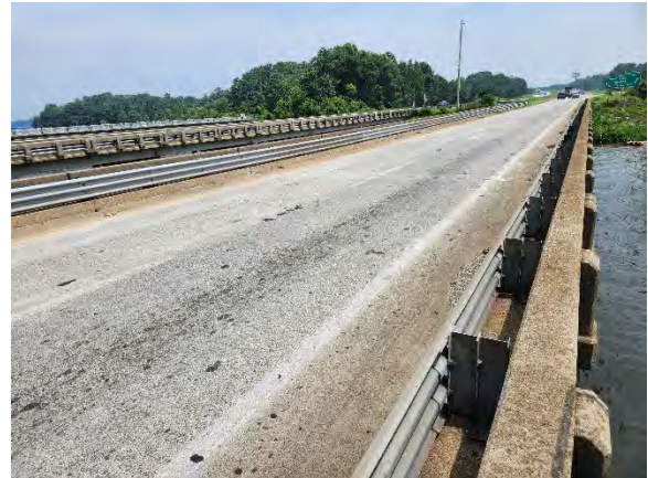
Photo 4. Top View of Bridge Deck.
