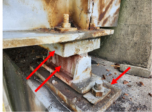
Photo 2. LBP on Rocker Bearing Top Plates, Rocker Bearing and Bearing Plates Associated with Bridge #2.
