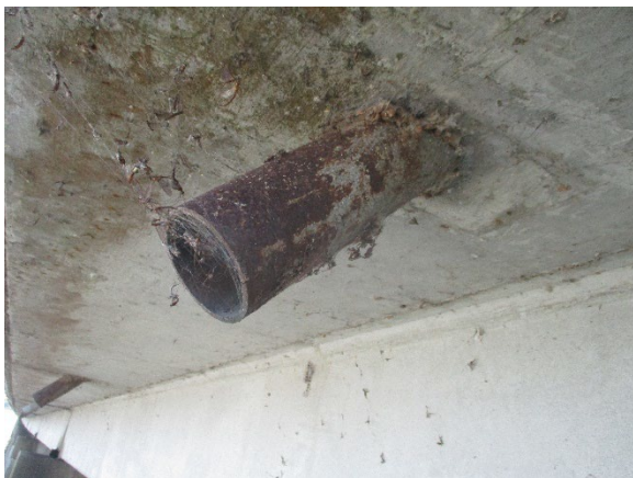
Photo 5. Metal Scupper on West Side of Bridge.
