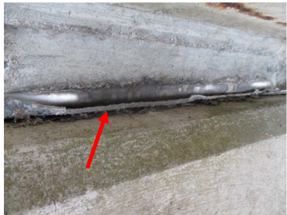
Photo 4. ACM Bond Break Bearing Pad Associated with Bent #28 of I-95 NBL Bridge #2.
