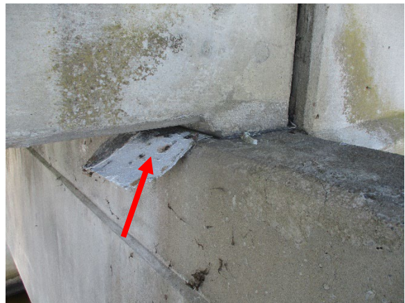
Photo 4. ACM Bond Break Bearing Pad Associated with Bent #28 of I-95 SBL Bridge #3.
