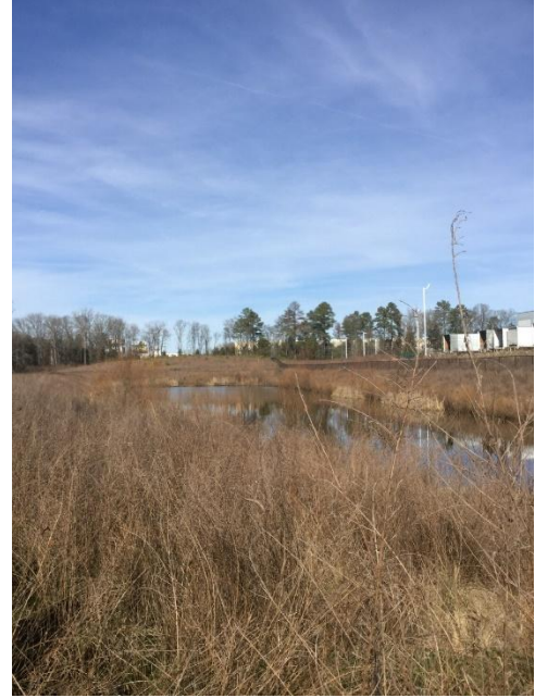
Existing Detention Pond
