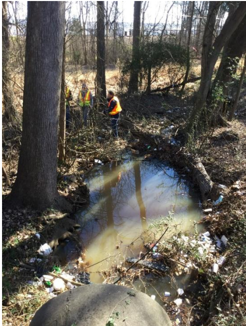
Existing outfall of Ex. 42" RCP
