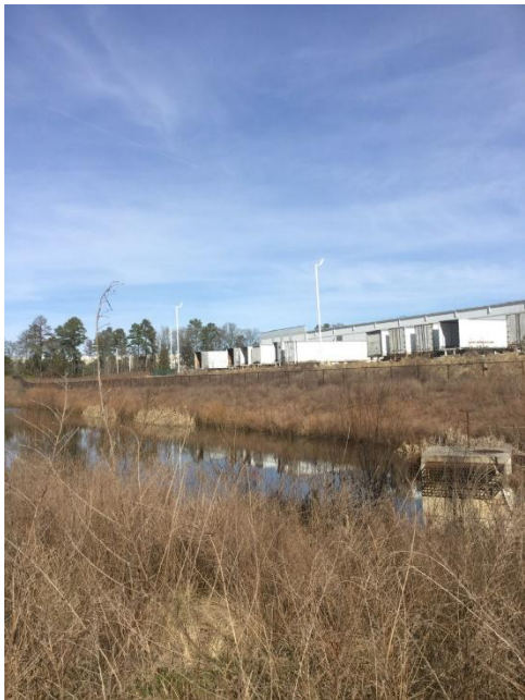
Existing Detention Pond
