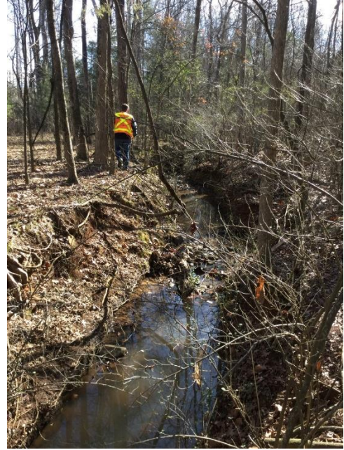
Existing Stream near Pipe 7 proposed outfall
