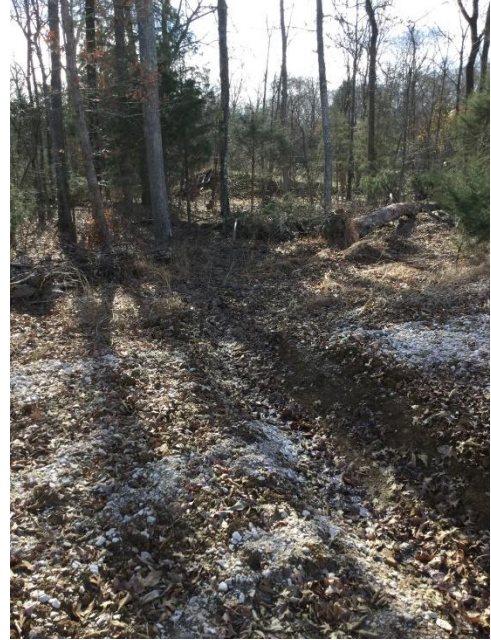
Existing swale near proposed invert in of Pipe 8
