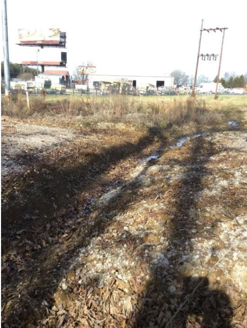
Existing swale near proposed invert in of Pipe 8
