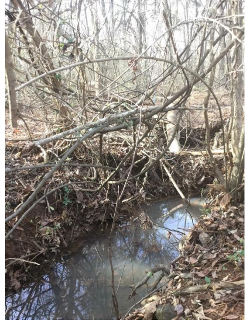
Existing stream from runoff parallel to I-77 coming to Ex. 42" RCP
