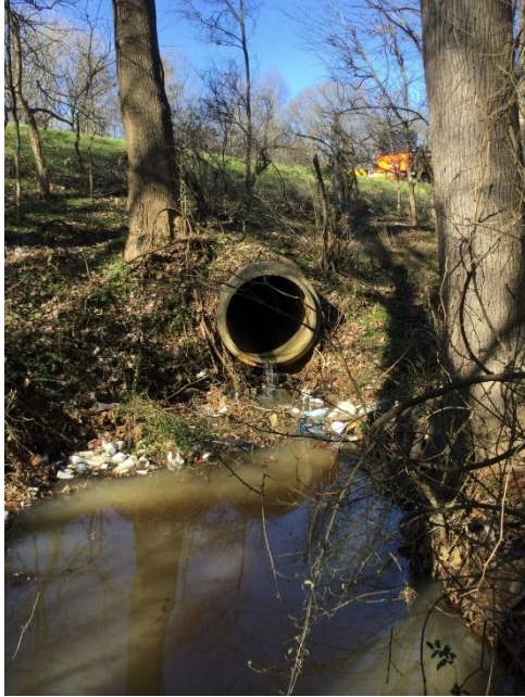
Existing outfall of Ex. 42" RCP
