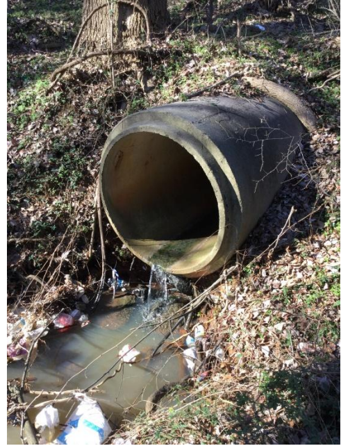
Existing outfall of Ex. 42" RCP
