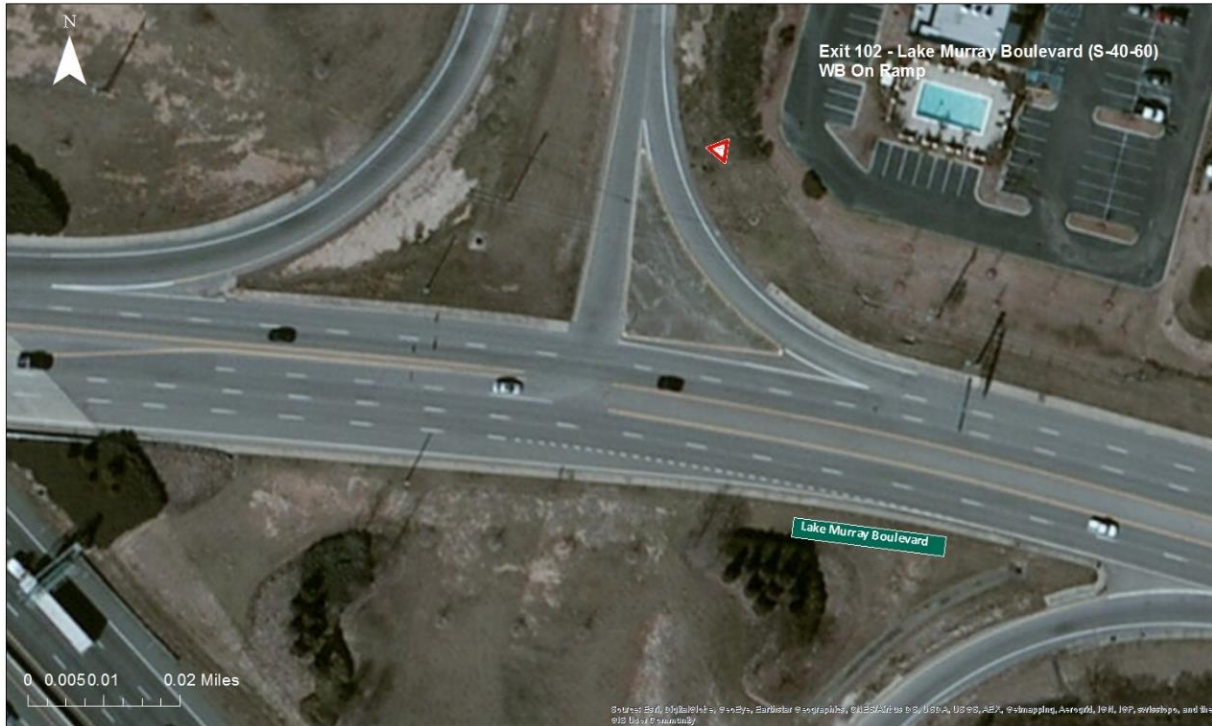
Figure 37 - Exit 102: Lake Murray Boulevard at Westbound On-Ramp
