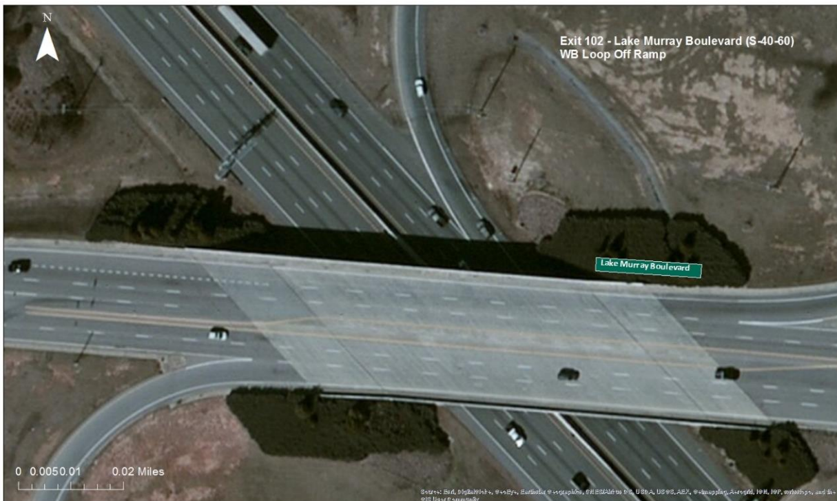
Figure 38 - Exit 102: Lake Murray Boulevard at Westbound Loop Off-Ramp
