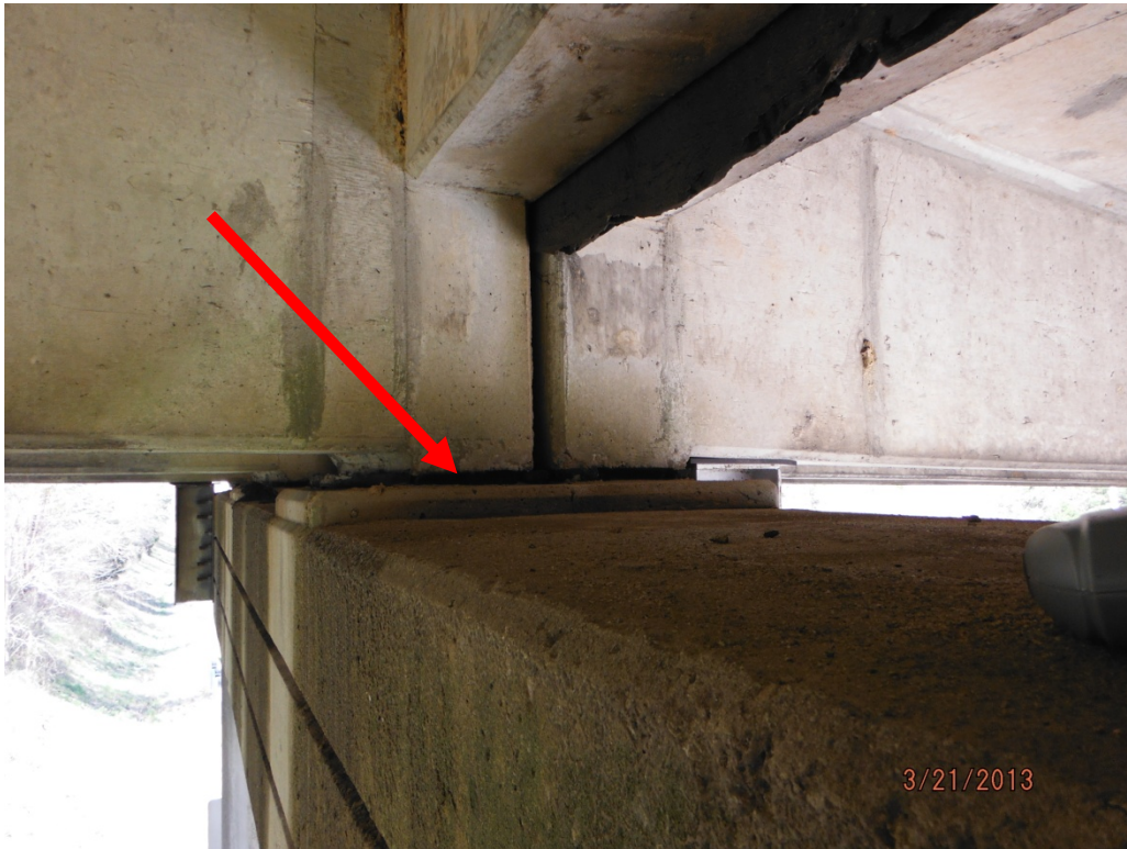
Asbestos-Containing Interior Bent Cap Pads
