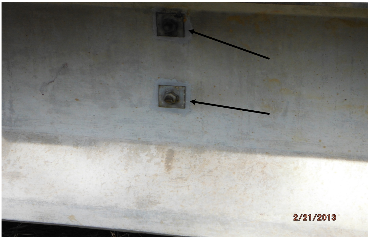
Beam Tie-Rod Assemblies
