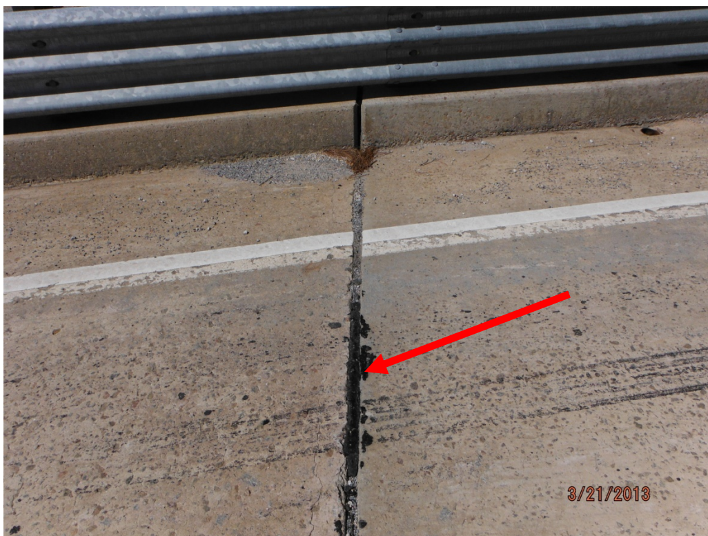
Asbestos-Containing Top of Decking Expansion Joint Material
