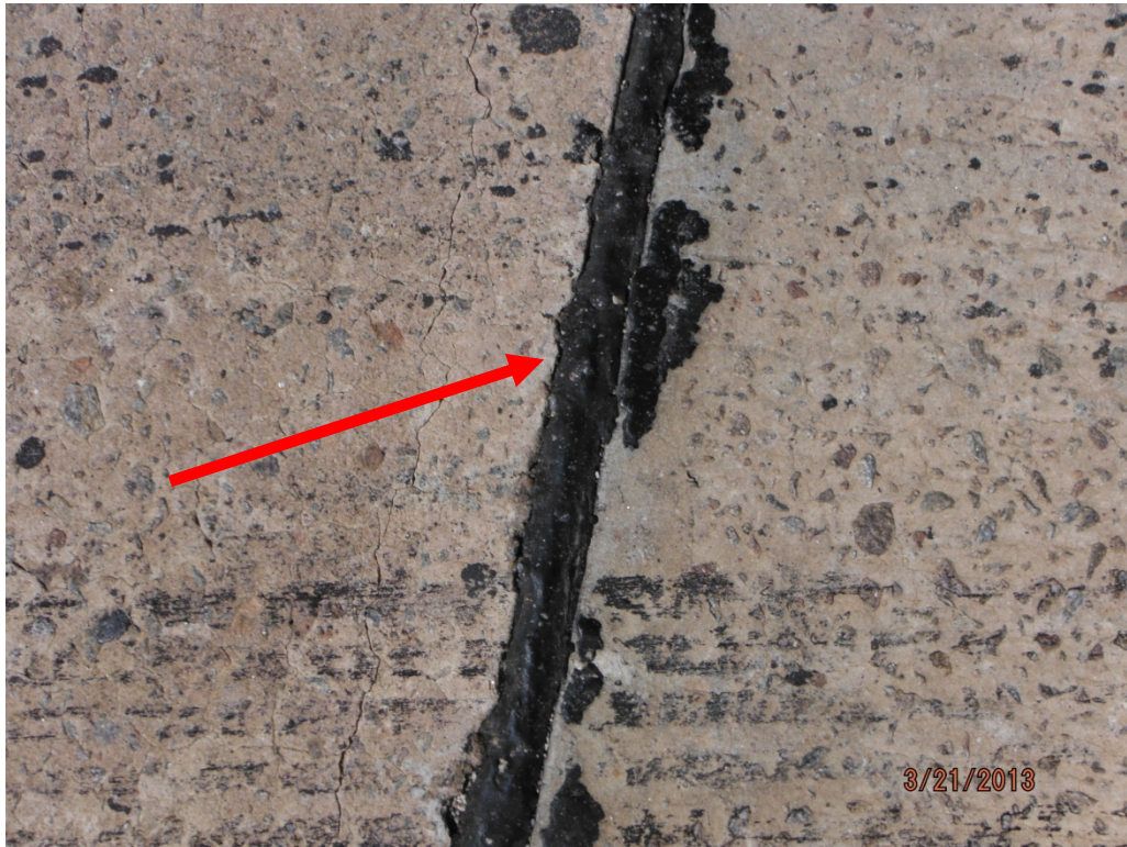
Asbestos-Containing Top of Decking Expansion Joint Material
