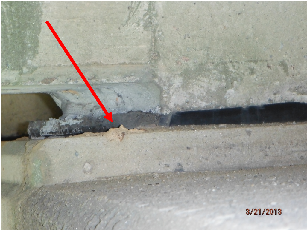
Asbestos-Containing Interior Bent Cap Pads
