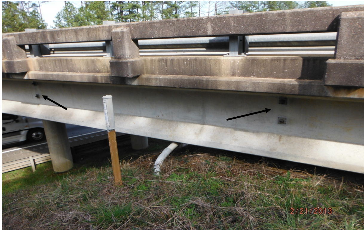
Beam Tie-Rod Assemblies
