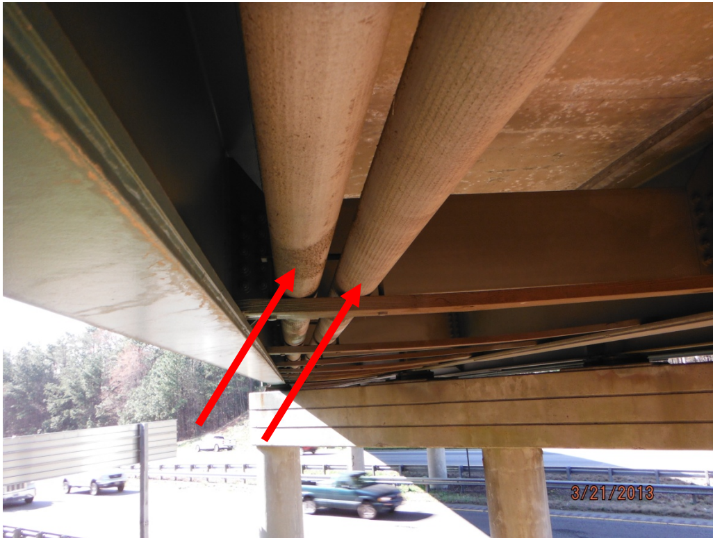
Asbestos-Containing Transite Utility Conduits
