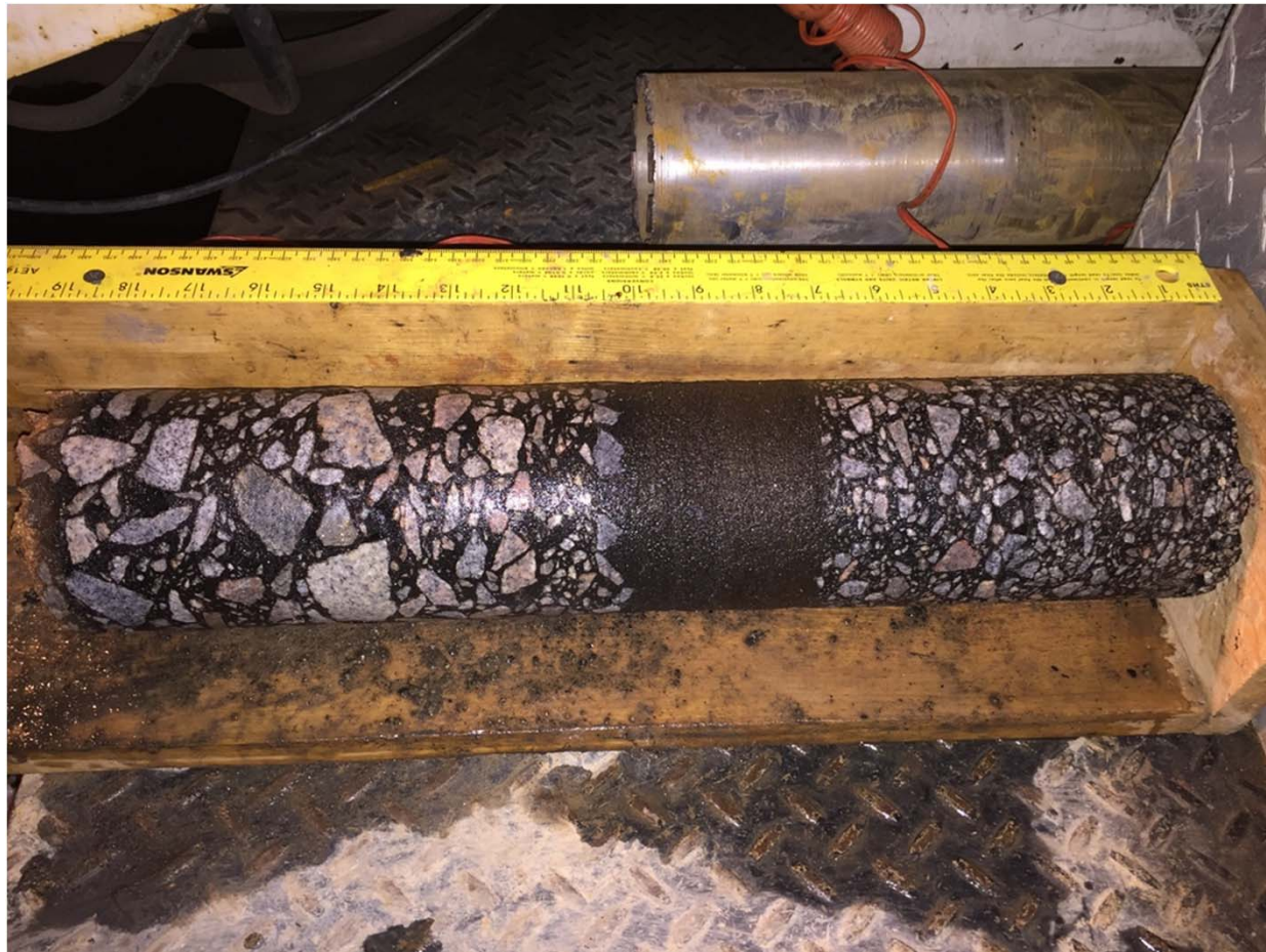
I-26 MM 94.0 westbound outside lane
