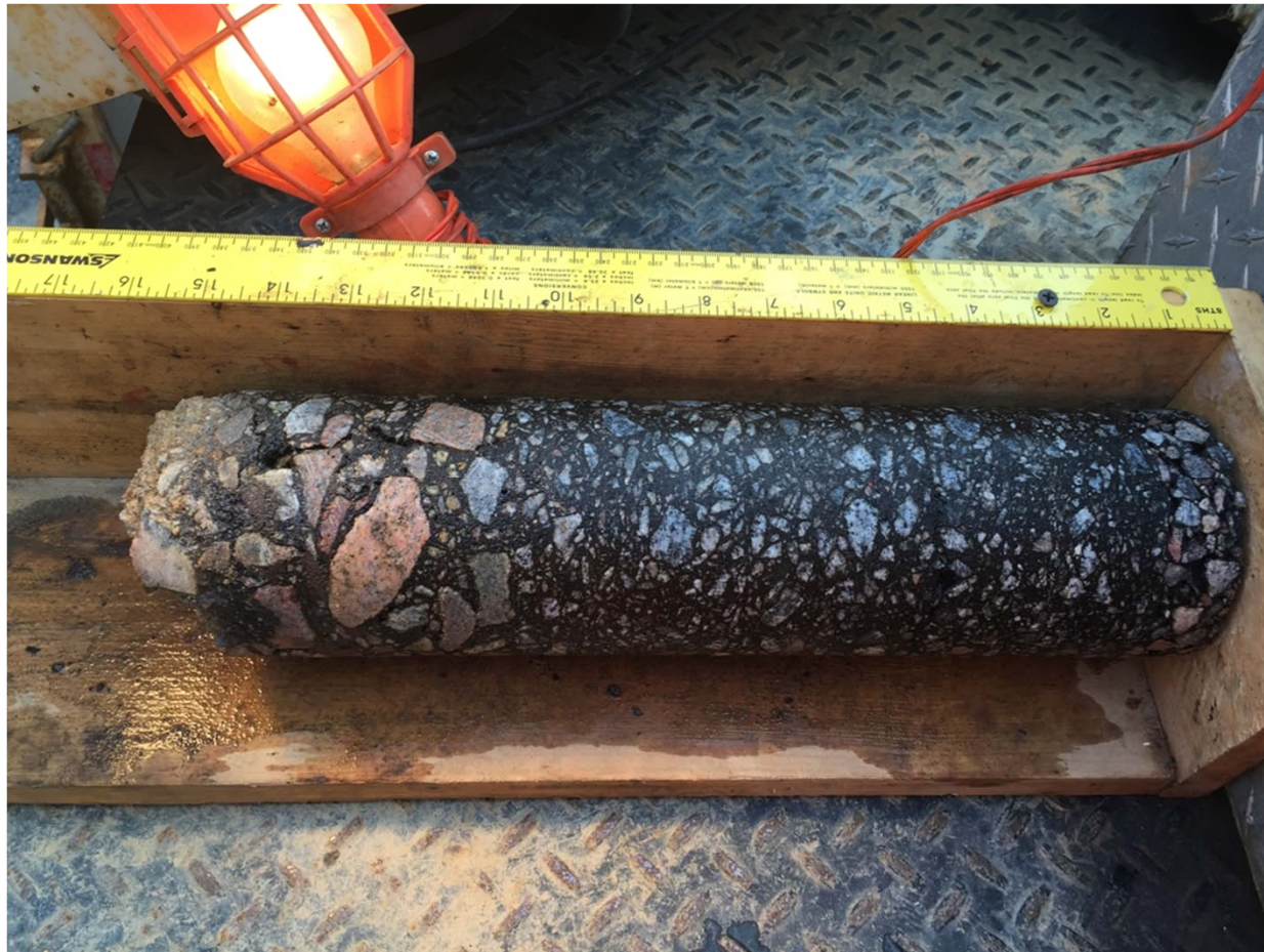
I-26 MM 99.0 westbound outside lane
