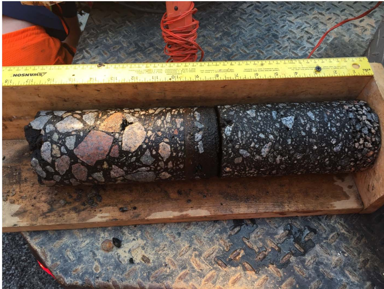
I-26 MM 98.5 westbound outside lane
