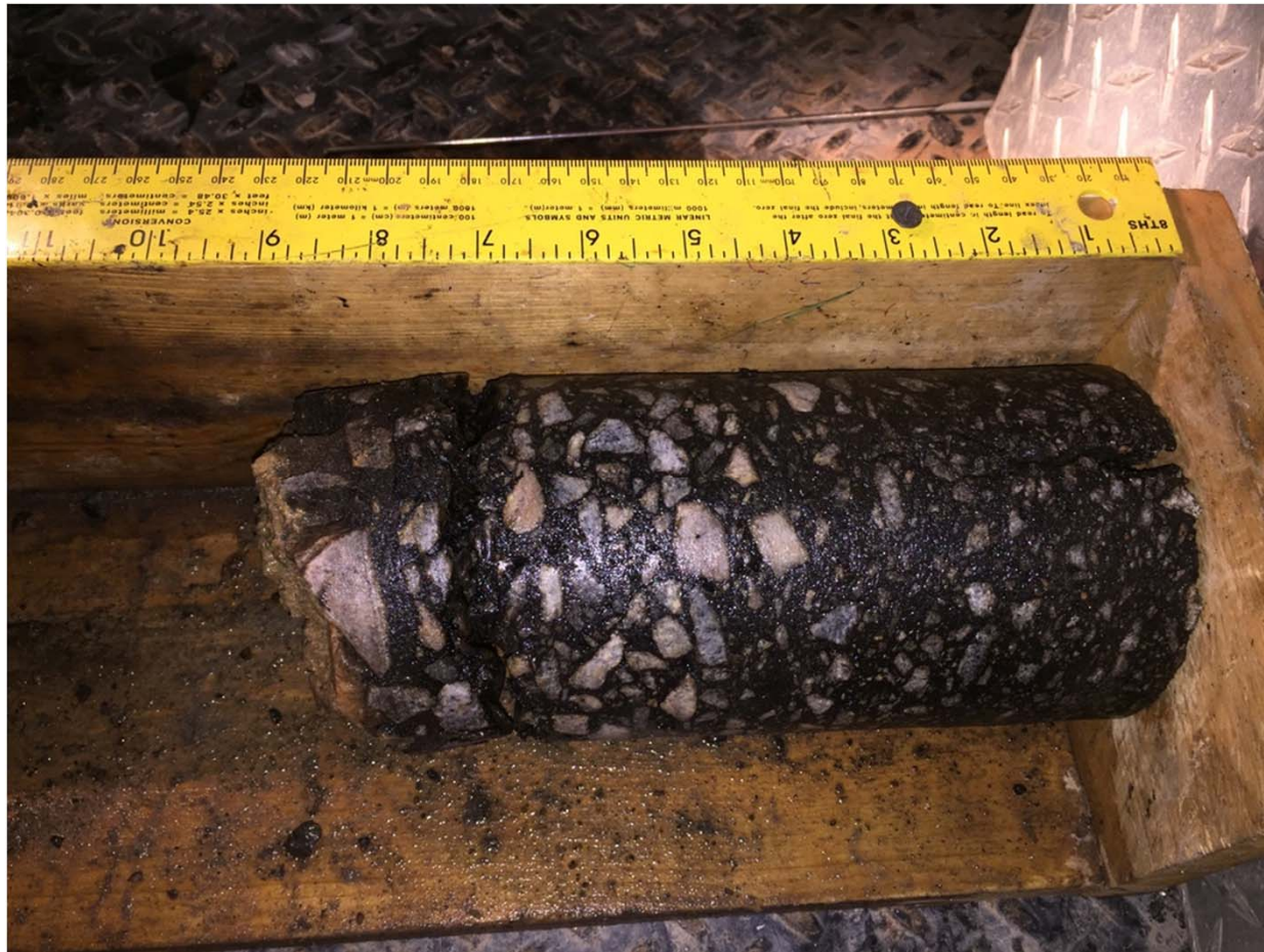
I-26 MM 88.0 westbound inside lane (b)
