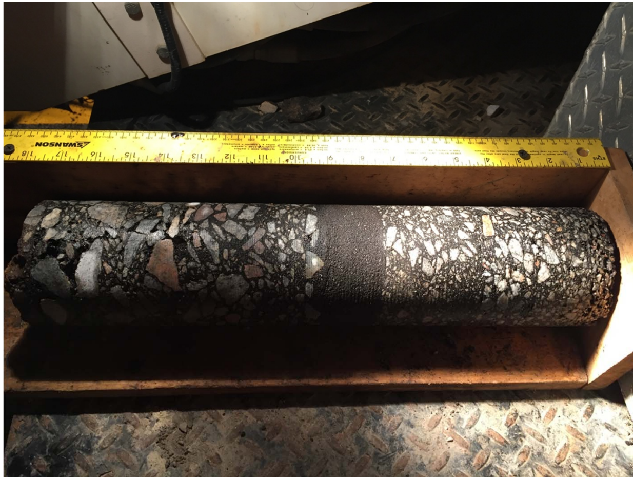
I-26 MM 94.0 westbound inside lane
