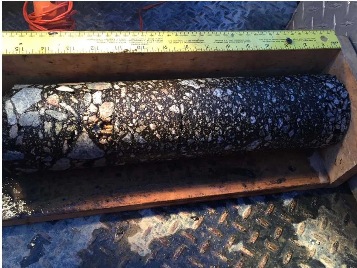
I-26 MM 97.0 westbound outside lane
