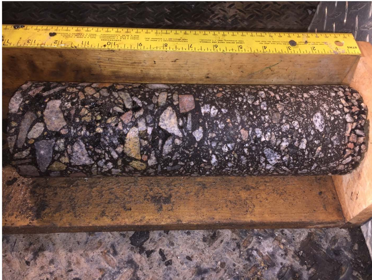
I-26 MM 99.5 westbound inside lane
