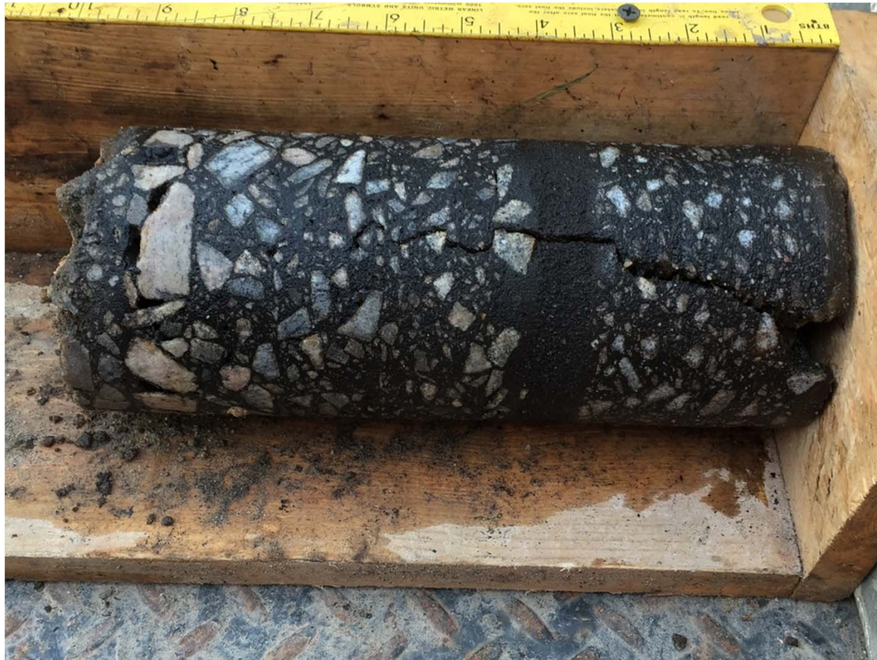
I-26 MM 89.0 eastbound inside lane
