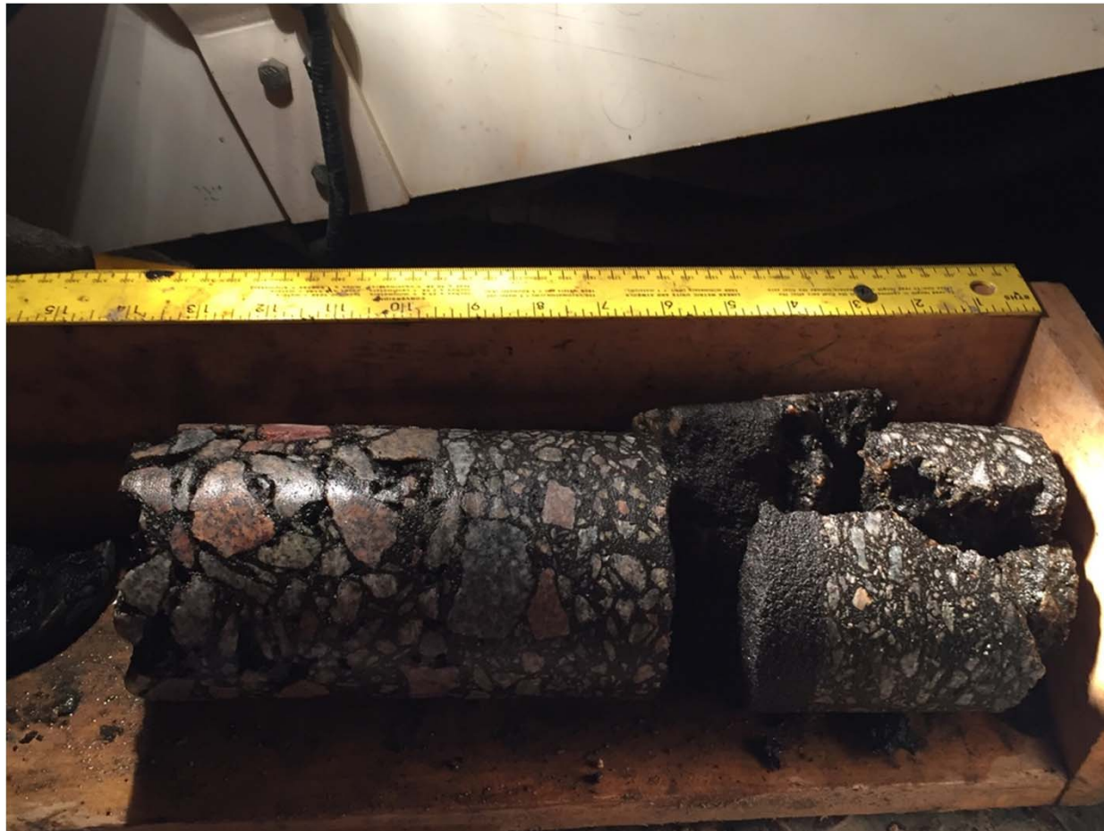
I-26 MM 98.0 eastbound inside lane
