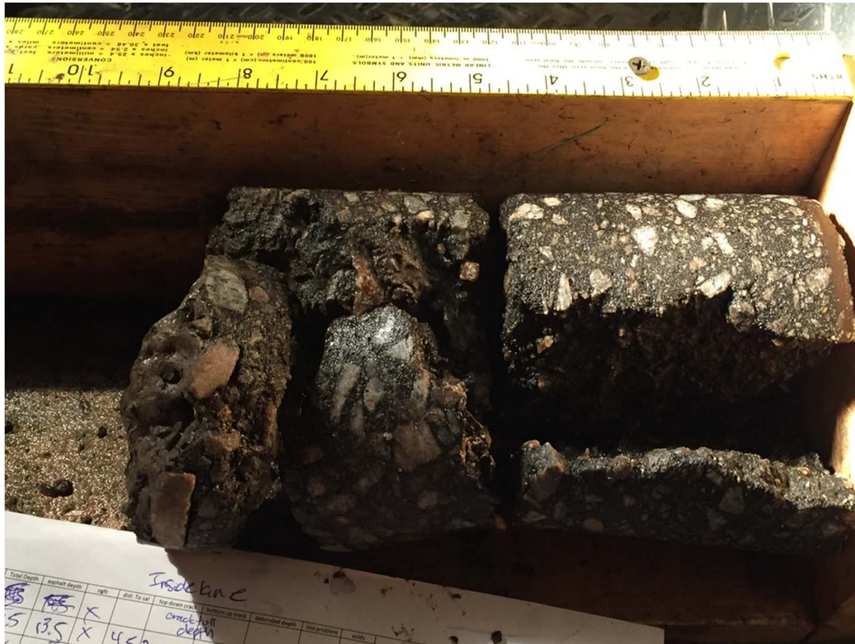
I-26 MM 86.0 westbound inside lane
