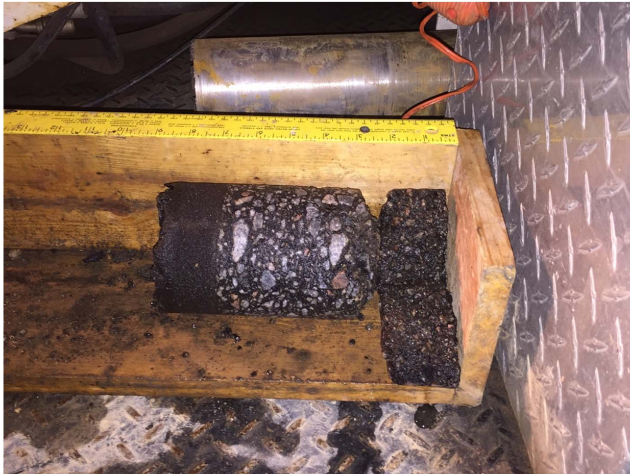
I-26 MM 94.5 westbound outside lane
