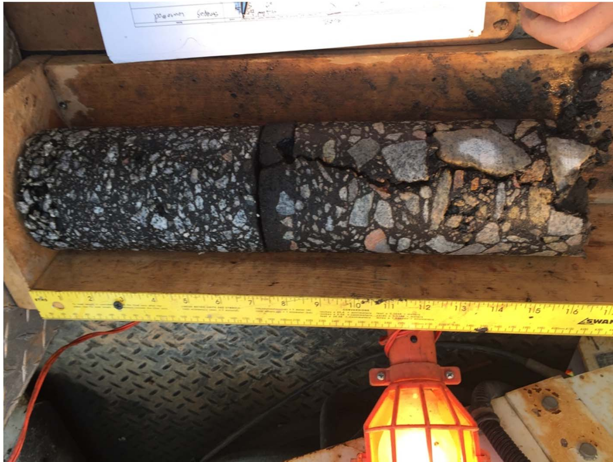
I-26 MM 98.0 westbound outside lane
