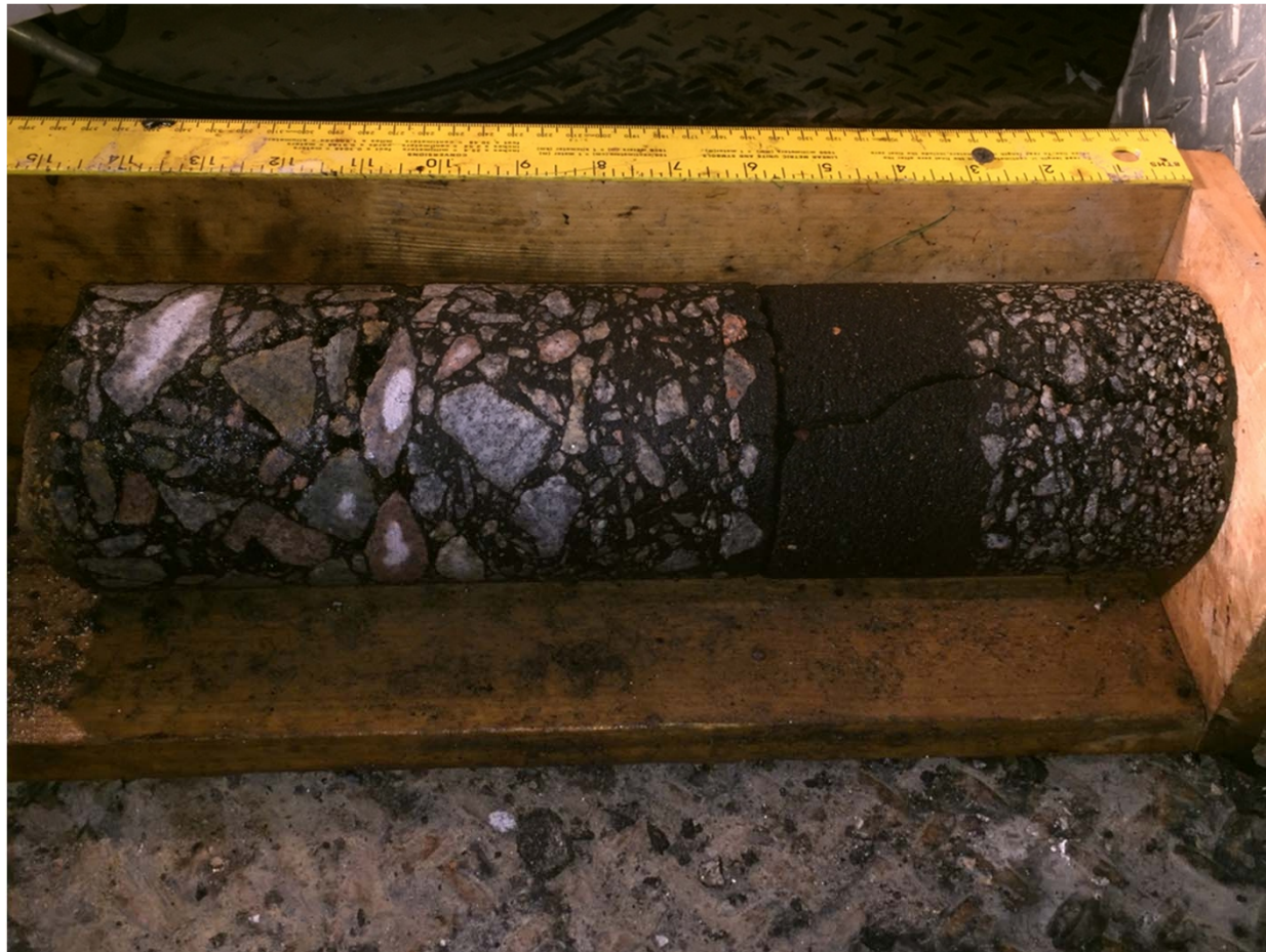
I-26 MM 96.5 westbound inside lane
