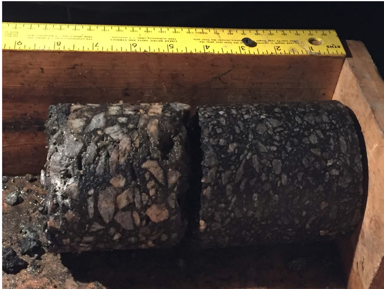
I-26 MM 86.5 - westbound outside lane
