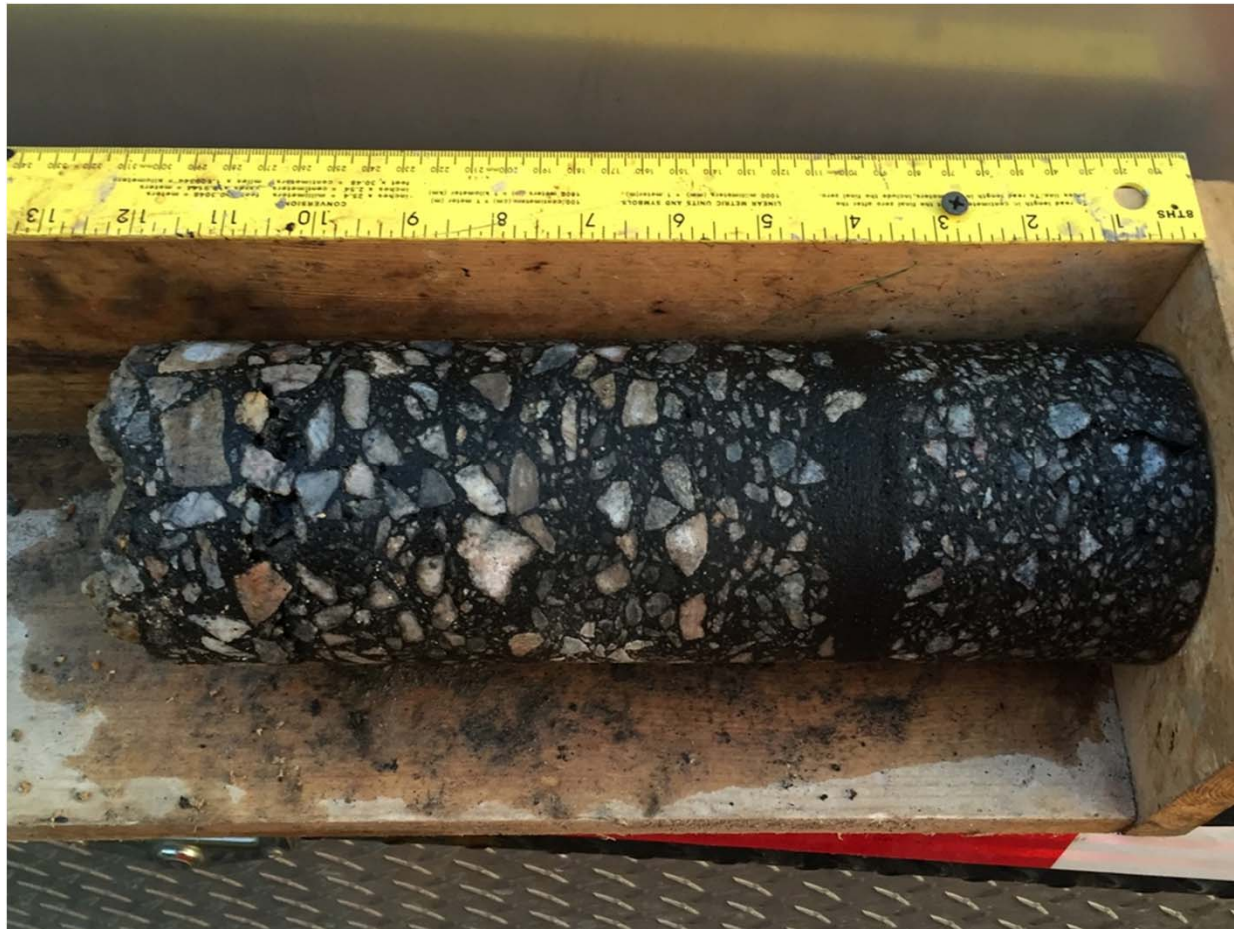
I-26 MM 91.0 eastbound inside lane (b)
