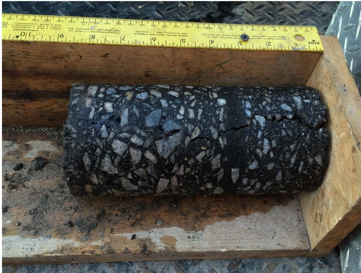
I-26 MM 87.0 eastbound inside lane
