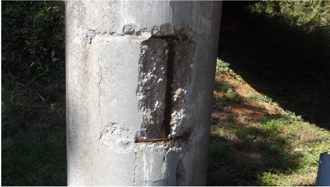
Figure 11 - Spall on Column
