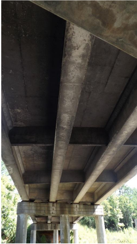
Figure 6 – Superstructure (from underneath) and Collision Damage to Bottom of Beam
