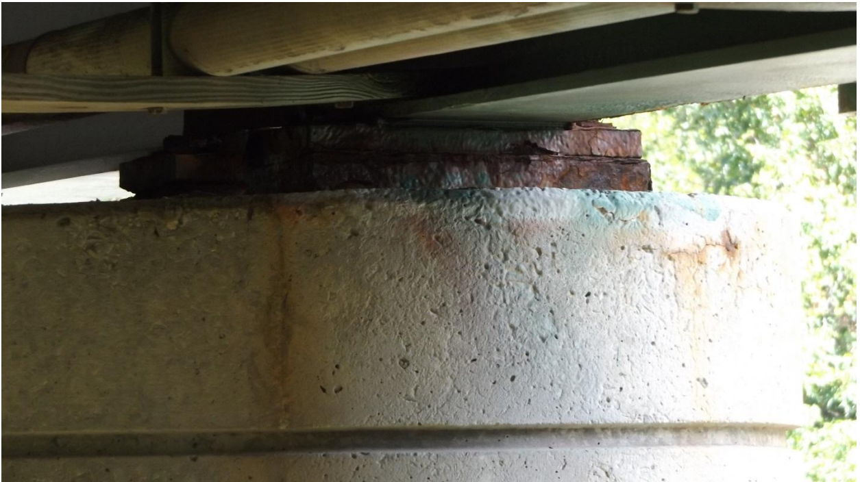
Figure 8 – Interior Bent Bearing
