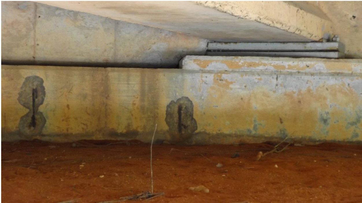
Figure 12 - End Bent Spalling
