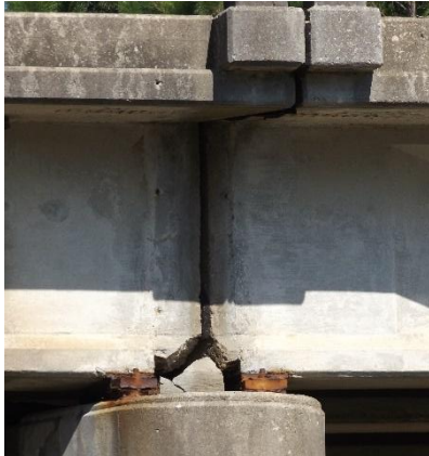
Figure 4 – Portion of Beam cracked off
