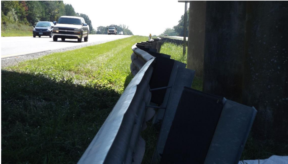
Figure 13 – Guardrail Damage
