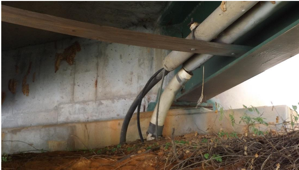
Figure 13 – Utilities going underground near End Bent
