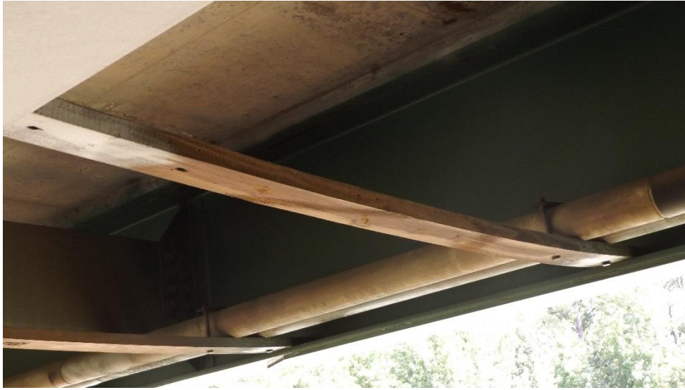
Figure 14 – Wooden Slats supporting Conduit
