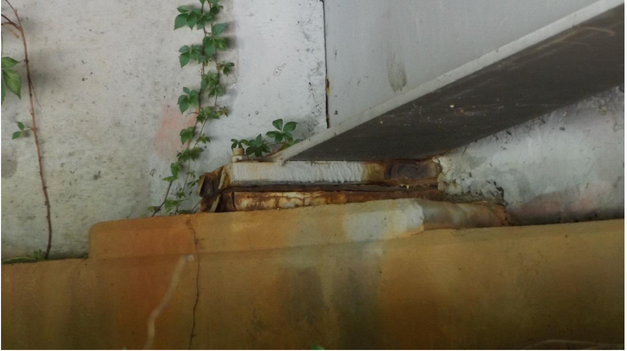
Figure 7 – End Bent Bearing
