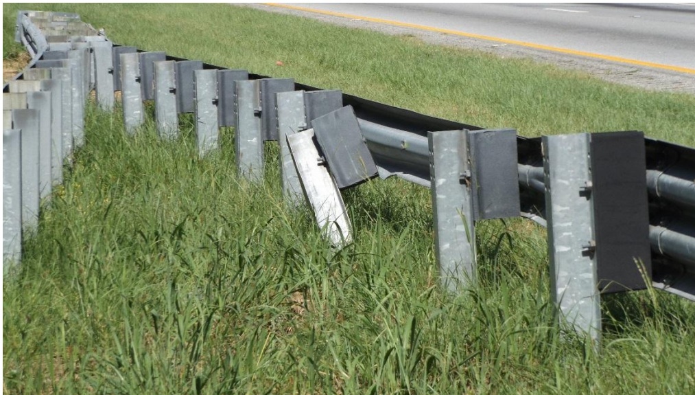
Figure 14 – Guardrail Damage
