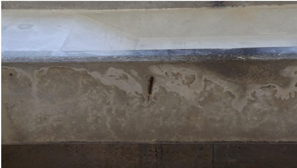
Figure 5 – Exposed Rebar in Beam
