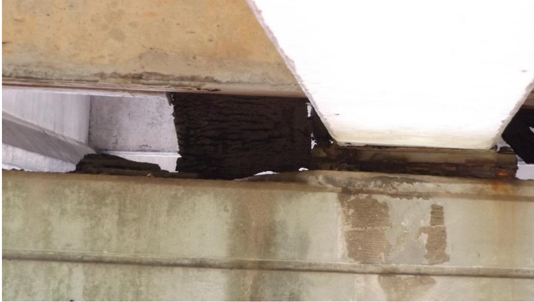
Figure 7 - Bearing Corrosion and Expansion Joint material falling through joint opening
