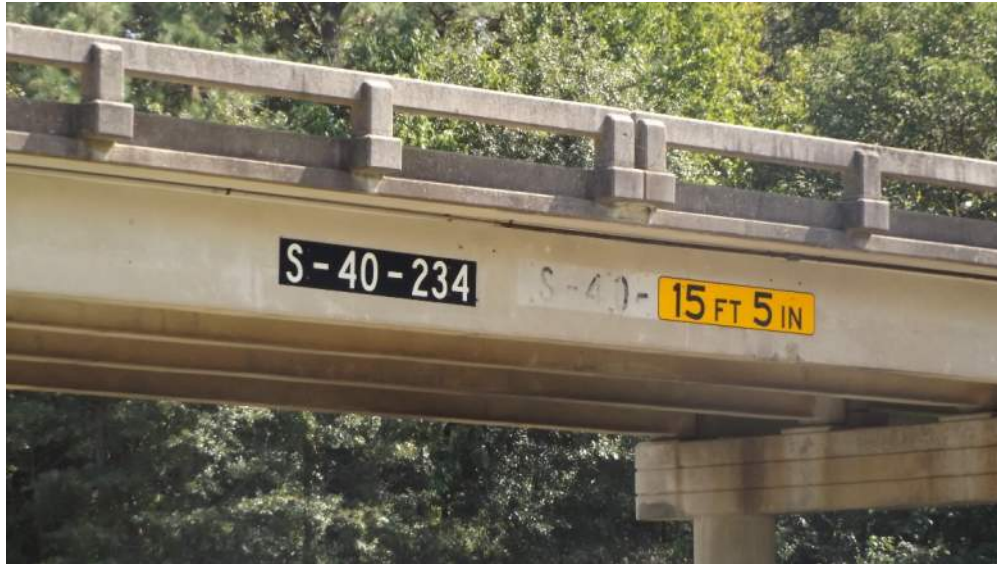
Figure 10 - Vertical Clearance (I-26 EB)
