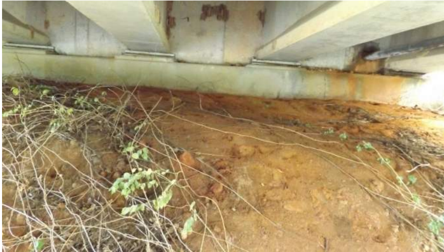
Figure 6 – End Bent Bearings
