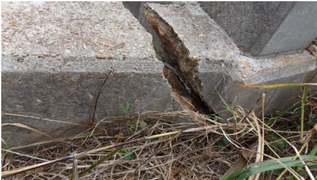
Figure 13 – Crack in Wing Wall
