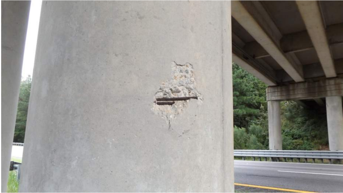
Figure 12 – Spall in Column
