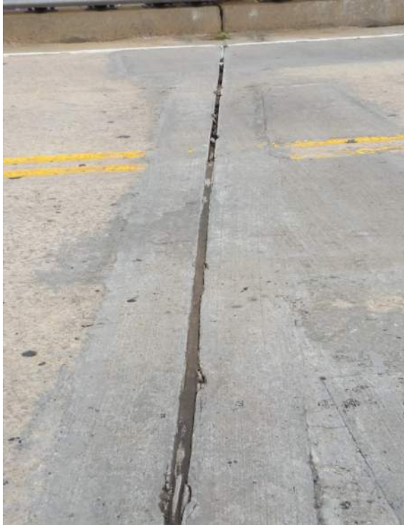
Figure 8 – Expansion Joint
