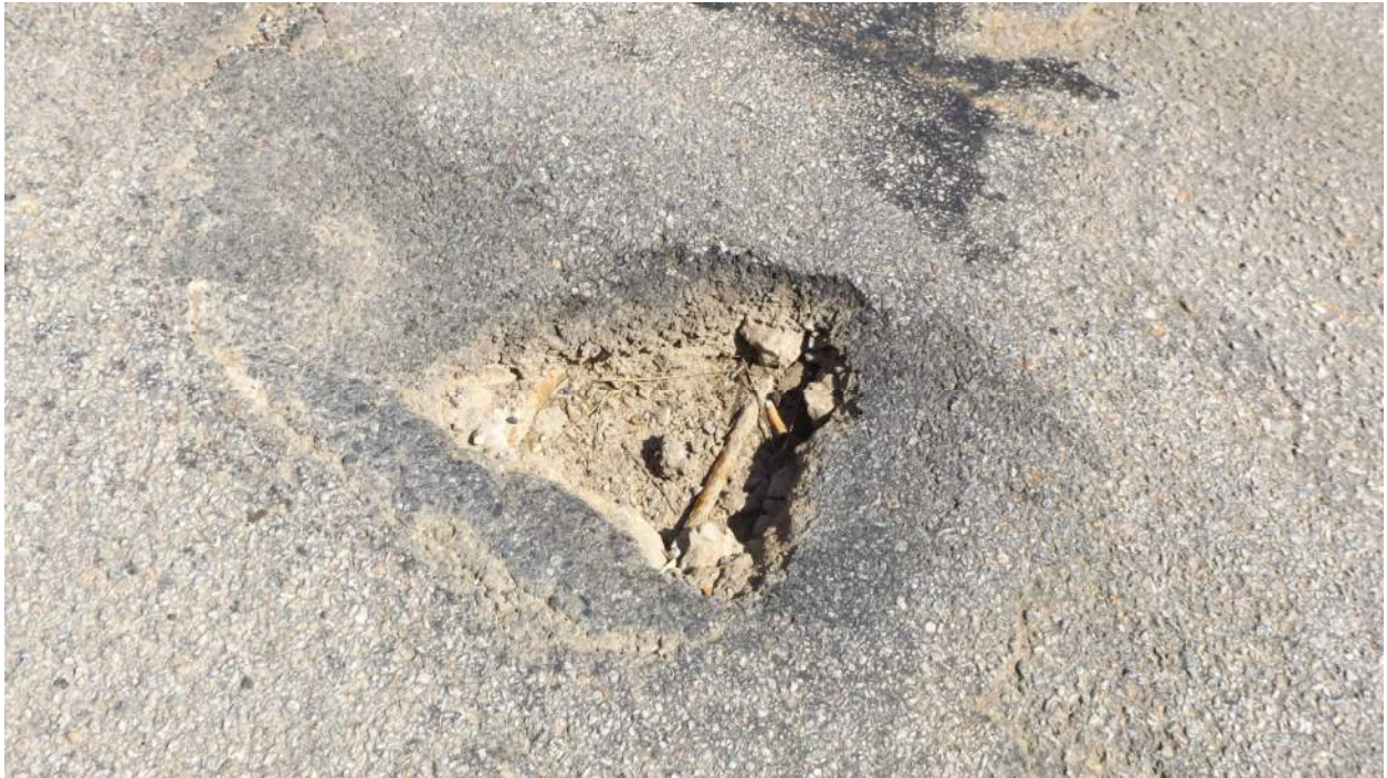
Figure 5 – Exposed Rebar in Concrete Deck
