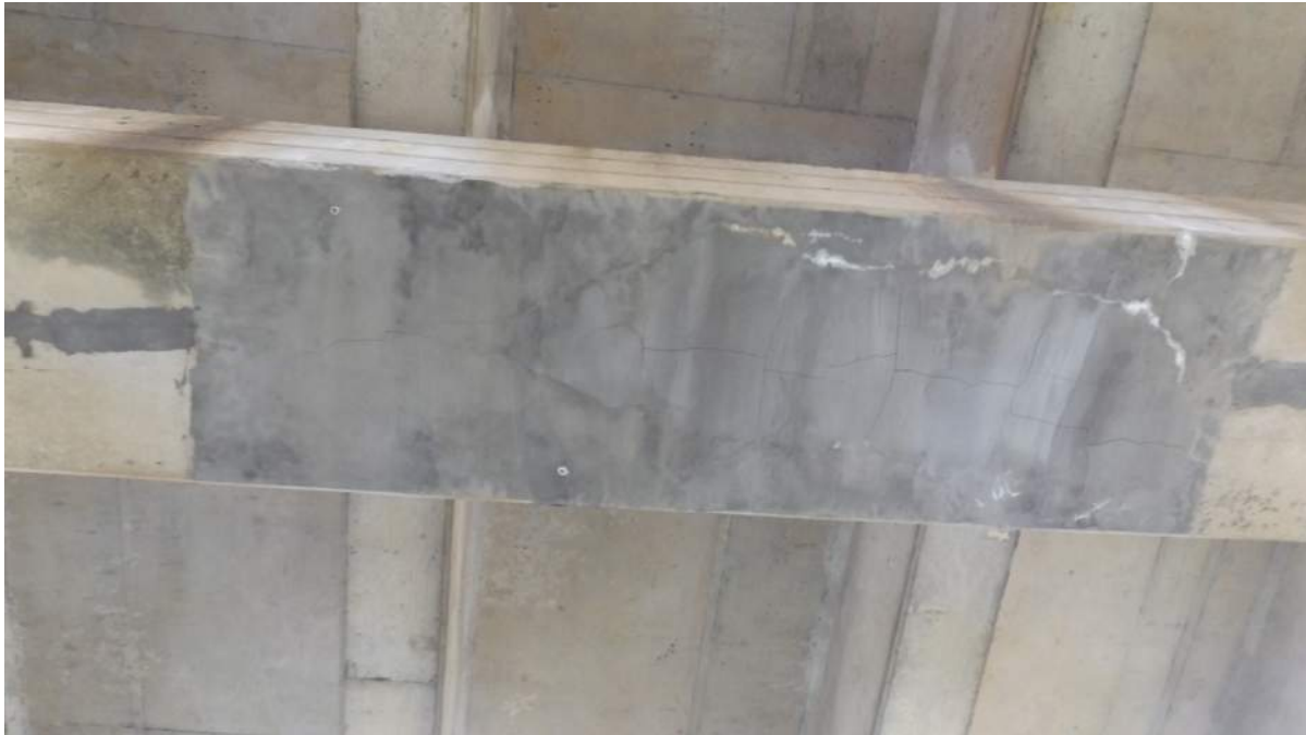
Figure 8 – Repaired Area in Cap
