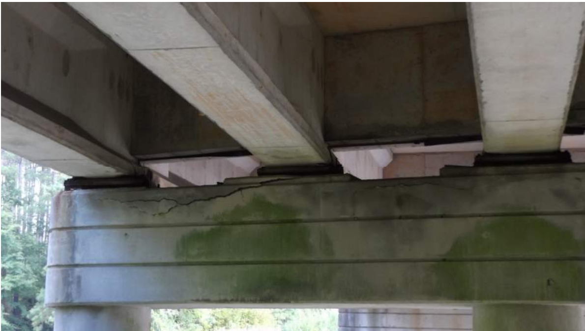
Figure 11 – Horizontal Crack in Bent Cap
