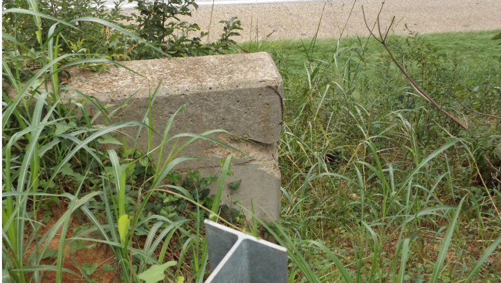
Figure 11 – End Bent Wing Wall
