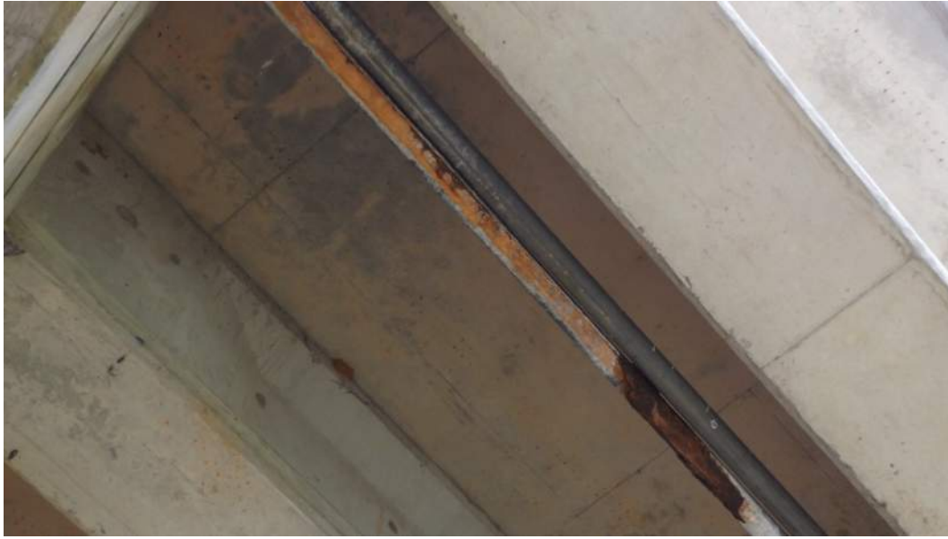
Figure 14 – Conduit Corrosion
