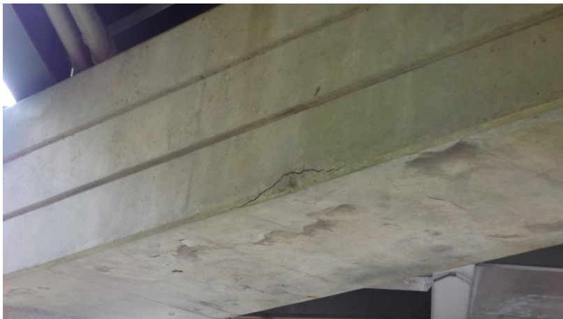
Figure 10 – Crack in Interior Bent Cap
