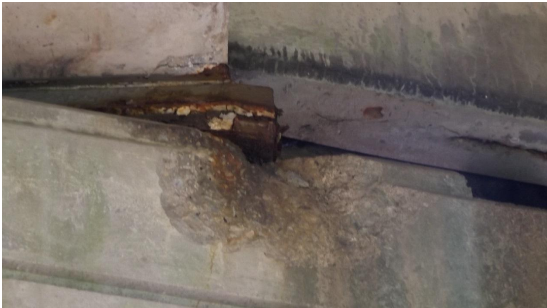
Figure 10 - Spall on Top of Pier Cap
