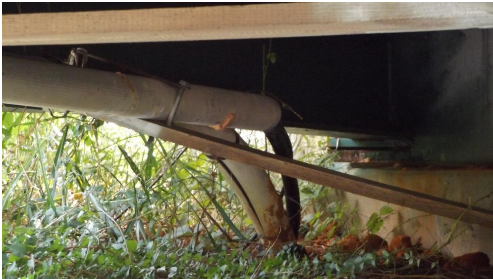
Figure 15 – Wooden Slat has fallen off the Beam
