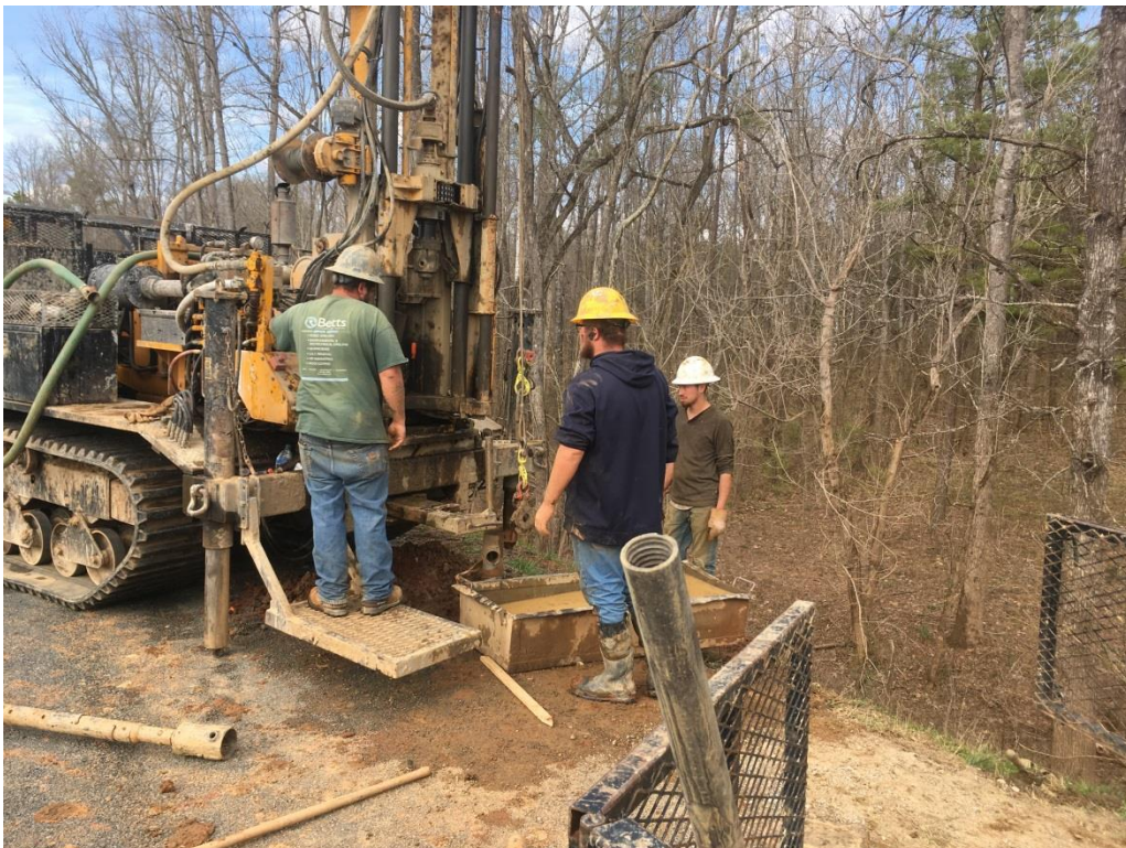
Photo 4: Drill Rig at Boring B-7
