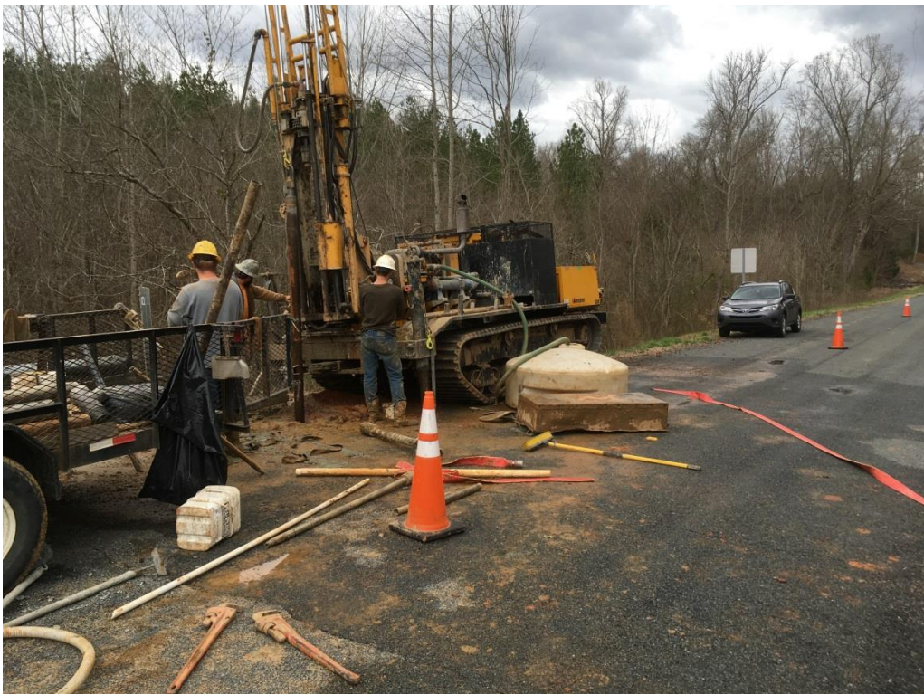
Photo 2: Drill Rig at Boring B-6
