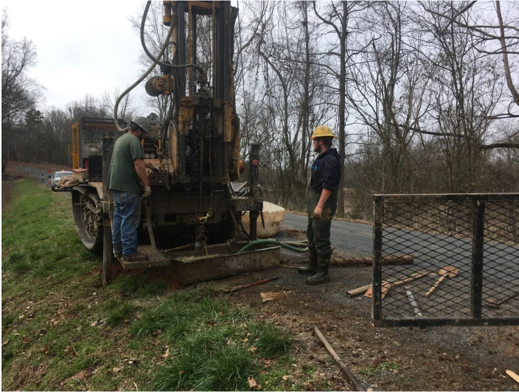
Photo 1: Drill Rig at Boring B-5
