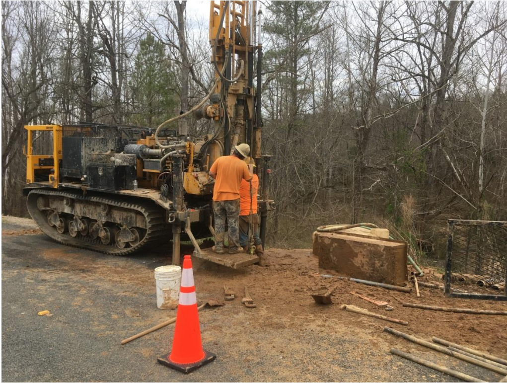
Photo 3: Drill Rig at Boring B-7
