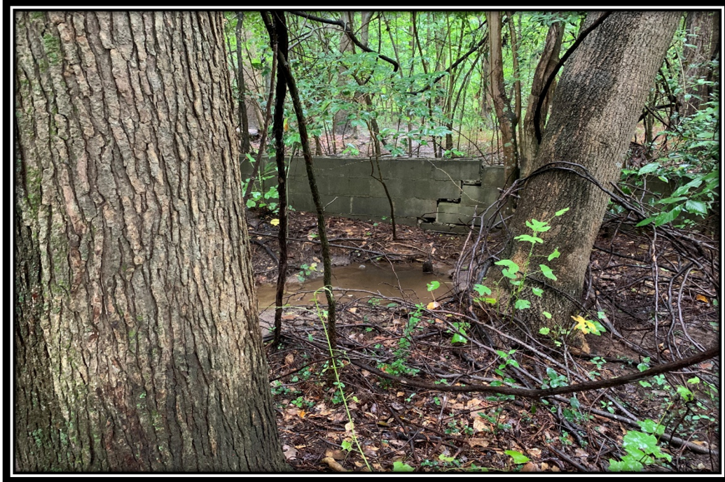
View of Parcel 270, facing west
