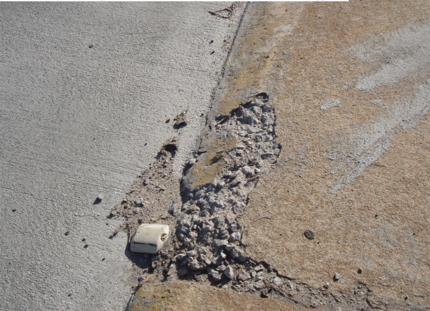
27 Feb 2019: Minor spalls in raised median between lanes on S-31, typical.
