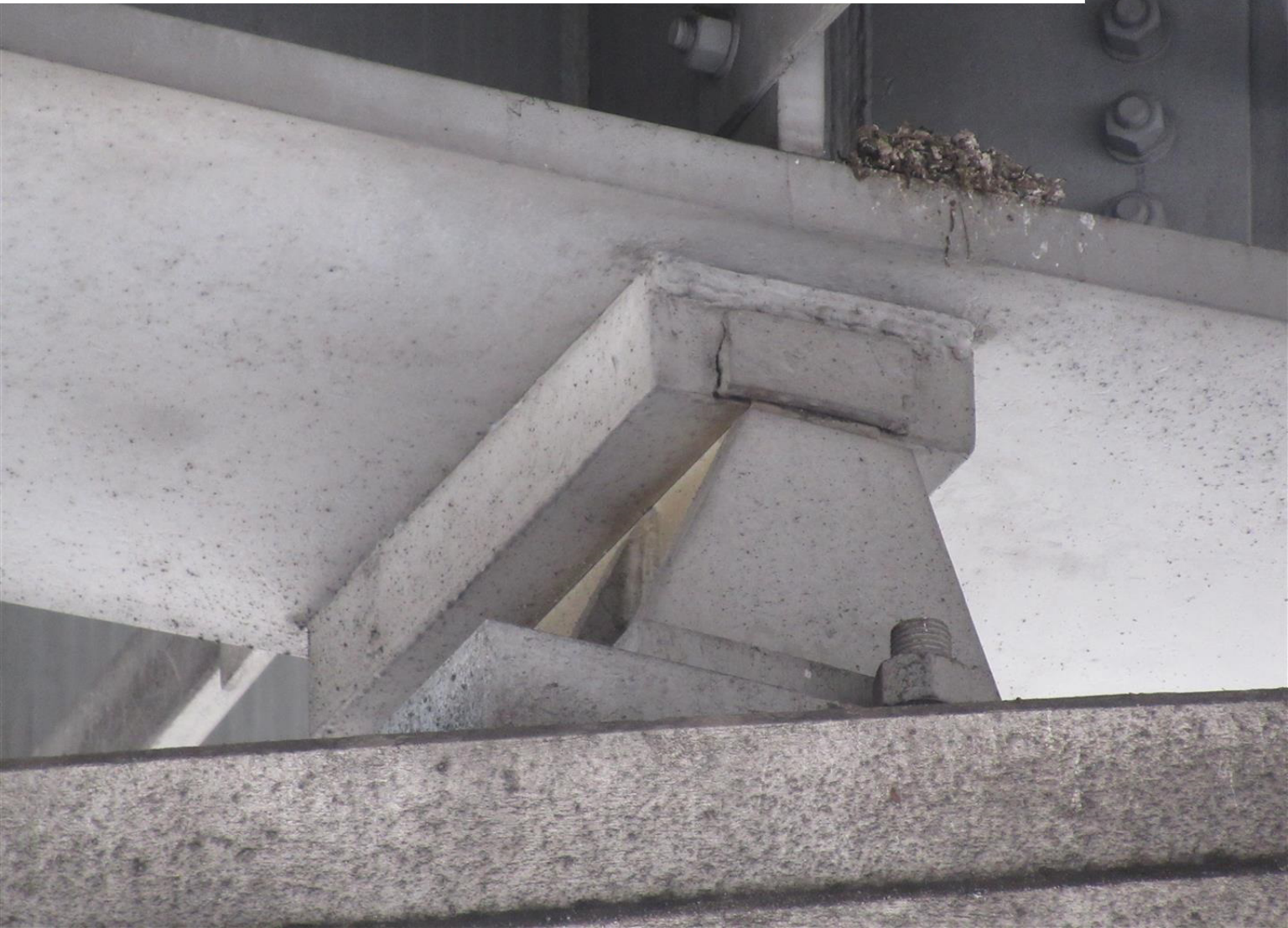
27 Feb 2019: Bearing at beam 9, bent 4 sole plate has broken welds, left side.
