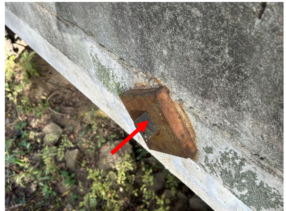
Photo 4. LBP on Orange Tie Rod Washer.
