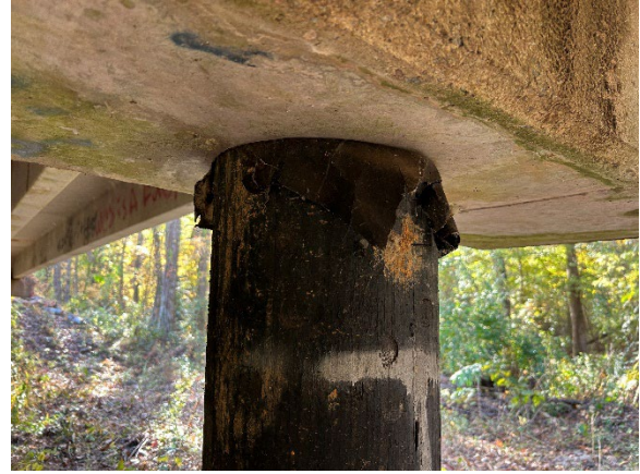
Photo 2. Non-ACM Timber Pile Cap Felt.
