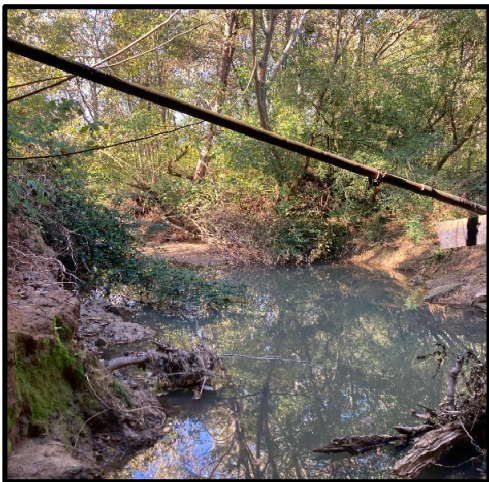
Steel Utility Conduit Adjacent South Side of Bridge
