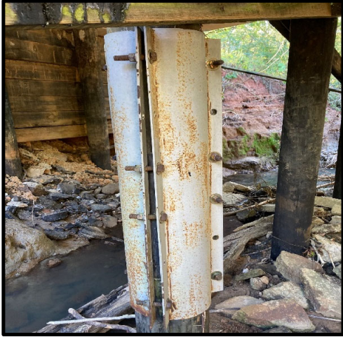
Timber Pile Support Brace
