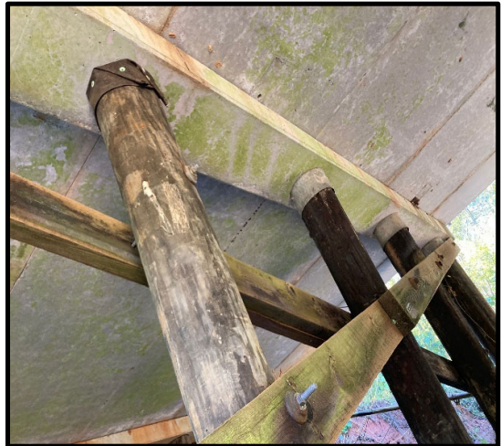
Timber Pile Foundation
