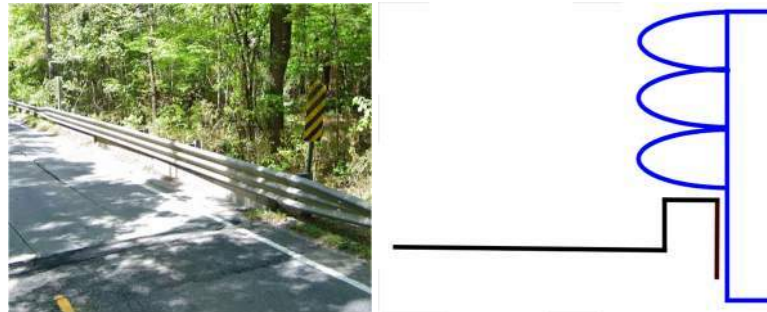
Figure 5.3.1.5 Hidden/Overhung Curb
