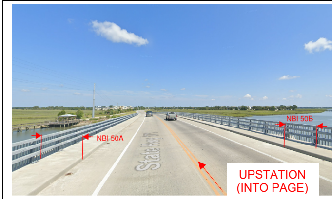
Figure 7.3.15-5 Bridge Without Curb or Sidewalk (Asset ID 2301)
