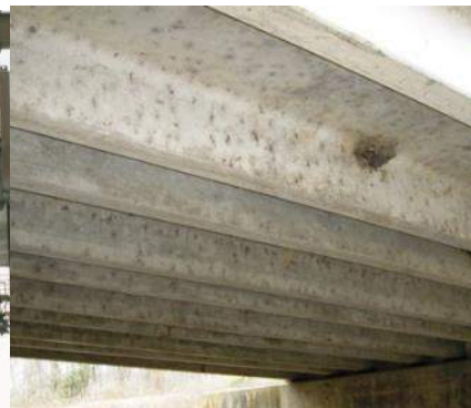
109 Prestressed Concrete Open Girder (Precast Double T)
