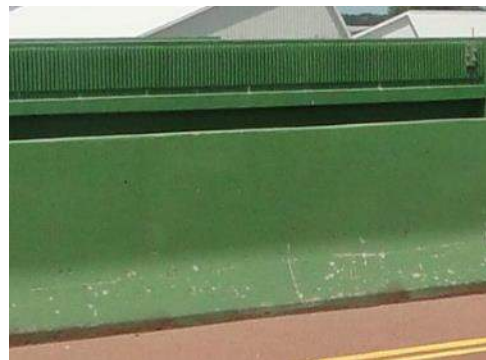
521 Concrete Protective Coating
