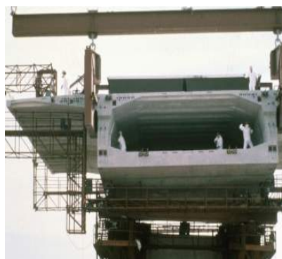
104 Prestressed Closed Web/Box Girder (Segmental)
