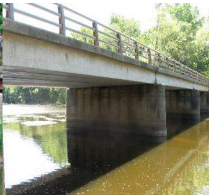
210 Reinforced Concrete Pier Wall
