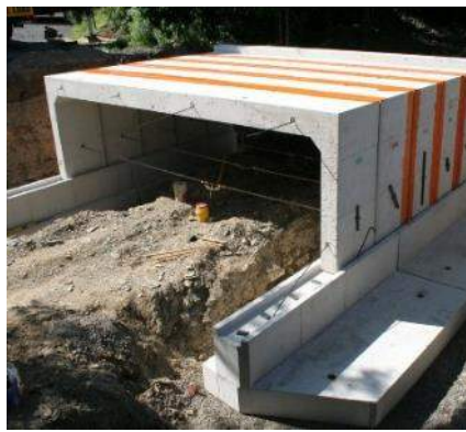
3-Sided Concrete Box Culvert
