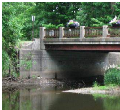
215 Reinforced Concrete Abutment
