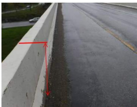
Figure 5.3.1.9.1.2-2 Reveal Measurement at Barrier
