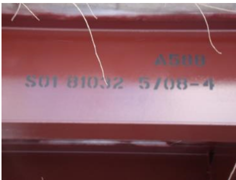
515 Steel Protective Coating
