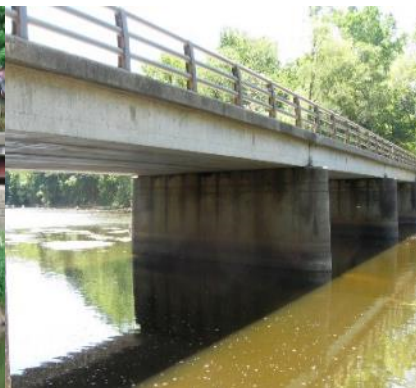
210 Reinforced Concrete Pier Wall
