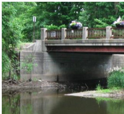
215 Reinforced Concrete Abutment
