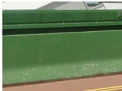
521 Concrete Protective Coating
