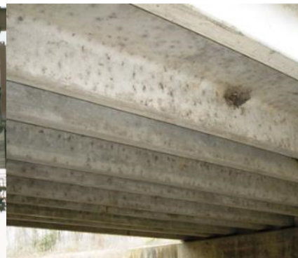
109 Prestressed Concrete Open Girder (Precast Double T)
