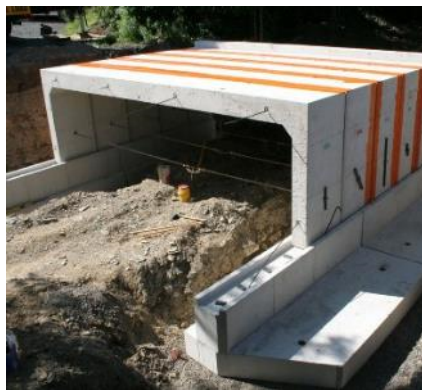
3-Sided Concrete Box Culvert
