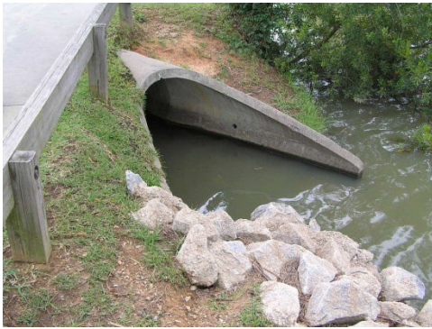
Use Pipe Flared End Section when specified in the plans or special provisions.
