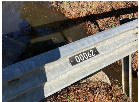
Photo 6. SCDOT Bridge Asset # Attached to Galvanized Metal Guardrail.
