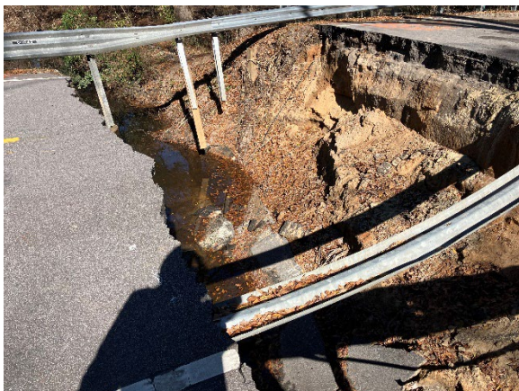
Photo 5. Eastern Side Wash Out of the Bridge.
