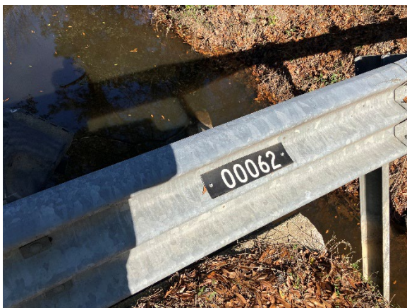
Photo 5. Bridge Asset # Attached to Galvanized Metal Guardrail.
