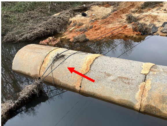
Photo 3. Exposed Utility Lines on the Southern Side of Bridge.
