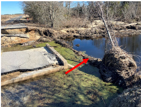
Photo 3. Exposed Utility Pipe on the Southern Side of Bridge.
