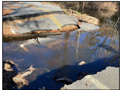
Photo 1: The washed-out portion of the former S-5-458 Bridge over Indian Camp Branch in Bamberg County, South Carolina.
