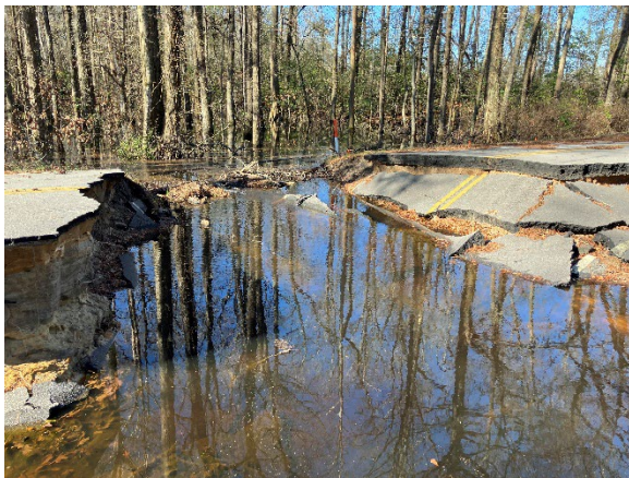
Photo 3. View of Road and Bridge Washout Looking Eastward.
