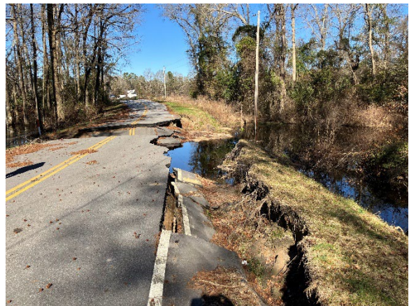
Photo 4. View of Bridge Washout and Roadway Embankment Washout Along Southeast Side of Road and Bridge.
