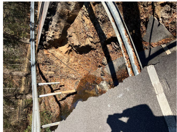
Photo 4. Eastern Side of Bridge Wash Out.
