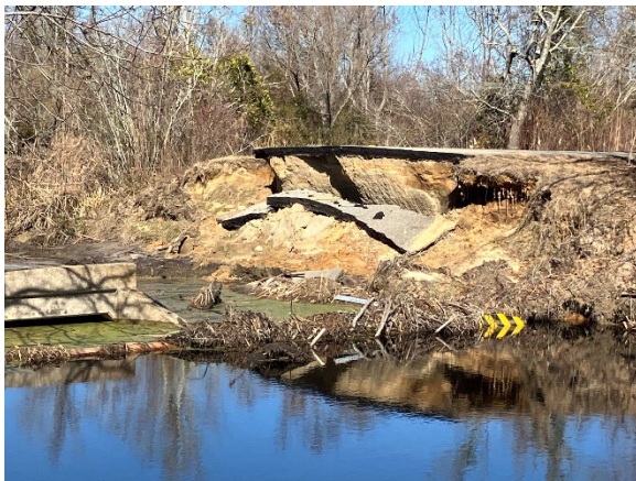
Photo 5. View of the Washout on the East Side of Bridge.
