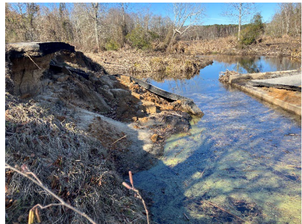
Photo 6. View of Washout on the West side of the Bridge.
