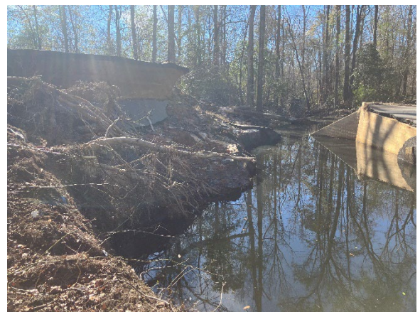
Photo 6. Northeastern View of Washout on the East side of the Bridge.
