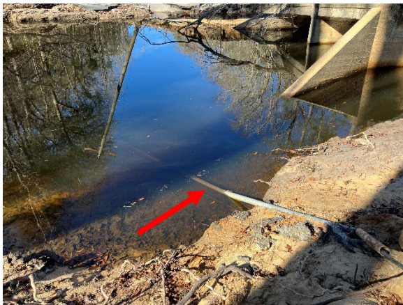
Photo 3. Exposed Utility Line on the Southern Side of the Bridge.
