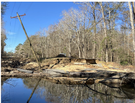
Photo 5. Southeastern View of the Washout on the West Side of the Bridge and the Leaning Power Pole.
