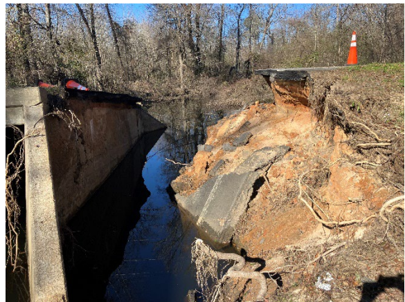
Photo 6. View of the Washout on the Southeastern Side of the Bridge.
