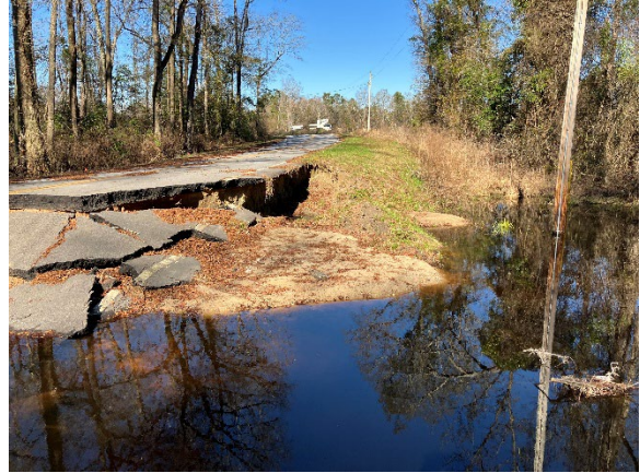
Photo 2. Northern View of Washed-Out Bridge.
