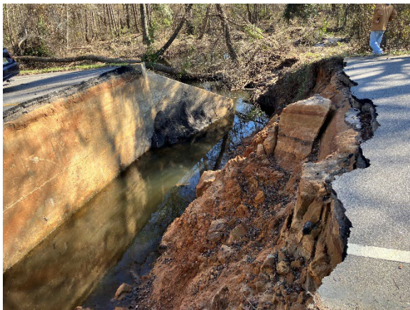
Photo 5. View of the Washout on the Northwestern Side of the Bridge.
