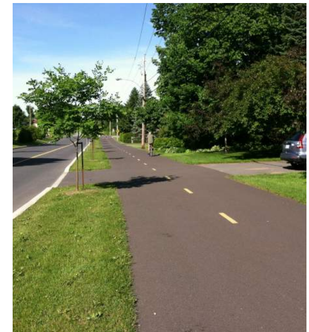
▲ Diagram cross section and plan view (left) and a sidepath in Granby, Quebec (right)
