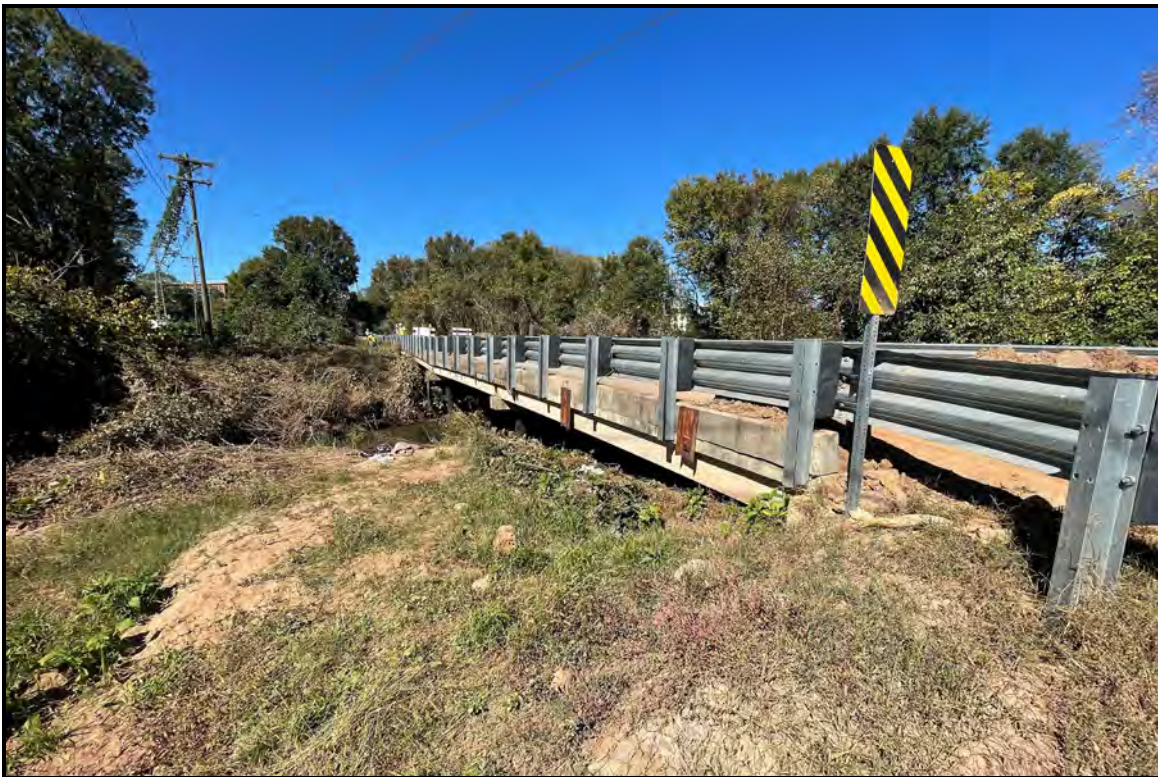
Figure 6. View of Project Area, looking north toward the bridge
