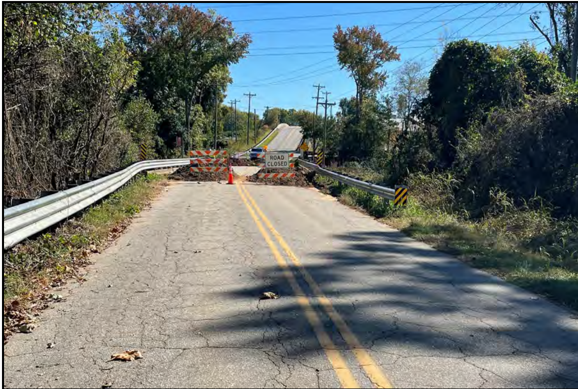
Figure 3. View of Project Area, looking southeast toward the bridge
