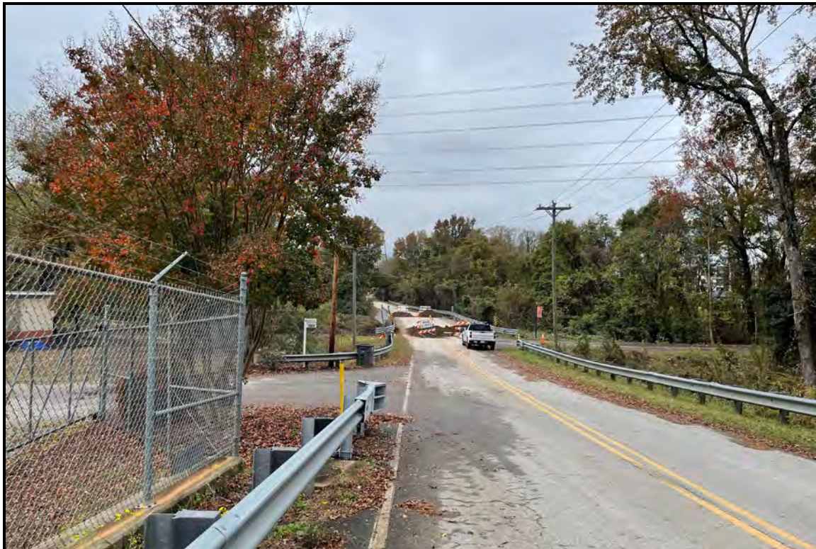
Figure 4. View of Project Area, looking northwest toward the bridge
