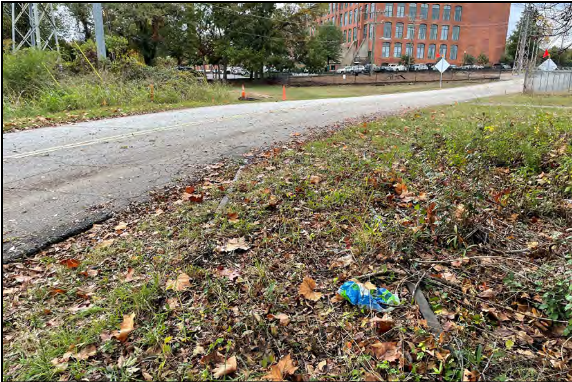
Figure 38. SHPO Site No. 6445, rail remnants on either side of S-147, looking northwest from Swamp Rabbit Trail toward Monaghan Mill
