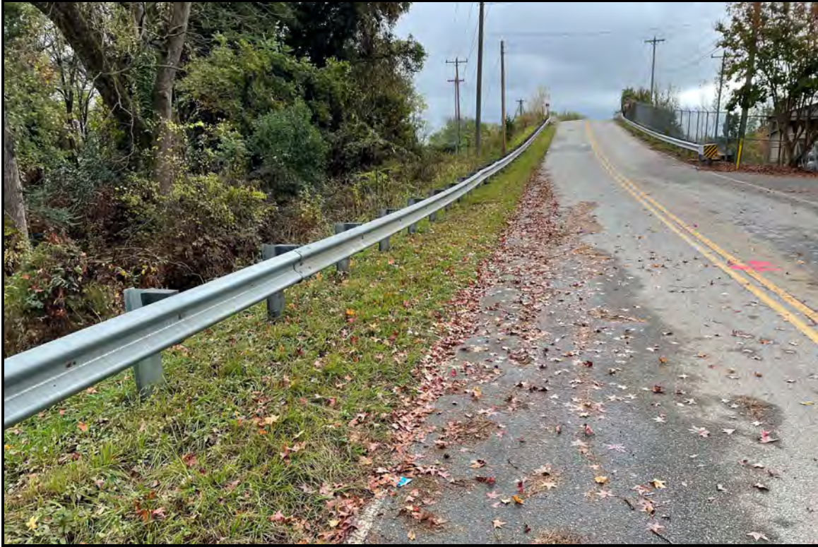
Figure 5. View of Project Area, looking southeast from bridge
