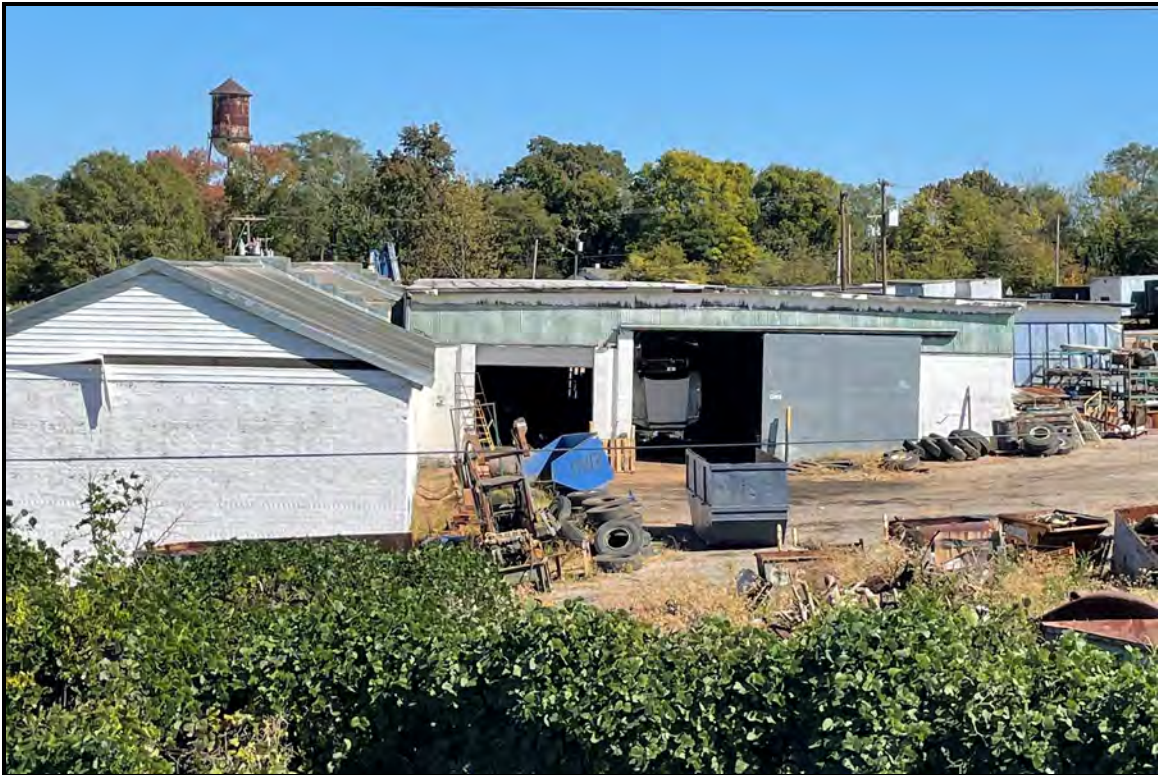
Figure 42. SHPO Site No. 6447, looking southwest
