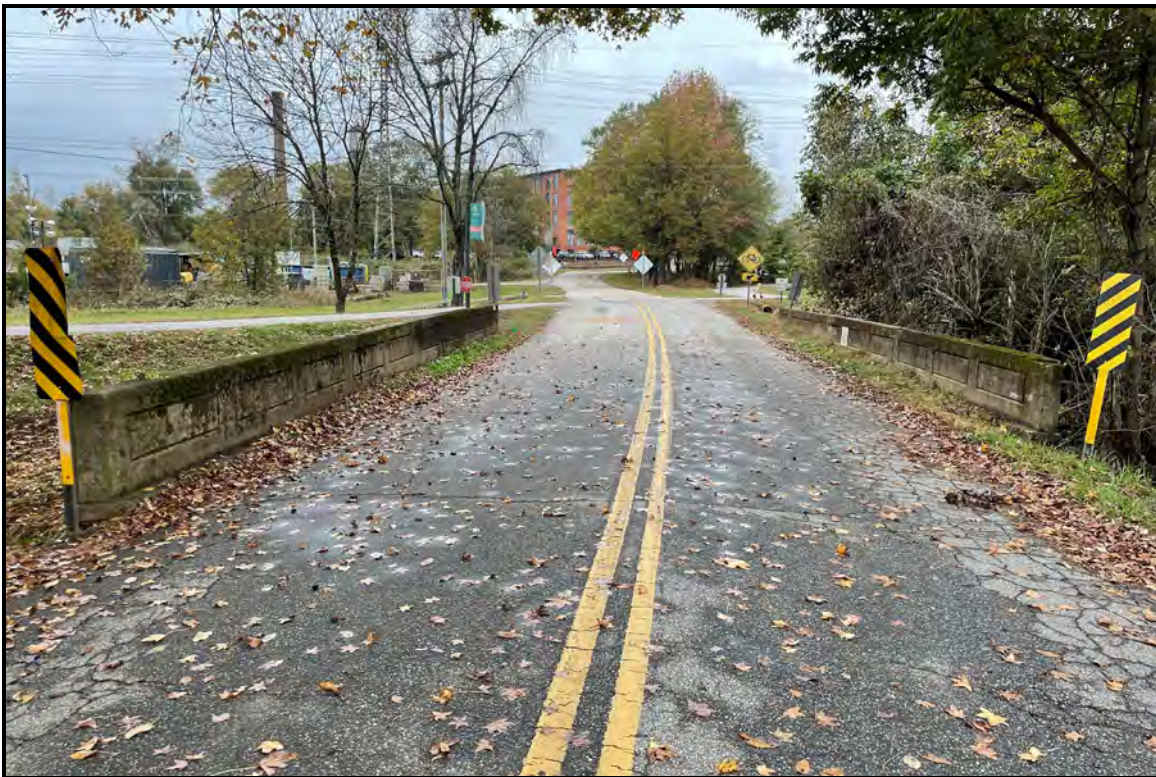
Figure 32. SHPO Site No. 6444, looking northwest
