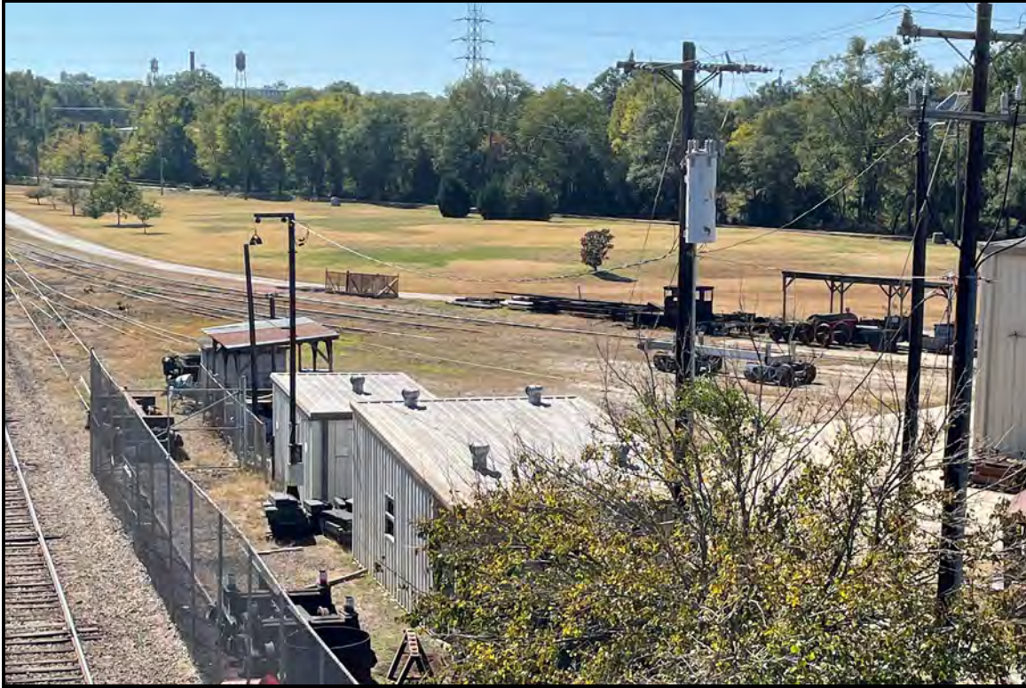
Figure 31. SHPO Site No. 1260.05, tracks connecting to CSX Railroad, looking southwest
