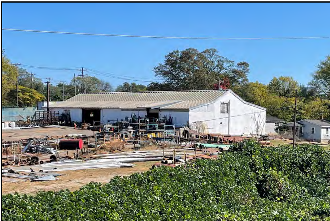
Figure 44. SHPO Site No. 6447.01, looking southwest
