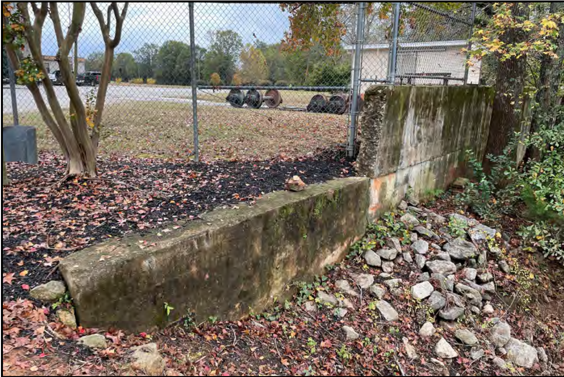
Figure 29. SHPO Site No. 1260.04, looking southwest
