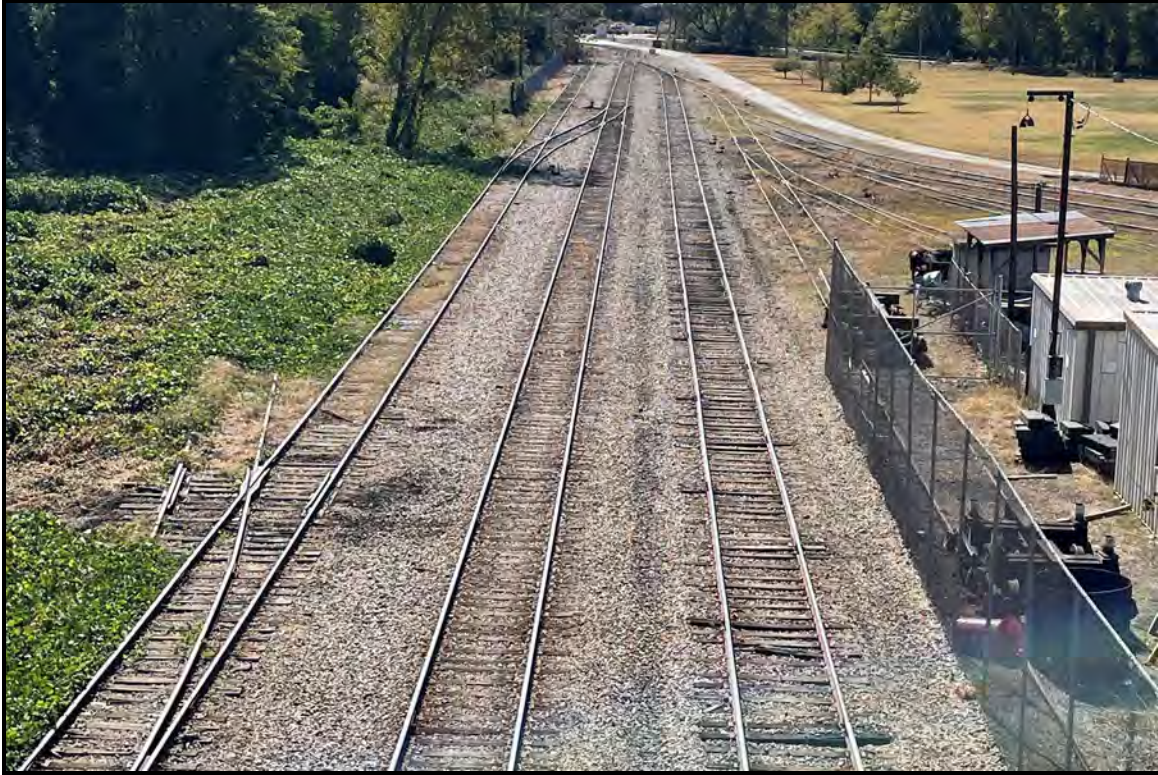
Figure 41. SHPO Site No. 6446, looking west from S-147 over CSX Railroad bridge
