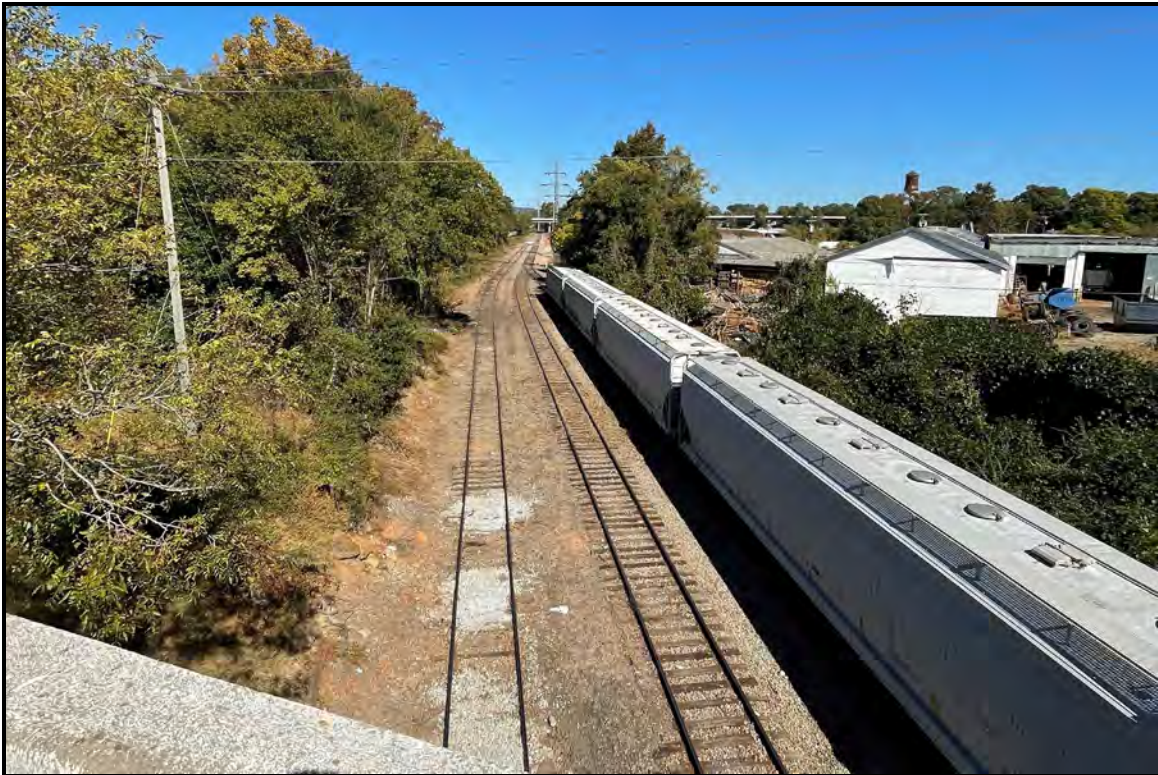
Figure 40. SHPO Site No. 6446, looking east from S-147 over CSX Railroad bridge
