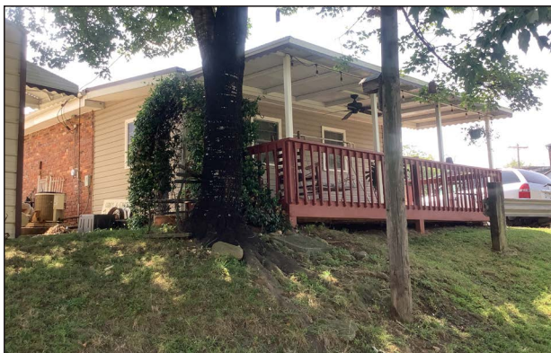
C. Rear Oblique, Looking Southwest
