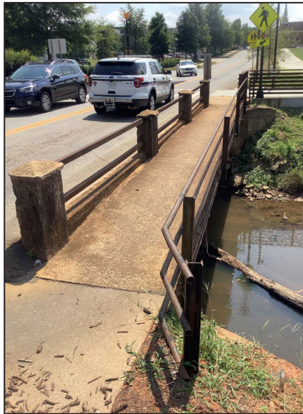
C. Original Concrete Columns and Metal Railings and Added Sidewalk on West Side
