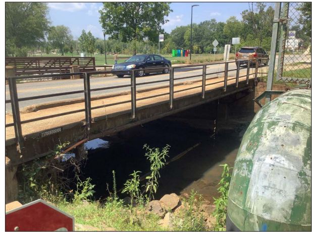
B. Looking Northwest
