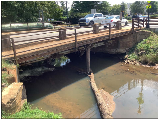
A. Looking Southeast
