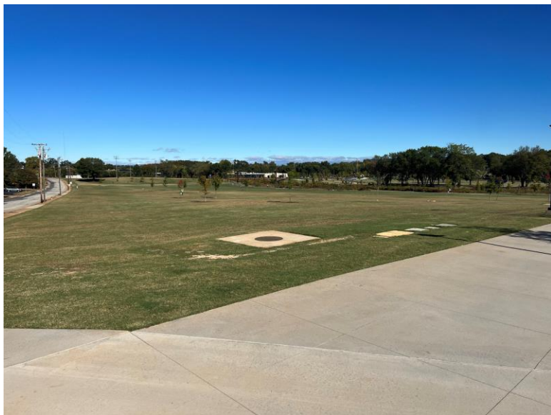
View of Parcels 3, 4, and 5, identified as City of Greenville Garage and Maintenance within EDR regulatory information, located at 348 and 360 S. Hudson Street within the Project Area. This UST/LUST site is considered CREC 2.
