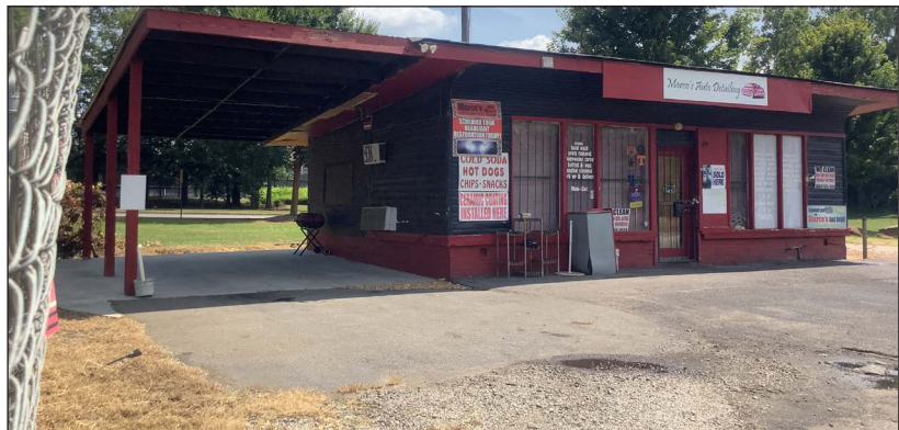
B. Oblique, Looking Southeast
