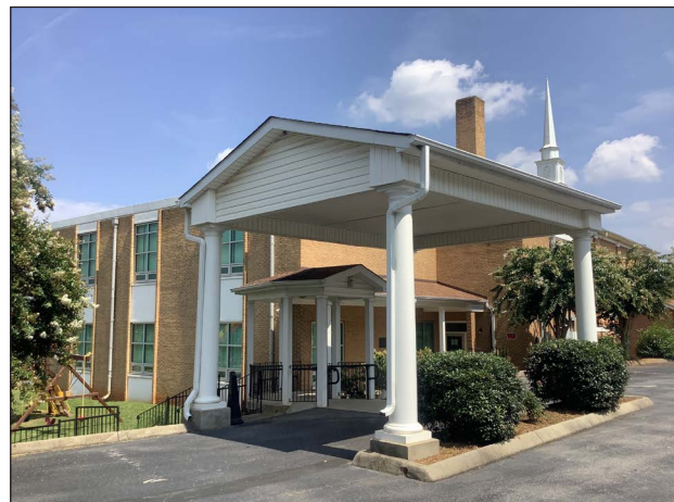
D. Rear Oblique, Looking Northeast
