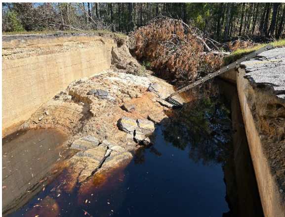
Photo 3. Washout Between the Culverts.
