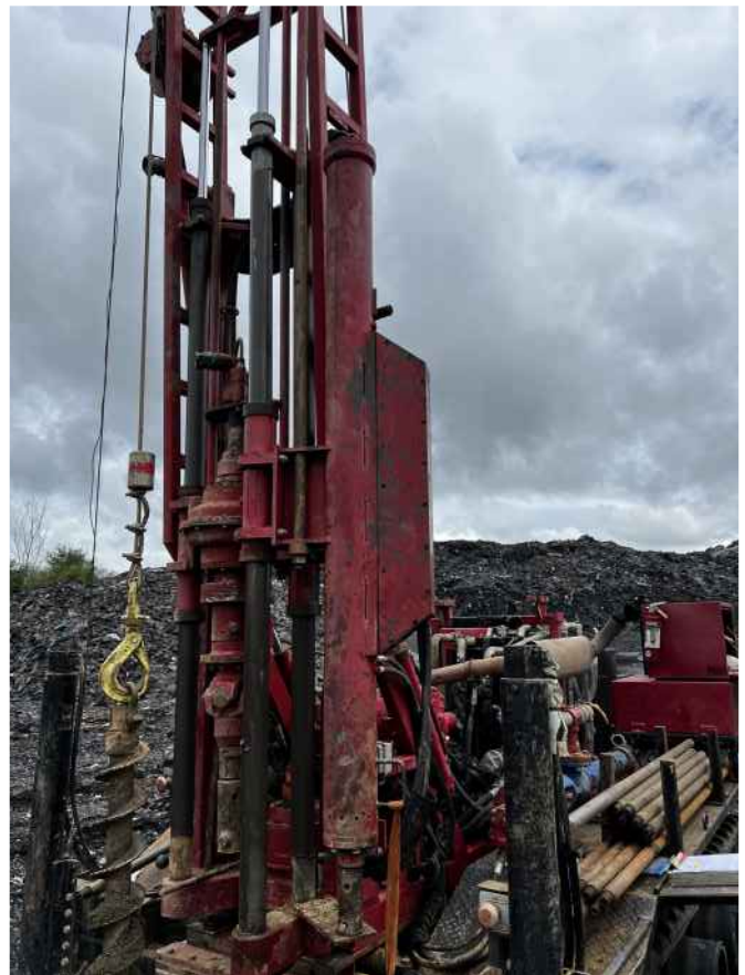
Figure No. 4: Automatic Hammer
