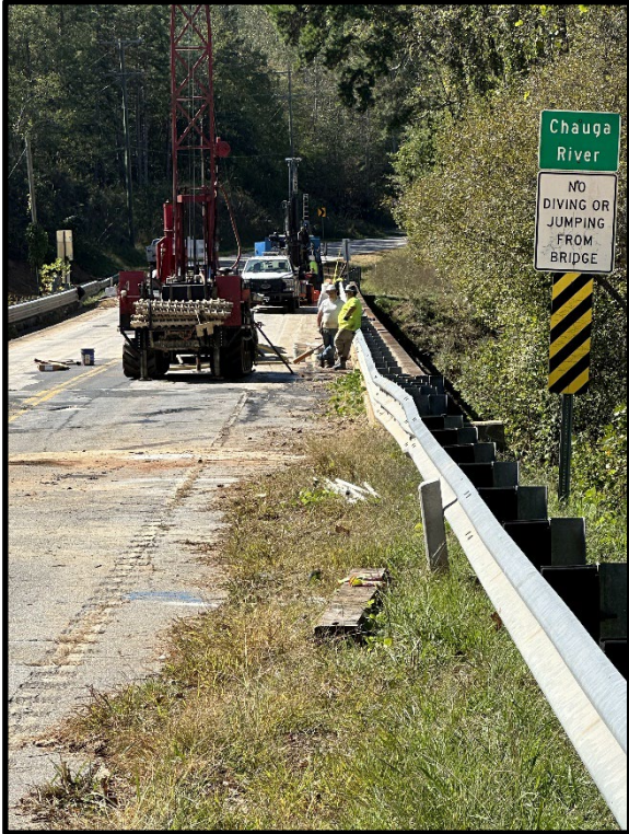
East Side of Bridge Facing West
