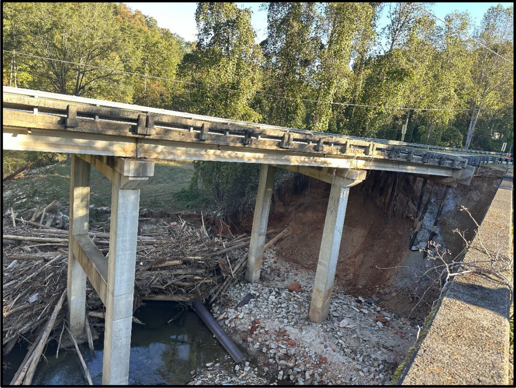
South Side of Bridge – Facing East
