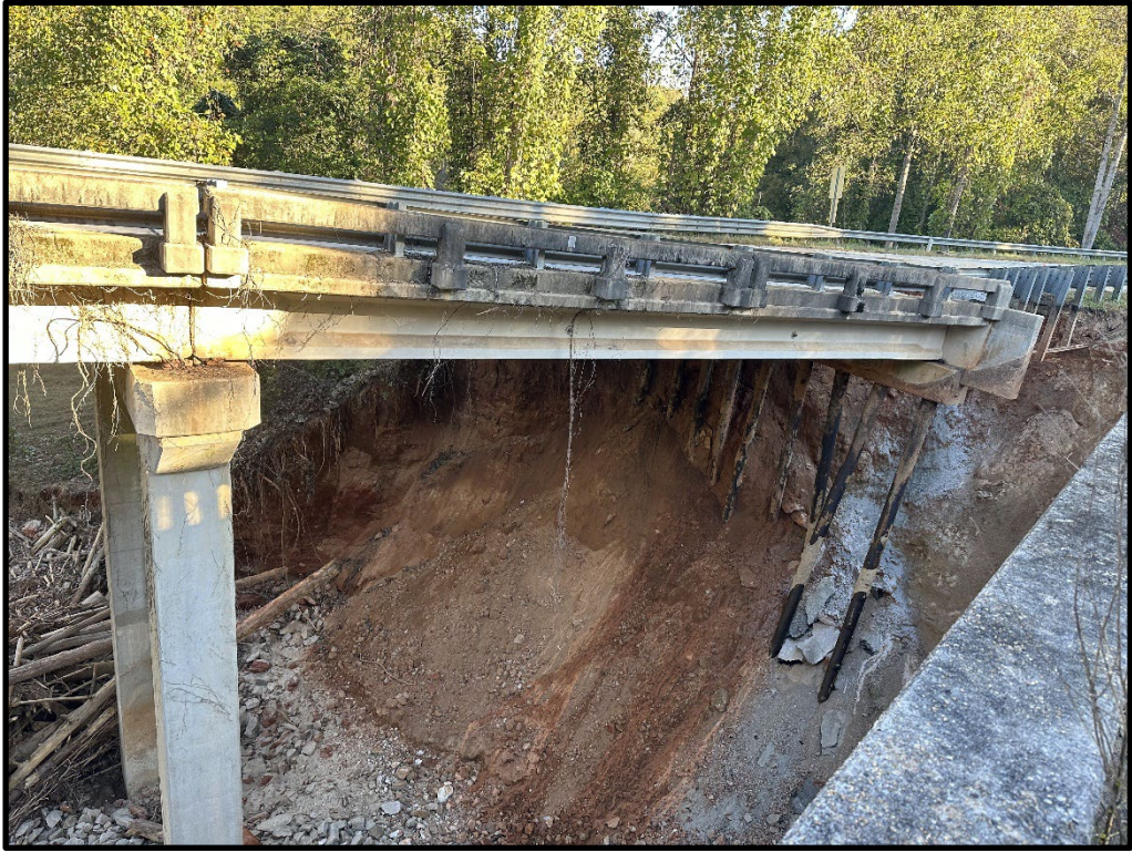
South Side of Bridge – Facing East
