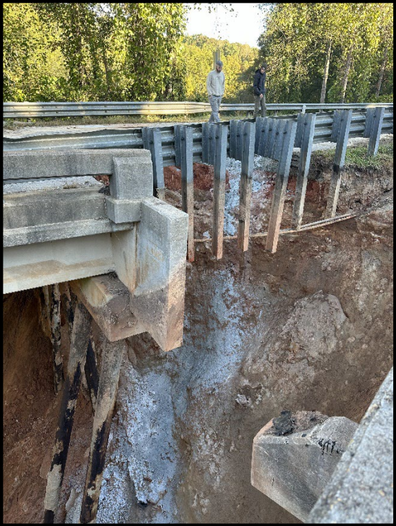
South Side of Bridge – Underneath (Southeastern Corner)
