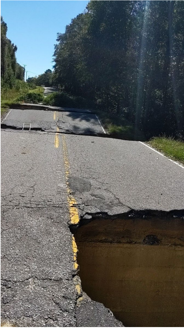
Bridge Deck Looking SW
