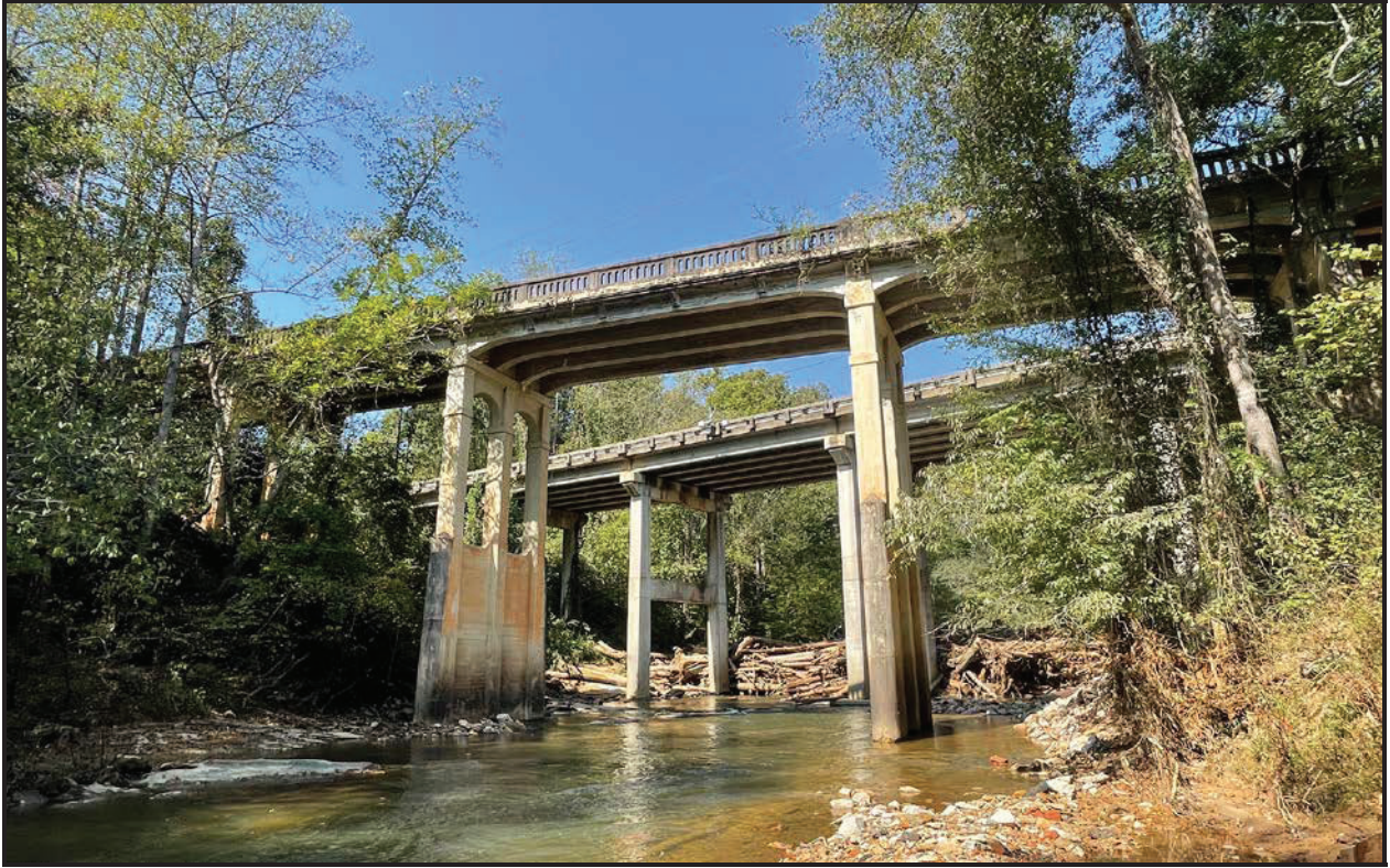
Figure 8. SHPO Site No. 0191, looking northwest
