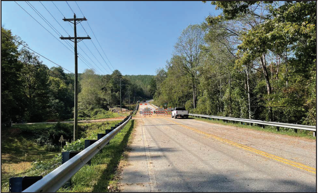
Figure 3. View of Project Area, looking west toward bridge
