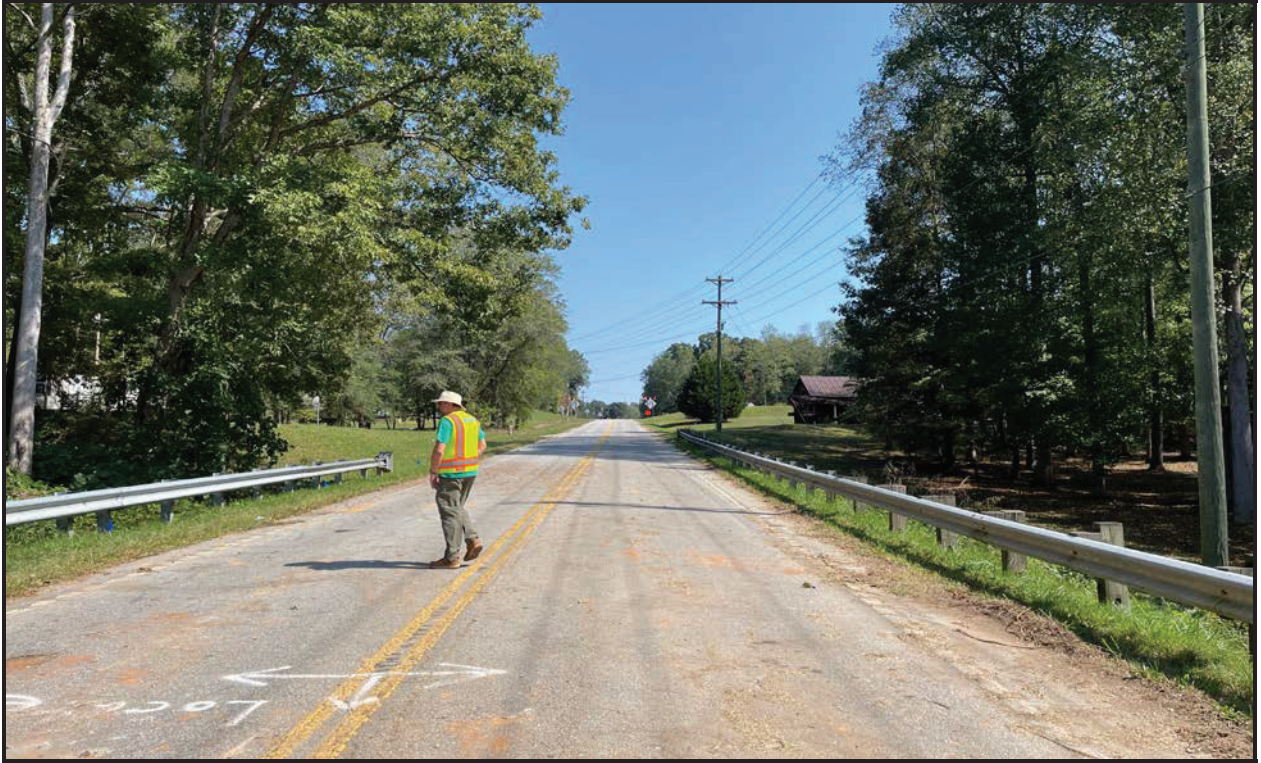
Figure 5. View of Project Area, looking east from bridge
