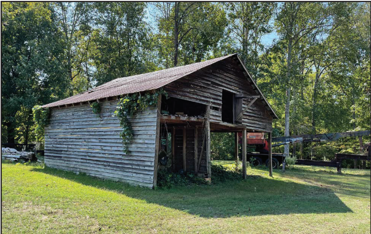
Figure 17. SHPO Site No. 0193, looking southwest
