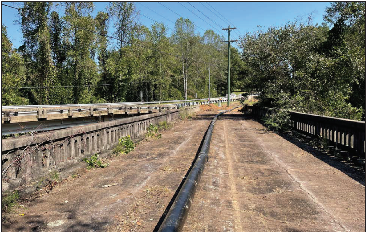
Figure 11. SHPO Site No. 0191, deck, looking east
