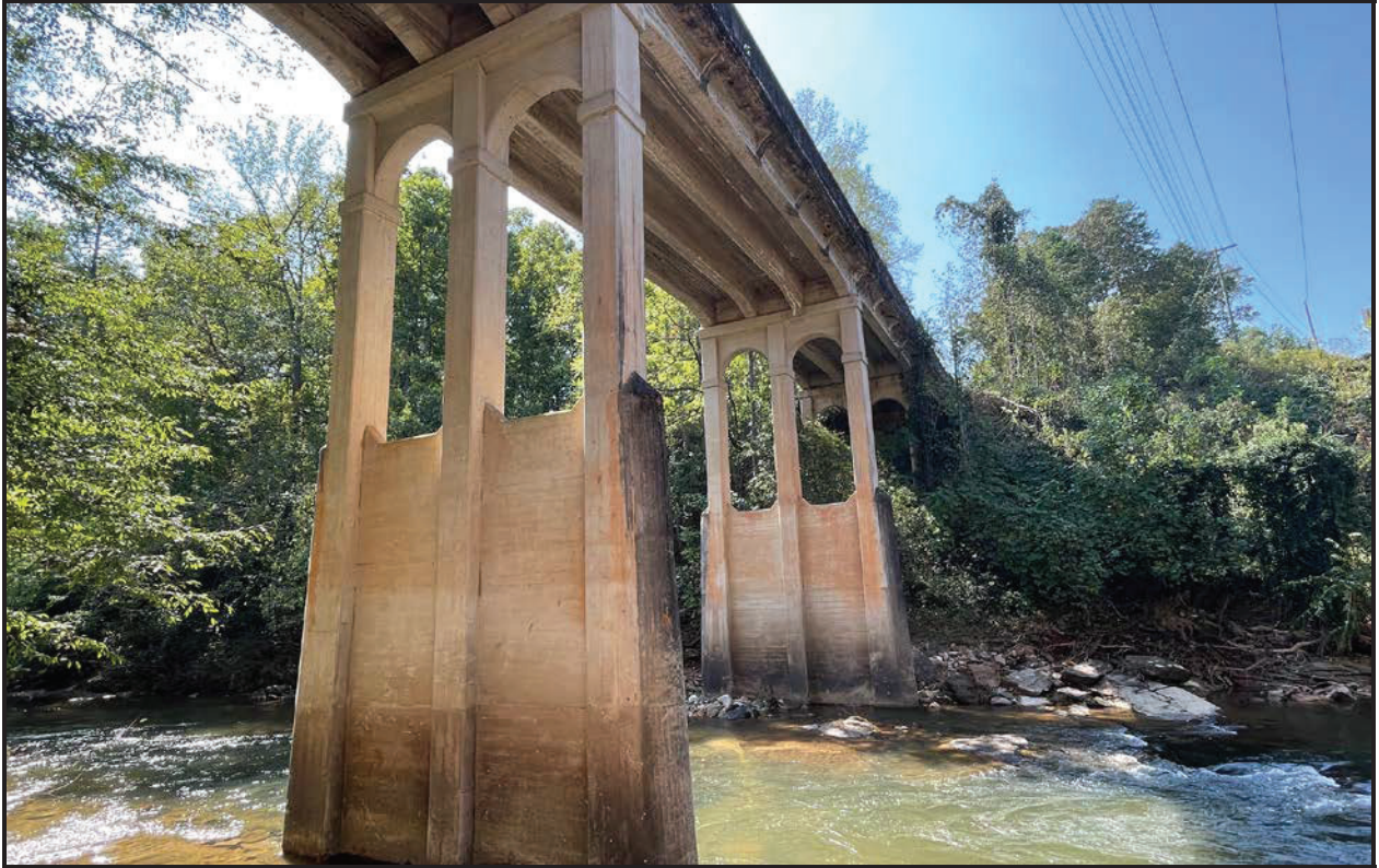
Figure 10. SHPO Site No. 0191, substructure, looking west
