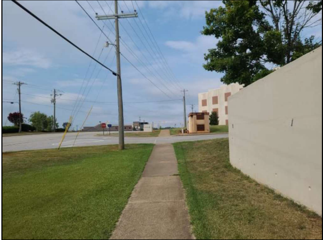
Figure 4: Modifications in the Northwest Quadrant of Project Area, Looking Southwest
