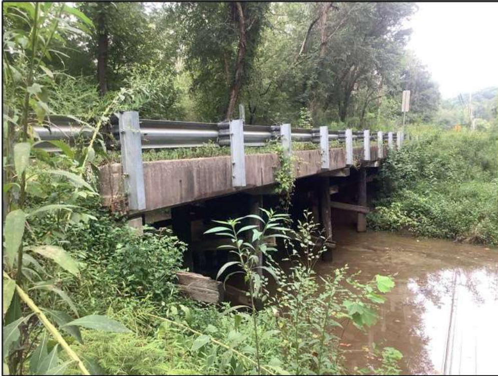
a. Northern Overflow Bridge (Built 1957), Looking Southeast
