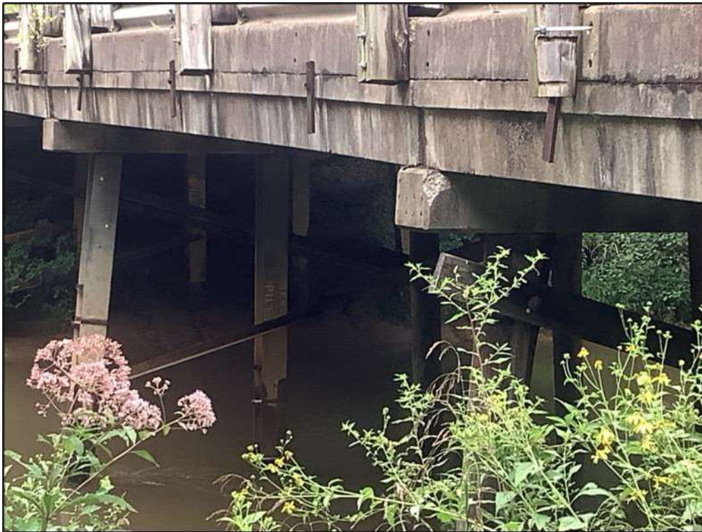
b. Bridge Structure Detail, Looking Northeast
