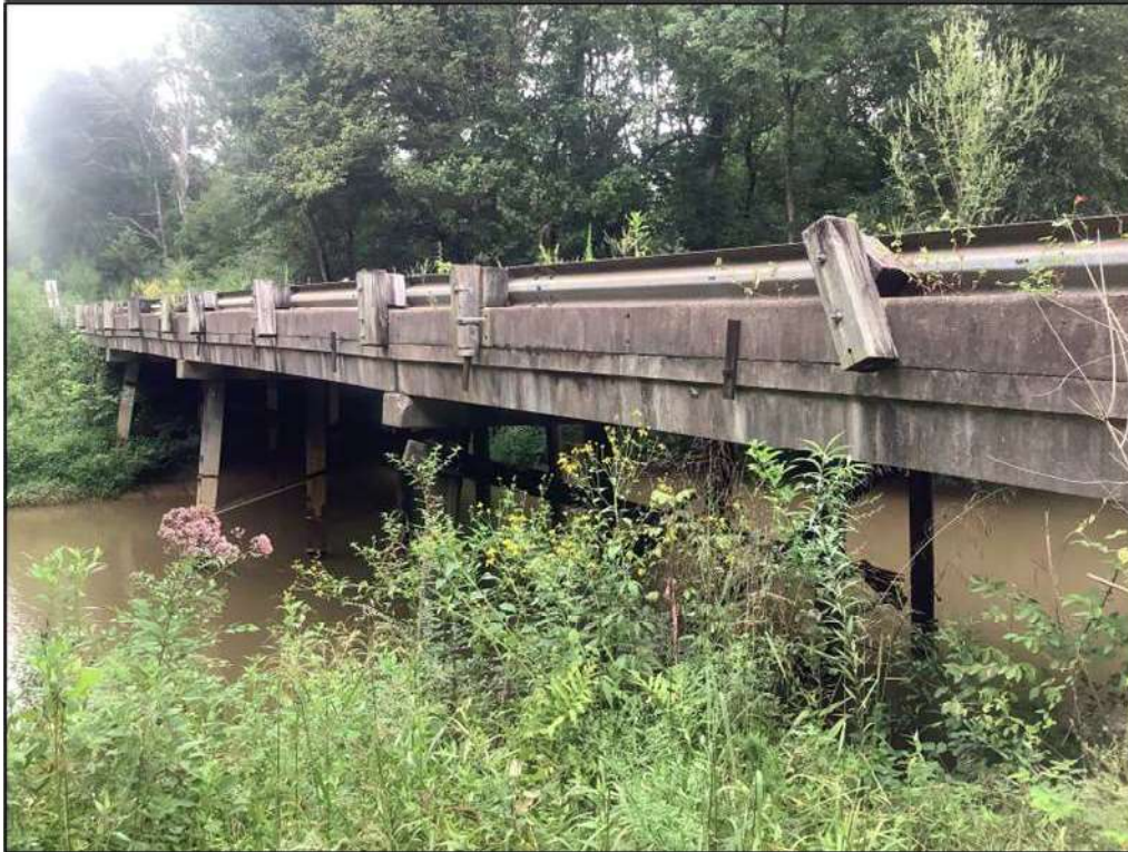
a. Bridge Structure, Looking Northeast
