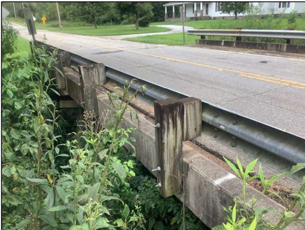
b. Southern Overflow Bridge (Built 1969), Looking Southwest
