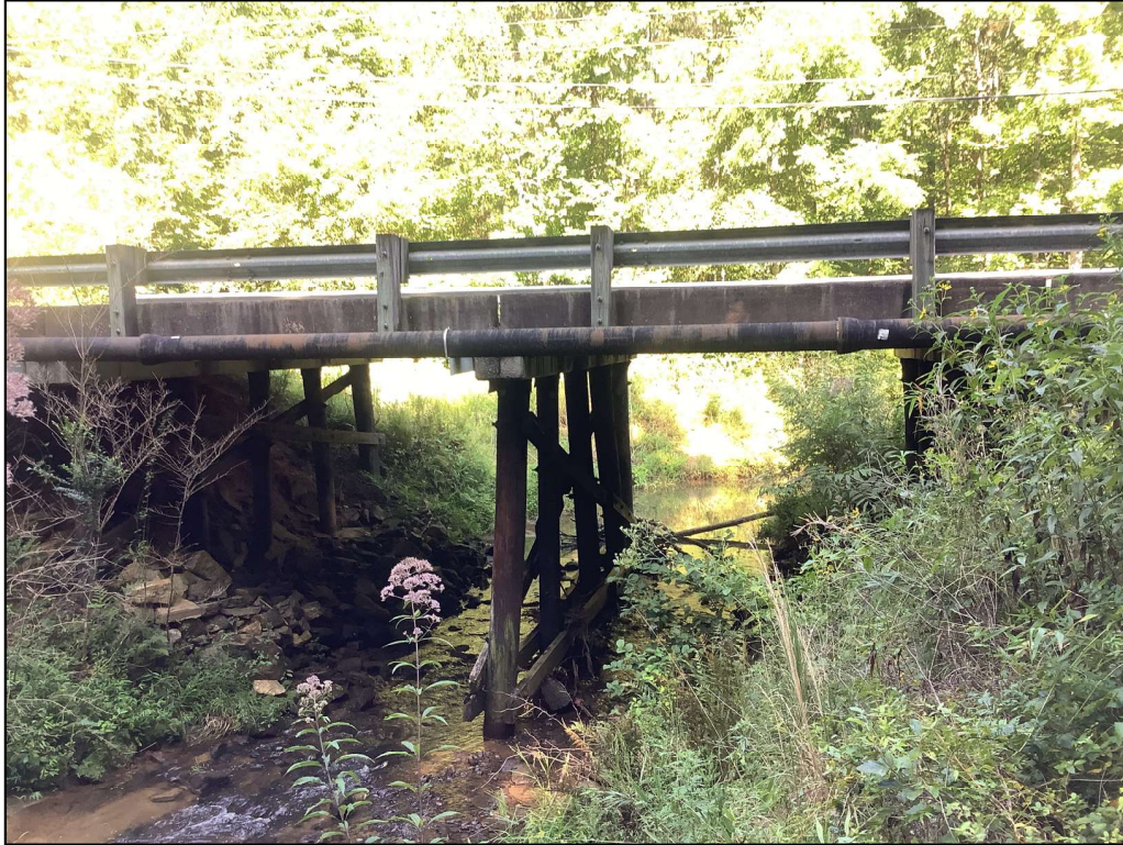
a. Bridge Structure, Looking West
