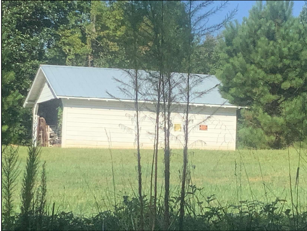
a. Oblique, Looking Northwest
