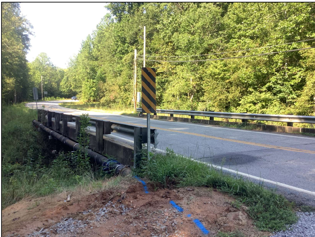
b. Bridge Surface, Looking Southwest
