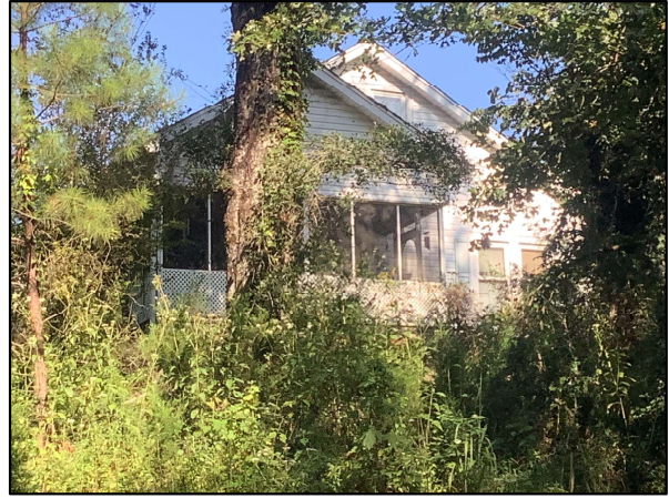
b. East Elevation, Looking West
