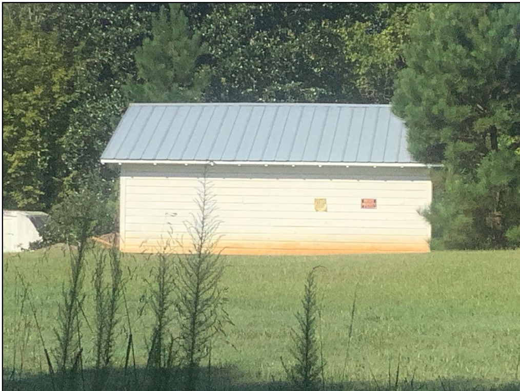
b. East Elevation, Looking West
