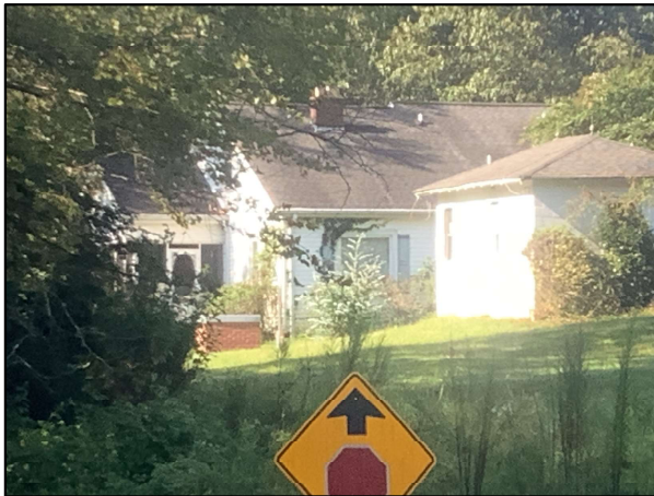
c. Rear Oblique, Looking Southwest
