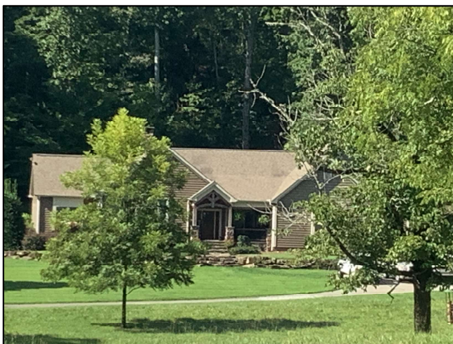
c. Façade, Looking South
