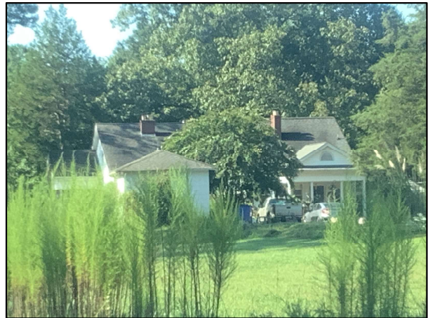
d. North Elevation (Rear), Looking South
